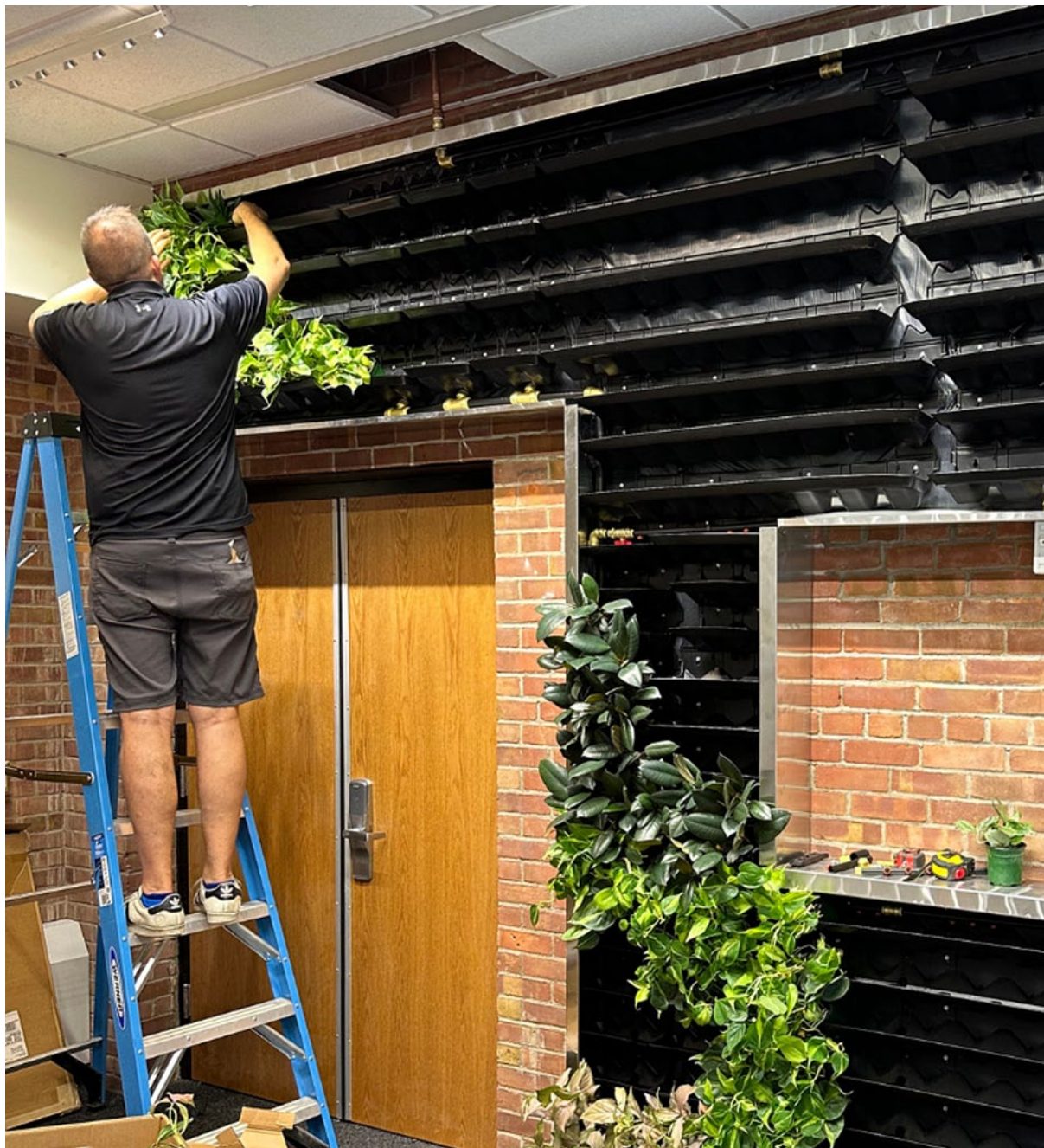
Planting process of the 100 square foot hydroponic Living Wall
