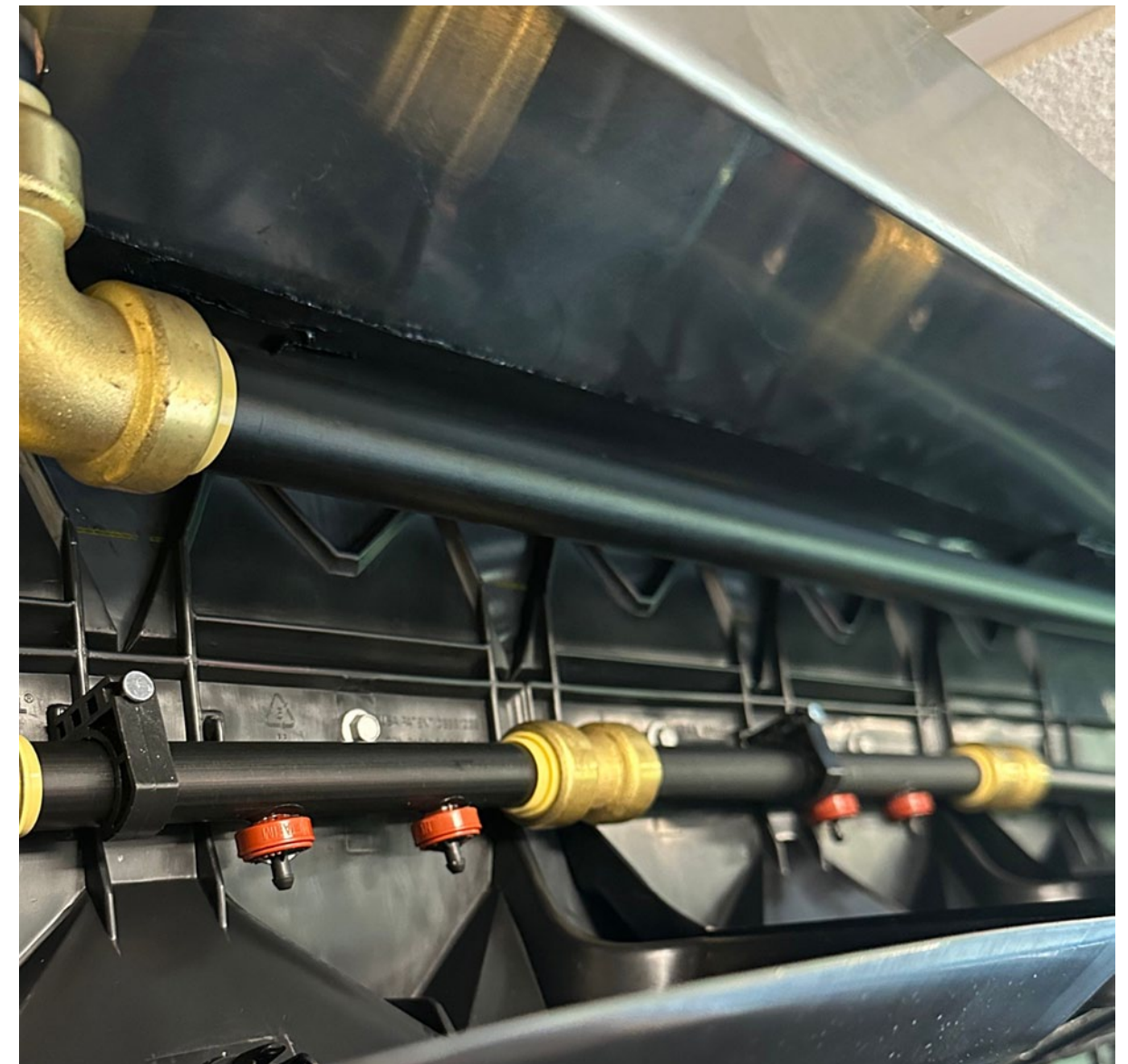
Close-up shot of the irrigation line, highlighting how each individual plant receives its own water
