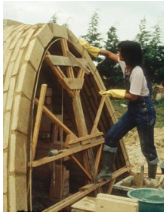
Image: Author working with earth blocks in France, creating a structure based on catenary arch – a form found in nature.
