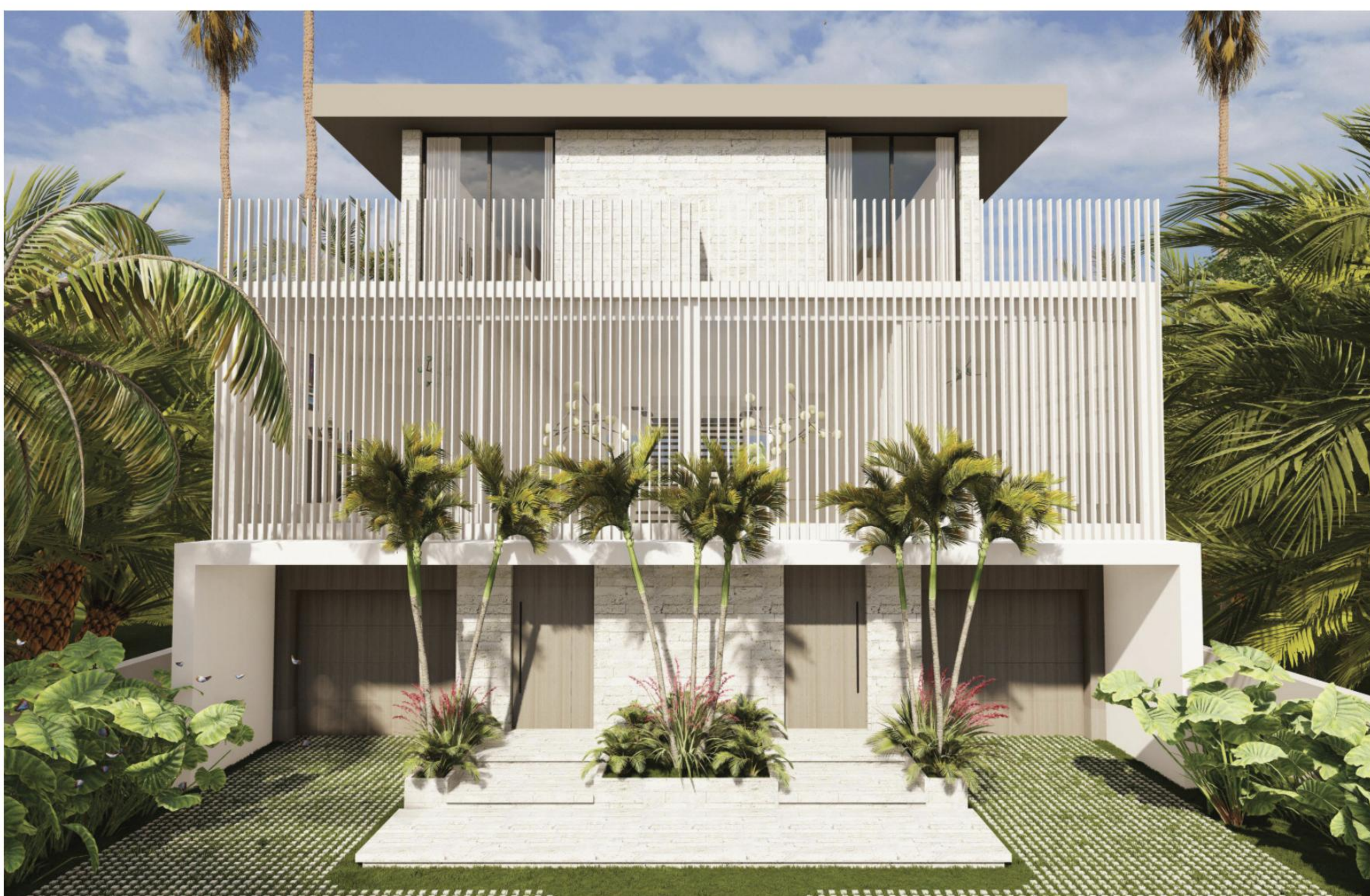
Water permeable paving lines the driveways of Kakun's design for this two townhouse project. The eastern façade has vertical shading devices that extend upwards to become a balcony railing.
