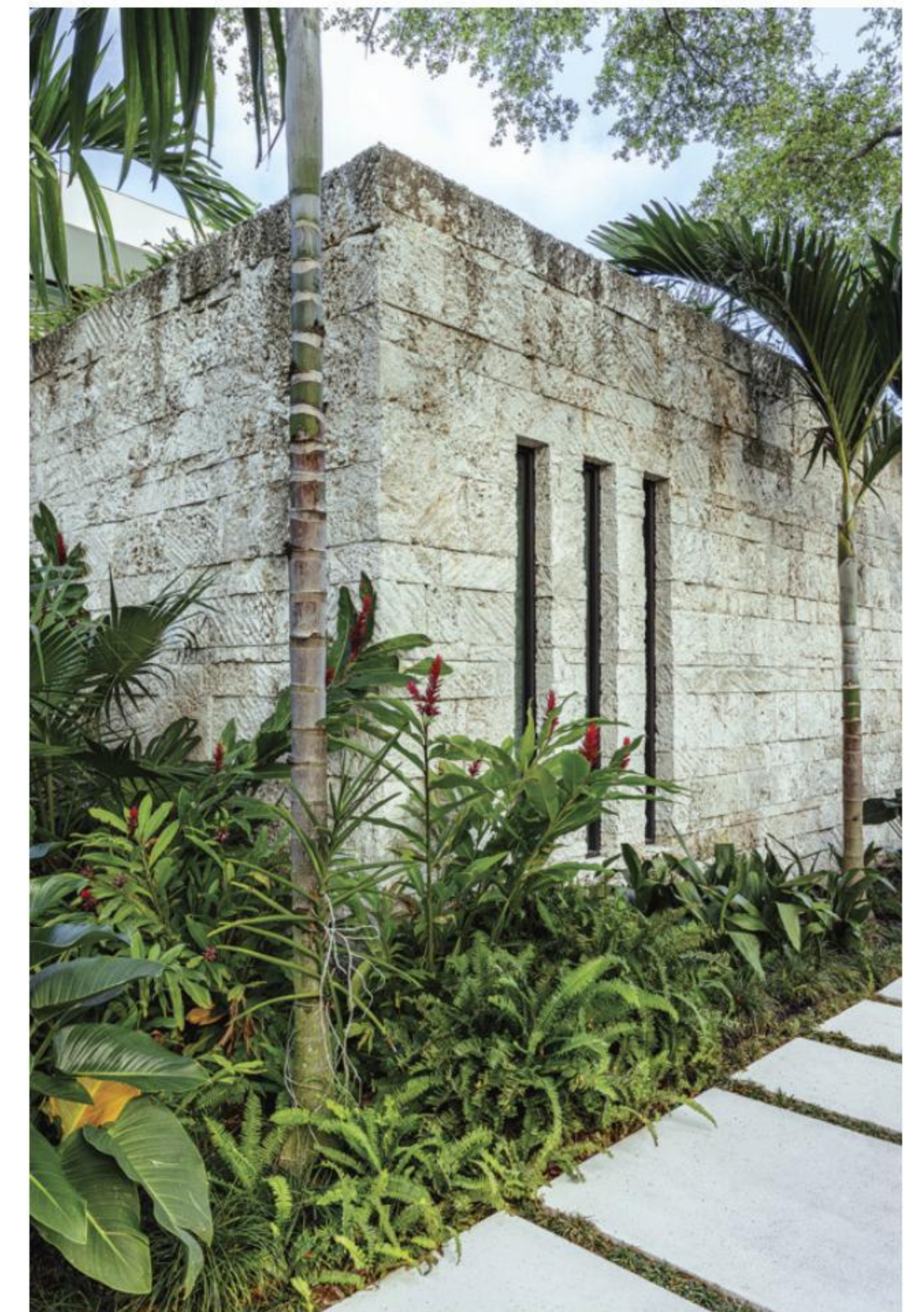
Rough, textured keystone, a stone found in Florida and the Caribbean, was used for detailing inside and out.
