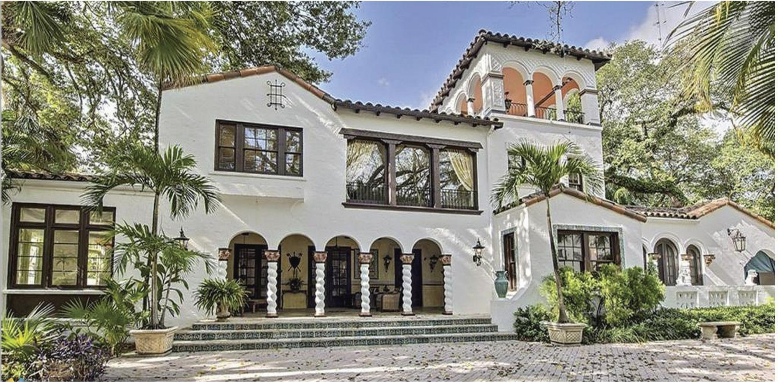
Designed by the architect H. George Fink prior to the Great Depression, the sprawling Sheppard Estate in Colee Hammock is a fine example of Mediterranean Revival, a term the architect is said to have coined. His original studio still exists on Ponce De Leon Avenue in Coral Gables.
