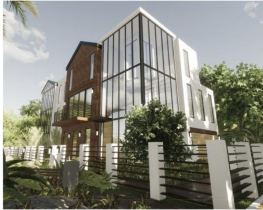
Las Olas | 215 SE 10 Terr | Under Construction The Industrial | 2967 Total SF | 3BR/3.5BA | Den Elevator | Pool | 2-CG | Roof Terrace
