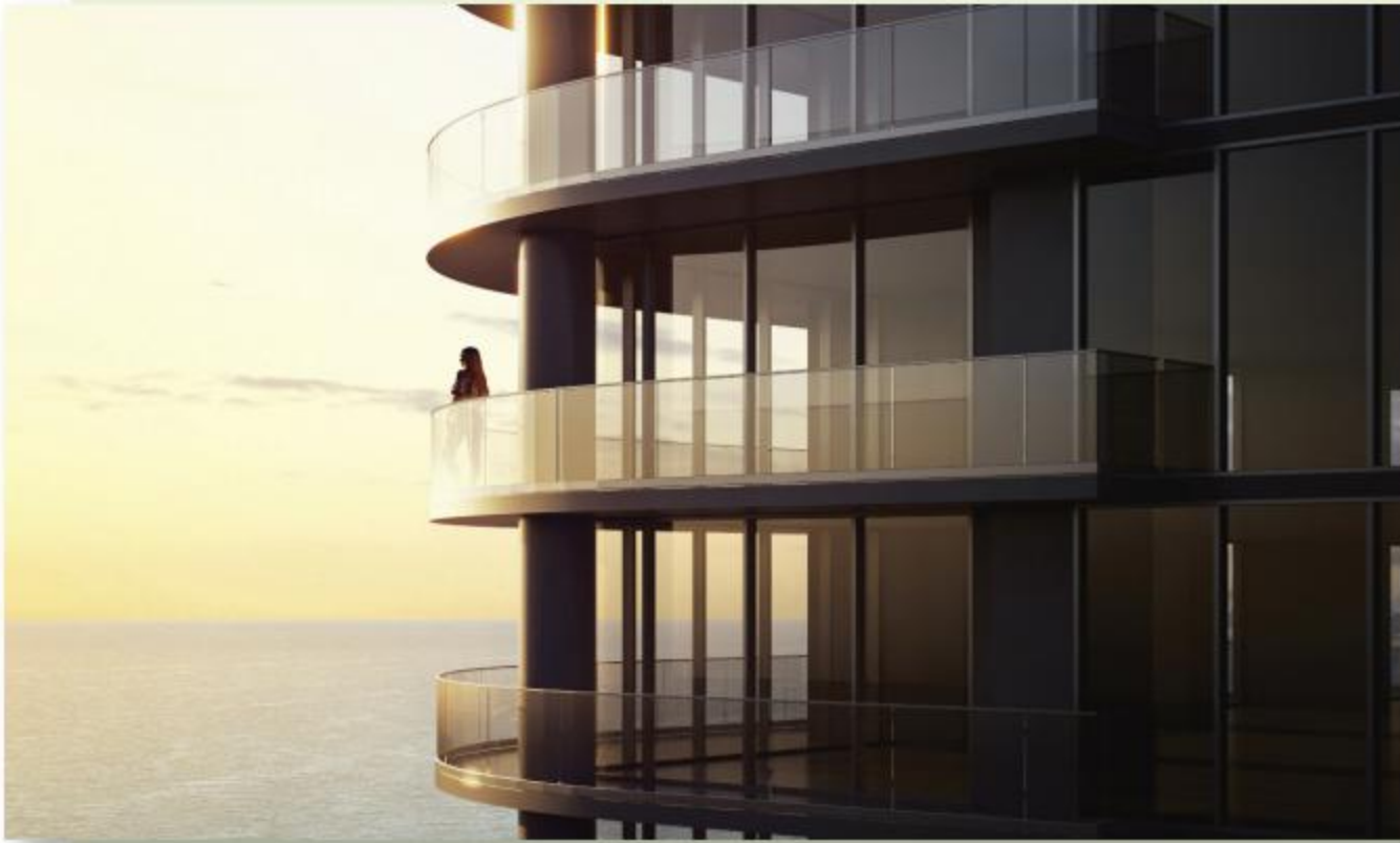
Terrace-like balconies at Selene — this month's cover feature — under construction just off Fort Lauderdale Beach.
