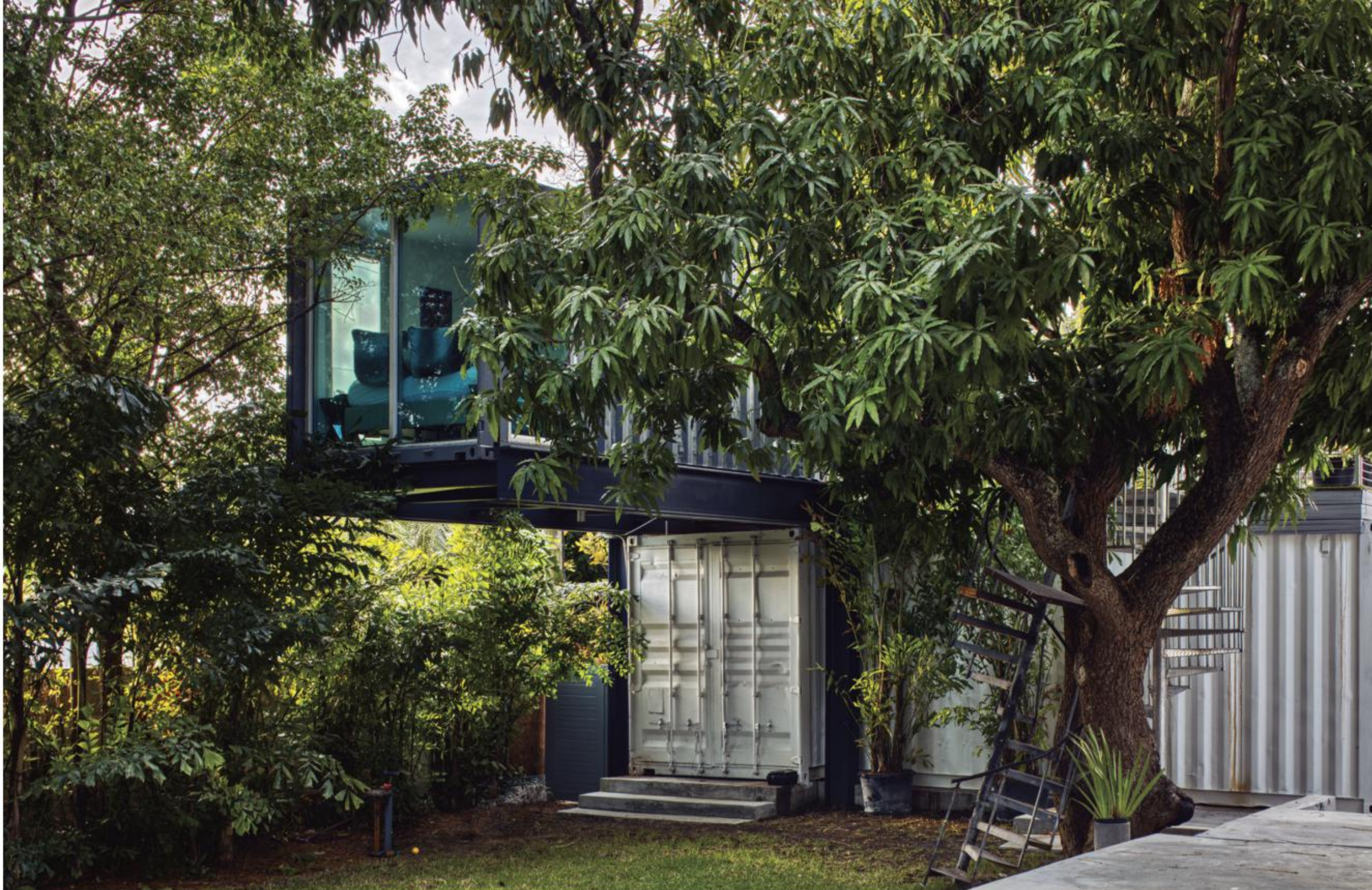
Even though part of the home is created from former shipping containers, its entirety nevertheless connects with the jungle-like nature of its surroundings.
