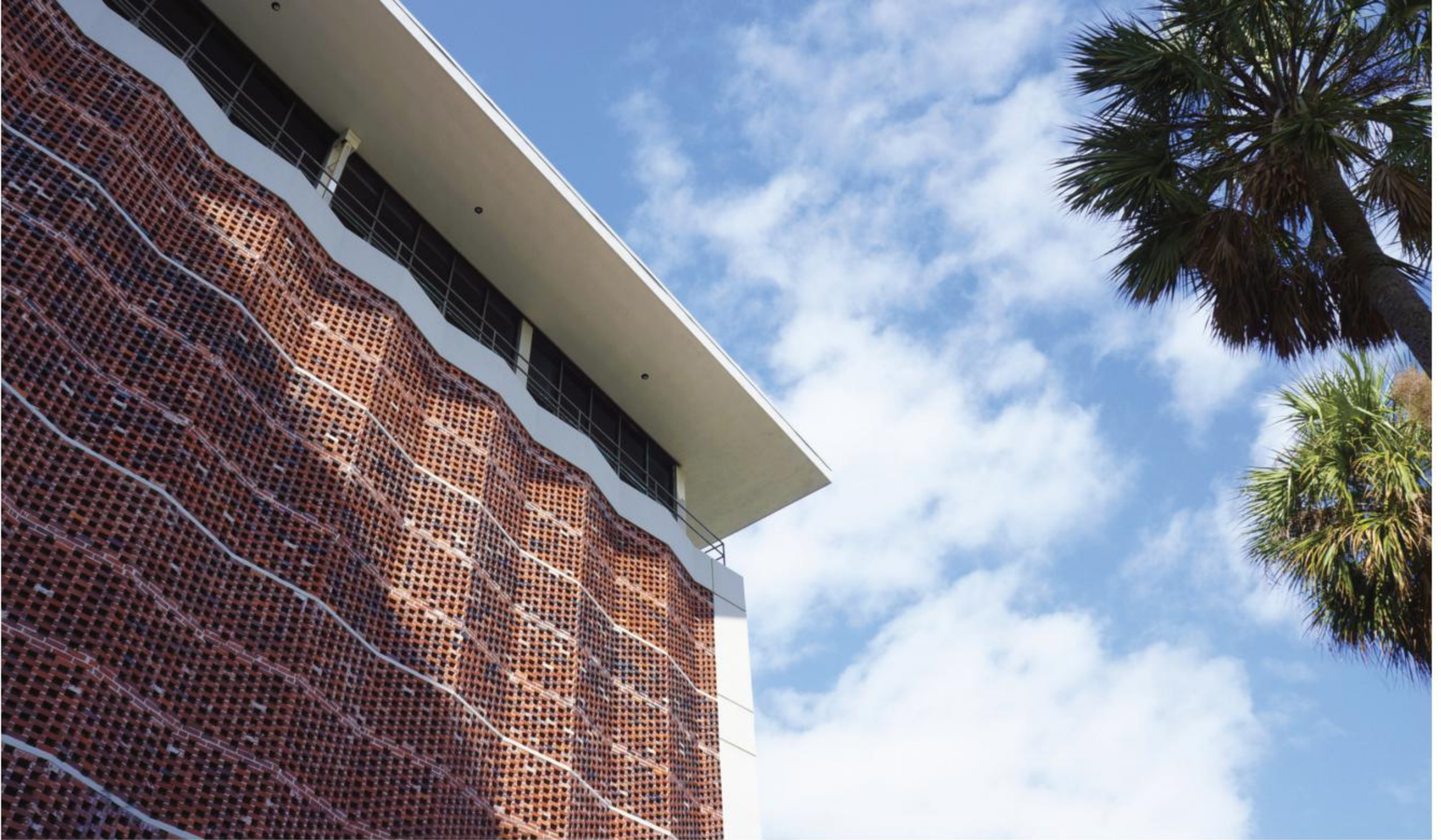
McKirahan's addition of the early 1960s opted for folded-plate, mesh walls of brick, contrasting with the breeze block walls of the original. The top floor and heavy, white stucco edging details are later additions by other firms and could easily be reversed, returning the two building set to its original appearance.
