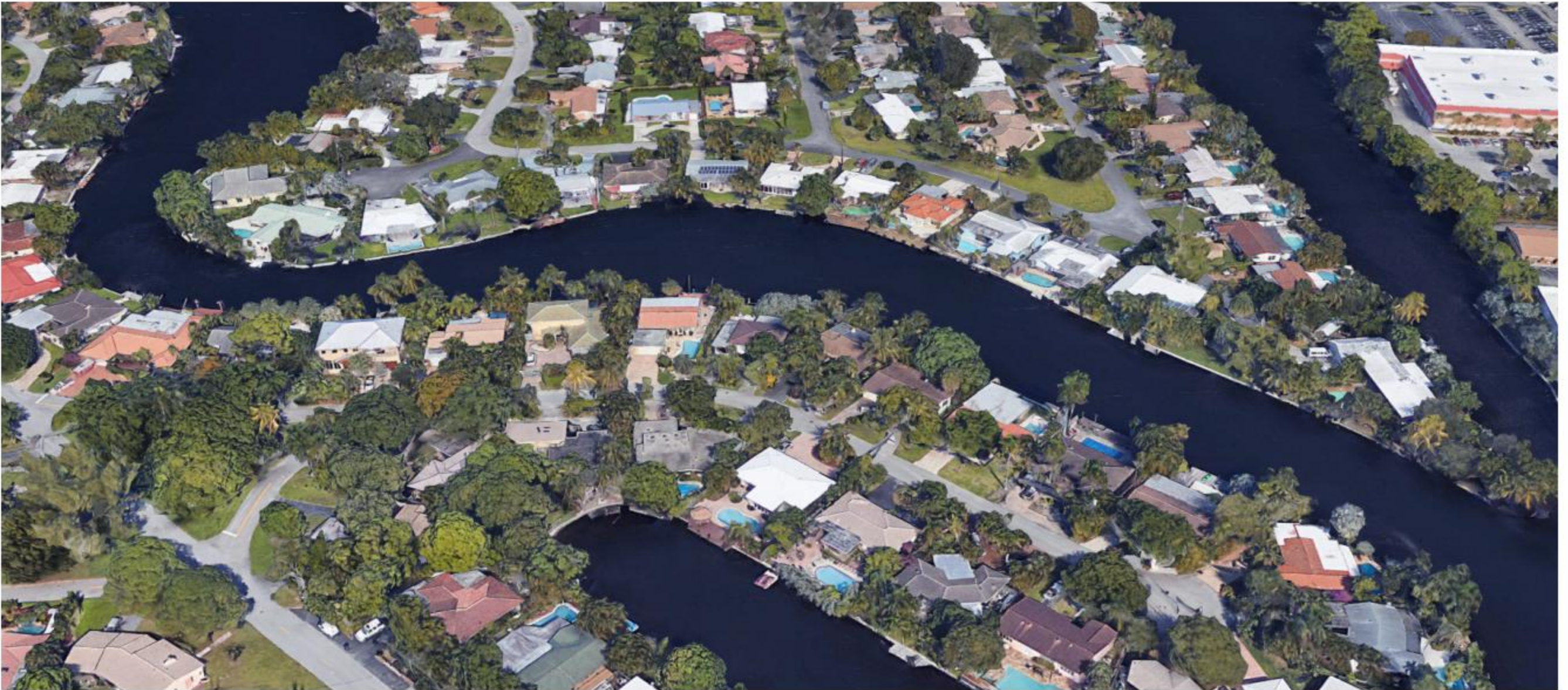
The peninsula of Coral Shores (top of above photograph) is separated by the north fork of the Middle River from Wilton Manors' Coral Gardens neighborhood.
