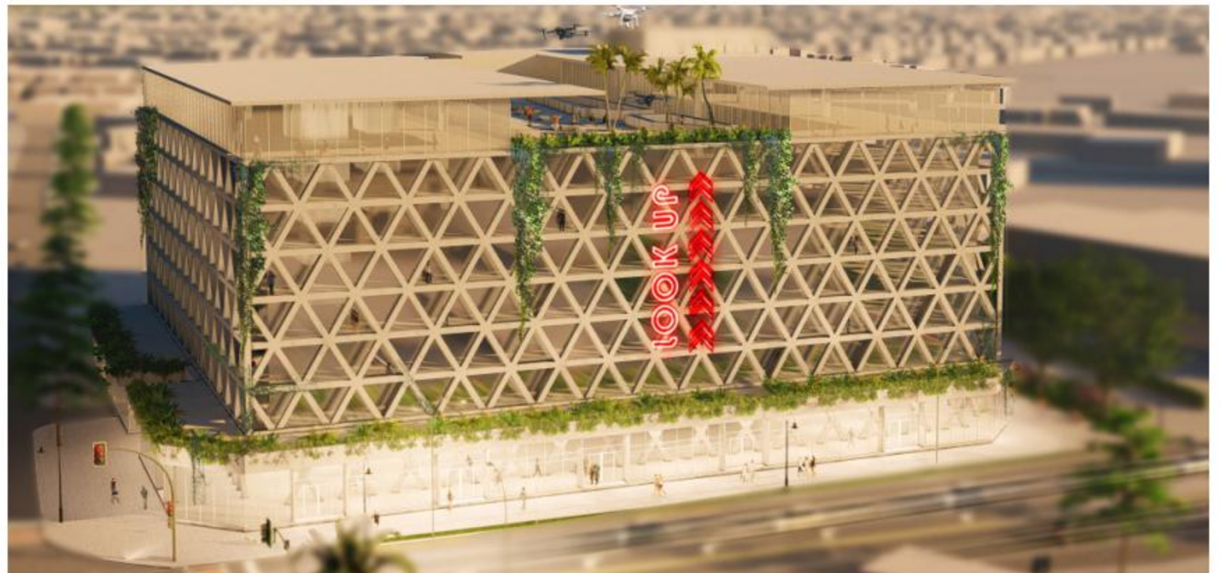
Clockwise, from top: Seen from Wilton Drive, the drone port would rise eight stories and would be landscaped to encourage vines to create a green wall. Above: the Drone Port would incorporate parking garage, ground level commercial space, and community center on top. Left: Diagram showing potential range of drones from the site.
