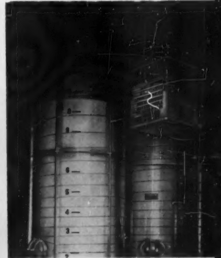
5. Storage tank, Metal-Cladding, Inc.
