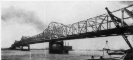
TRI-TEN Steel has cut weight and cost of dozens of major bridges. In the bridge shown here, TRI-TEN Steel saved a quarter of a million dollars.
