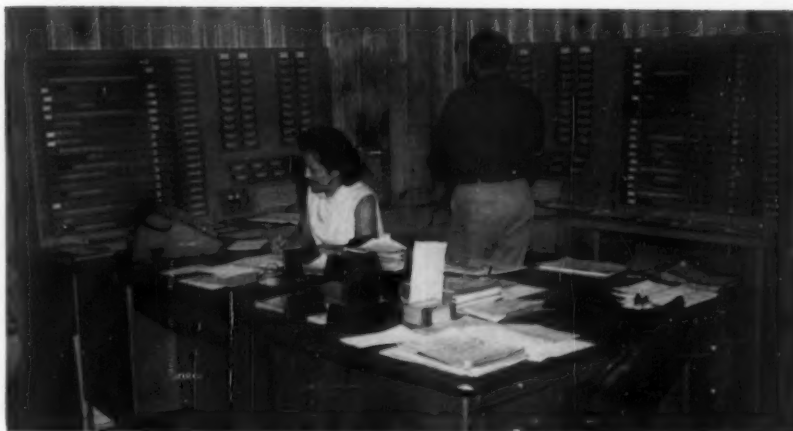
Productograph gathers and summarizes data from 40 assembly line machines
