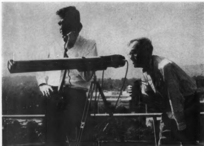
Bell Scientists align optical maser for communication experiments
