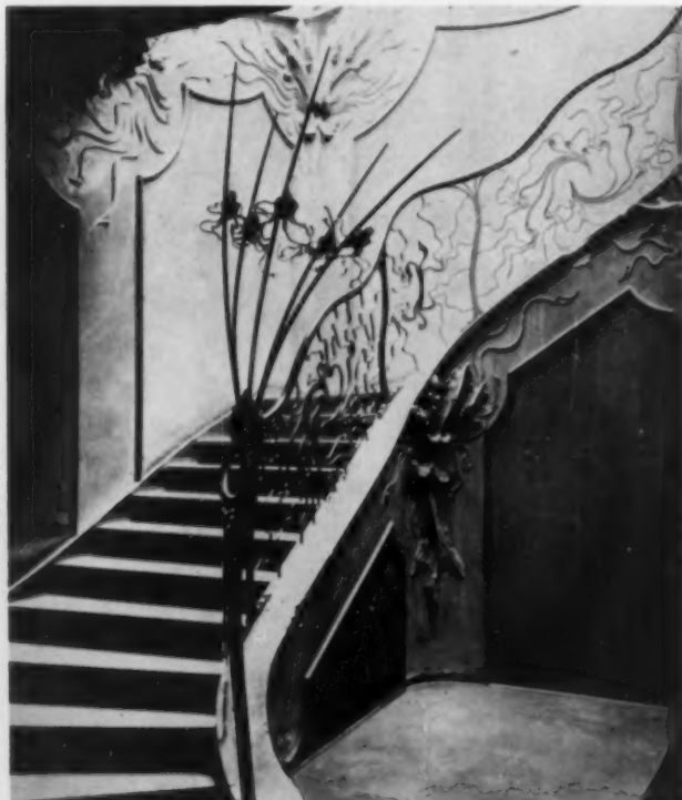
Stair hall, Atelier Elvira, Munich: August Endell
