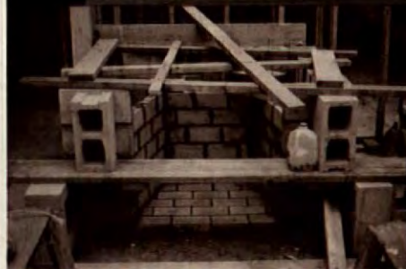
Construction photo (inset, above) shows the fire-brick components of the ground-floor hearth. The fireplace was relocated when the plans were altered.
