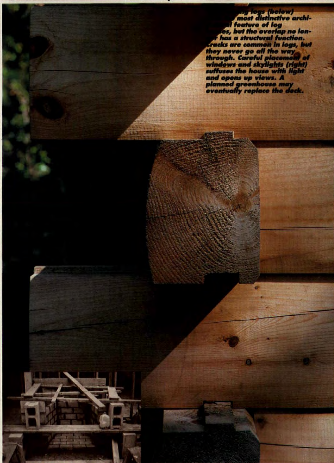
Construction photo (inset, above) shows the fire-brick components of the ground-floor hearth. The fireplace was relocated when the plans were altered.
