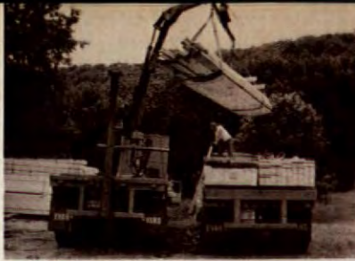
Logs are pre-cut and numbered to simplify on-site construction. Delivery of a kit (left) should be timed so that construction (right) can begin immediately.
