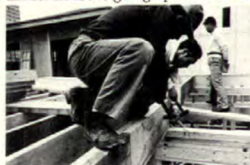
Hammer-nail method is replacing Japan's system of mortised joints.
