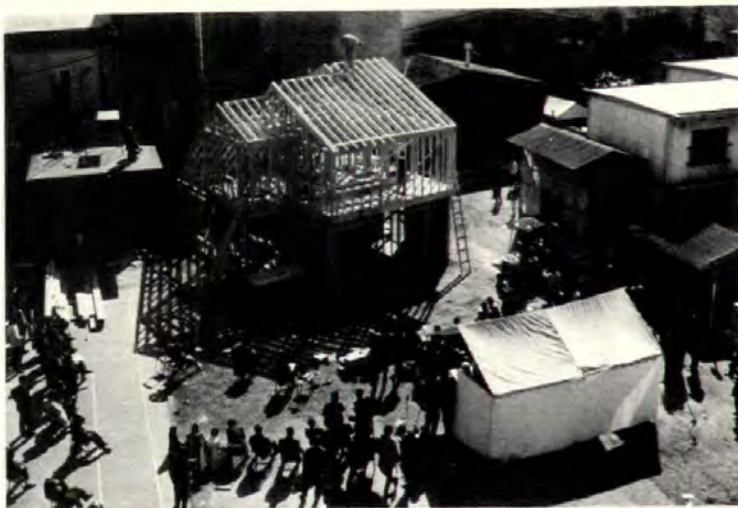
American-style framing is demonstrated by U.S. carpenters building model house on laboratory grounds of Japan's Ministry of Construction.
