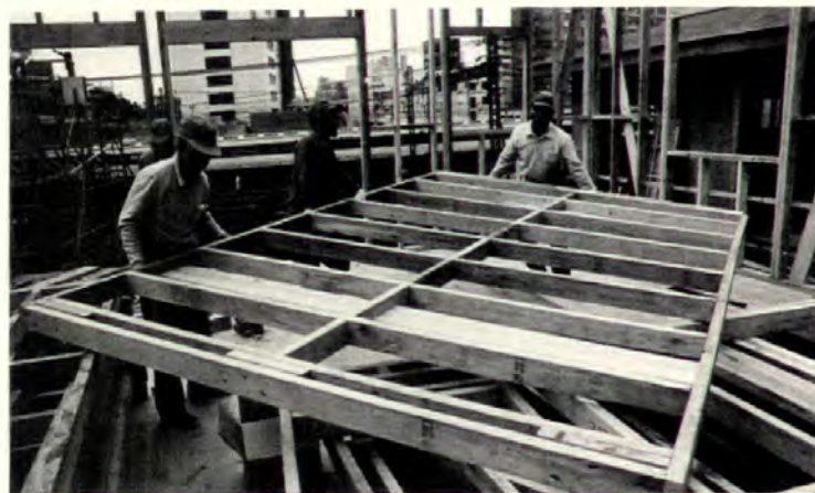
Tilt-up panel is assembled in American manner by Japanese carpenters. This model house is going up in downtown area so crowds can take a look.
