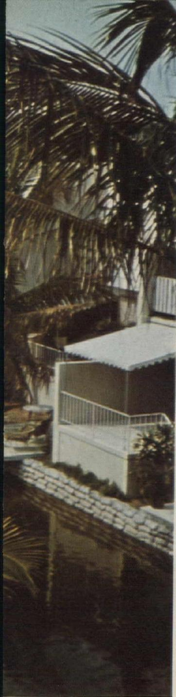
**Narrow waterway** (above right) gives the effect of a long canal, brings a feeling of unlimited space to the project. Rip-rap at edge of water is made of bagged concrete dropped in place and spiked down with reinforcing bars. Entrance and parking courts (right) are sited between each two rows of houses.
