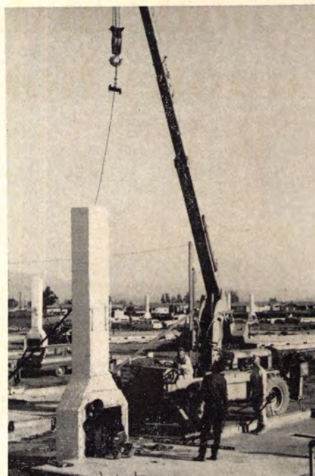
TEMPORARY SUPPORT , seen at rear of chimney in foreground, serves until framing is up.
