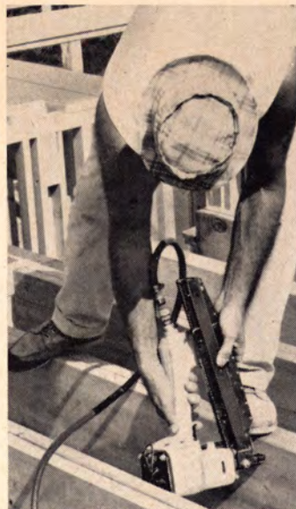
Pneumatic nailer drives full round-headed nails from 6d to 10d. Air-pressure requirement for hardest wood is 80 psi, and can be reduced for softer wood. Nail is driven with single impact, by trigger or touch-trip. Duo-Fast, Franklin Park, Ill.
