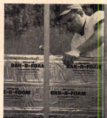
Foam-backed aluminum permits lap siding to be nailed directly to studs—no sheathing. Alsco, Akron, Ohio. Circle 259 on Reader Service card
