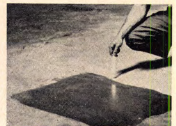
Epoxy patching compound for concrete is mixed with sand to produce a trowel-on mortar. Result: a patch stronger than heavy-duty concrete. Contractors Chemical, San Leandro, Calif. Circle 230 on Reader Service card
