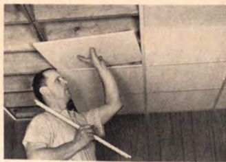
Grid ceiling system for installations where headroom is at a premium fastens flush to joists, using only 1/4" of overhead space. However, ceiling clips permit grid to be lowered as much as 2 1/4" to clear pipes. Insulite, Minneapolis.
