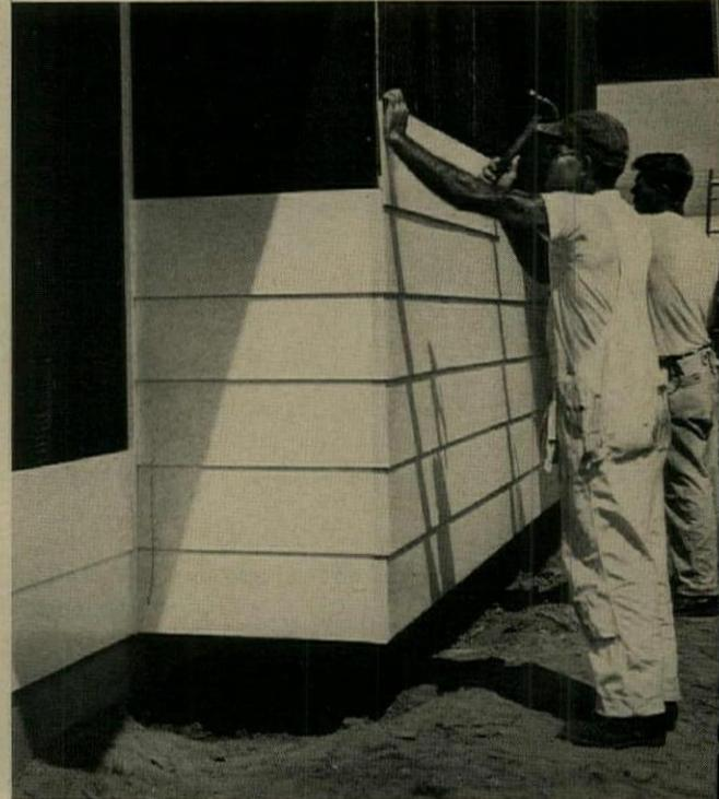
**TEDLAR\* PVF film** is a tough new film-finish—not a liquid or a spray. TEDLAR is factory-bonded with special Du Pont adhesives to wood or metal, actually becoming part of the material it protects.
