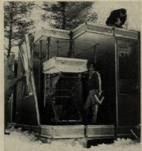
LIFT raises roof panels into position. Fascia panels finish roof and floor.
