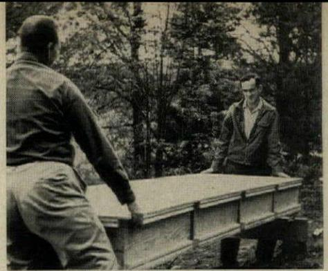
FLOOR PANELS are assembled into 12' lengths before they are placed on the foundation.
