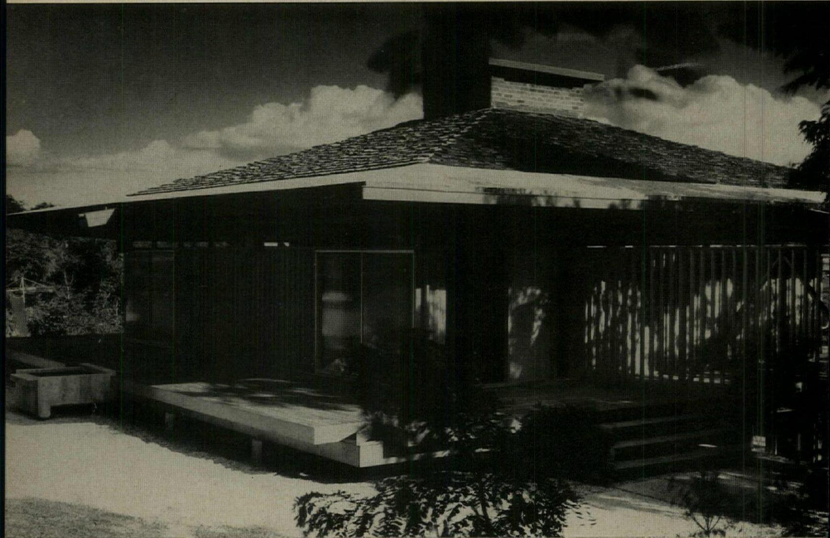
Broad deck and huge roof extend out 9'. Hillside site gives the illusion that the house is one-story, though the lower level opens to grade on three sides. Walls are rough-sawn board-and-batten; roof is cedar shakes.
