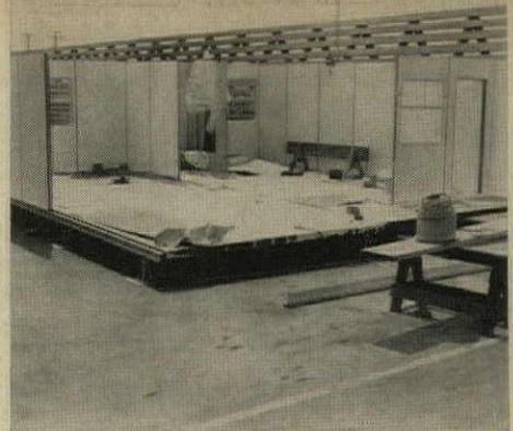
**ERECTION** starts with placing foundation jacks, floor channels, and panels. Then walls go up.
