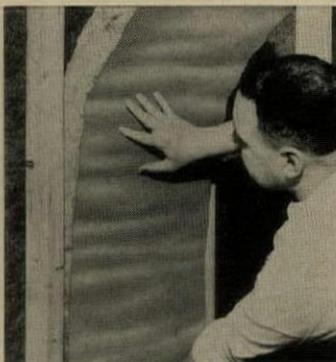
**Mineral-wool insulation** is made slightly oversize for fast fitting between studs. When blanket is pressed in place, the spring-back of the mineral fiber holds it without stapling. Sizes: 15" wide, 4' and 8' long, 2", 3", and  $3\frac{5}{8}$ " thick. Celotex, Chicago.
