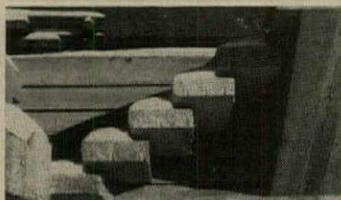
Granite steps cantilevered from the concrete terrace wall are another design surprise.
