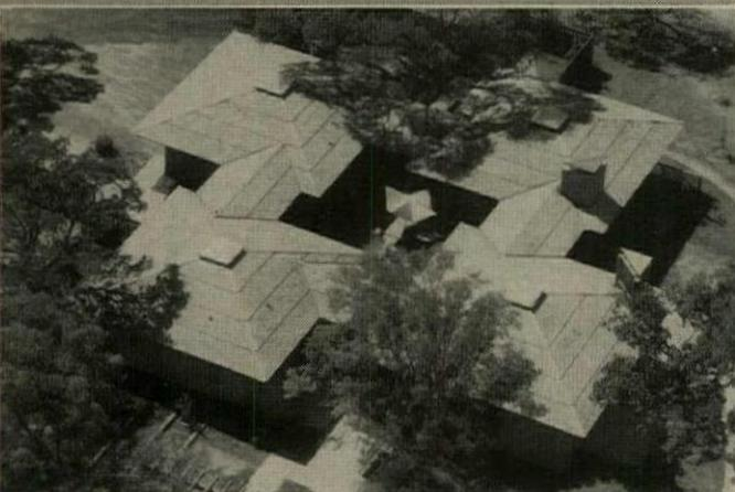
Aerial view and plan show how the galleries tie different zones together, and how the deep (4'6") roof overhangs shelter the center court.
