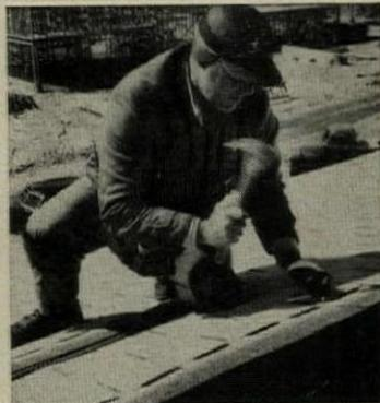
**A SHEATHING-SIDING COMBINATION THAT INSULATES AND GOES UP FAST!** Save \$40 to \$80 a house with Barrett nail-base Rigidwall sheathing, a product so dense you can apply shingles directly to it, so strong it needs no corner bracing. Maintenance-free Barrett asbestos-cement siding comes in the widest range of colors, colors sealed in plastic to prevent fading. Available in more locations than from any other manufacturer.
