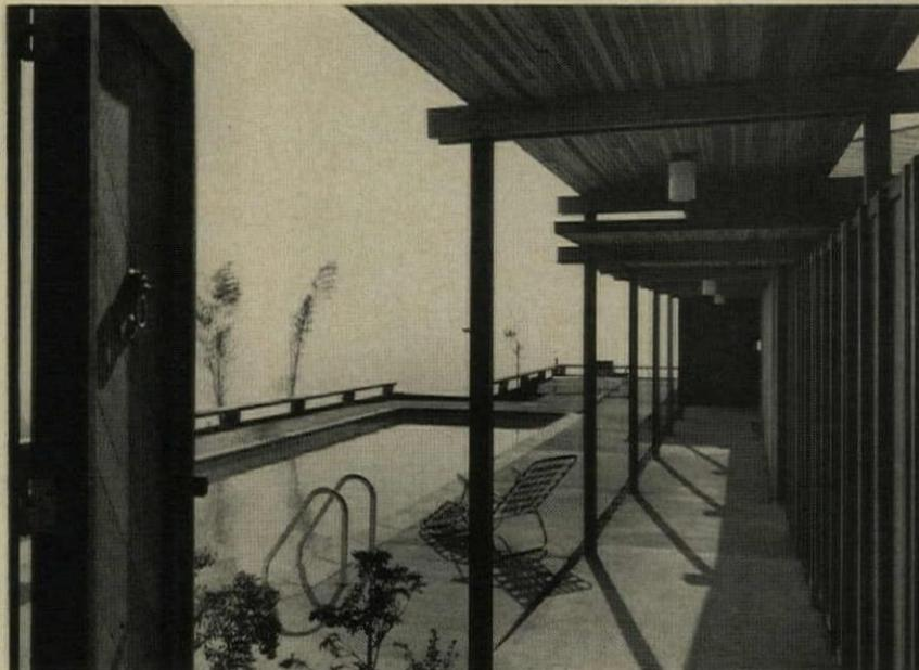
Covered entryway has the only flat roof plane, extends 60' from carport to front door. Pool is set in broad terrace behind retaining wall.
