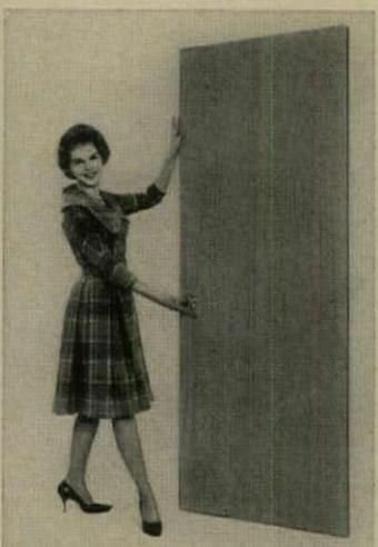
**Prefinished interior door** with Laminex surface is factory-sized, beveled and machined for hinges; and lockset to specification. Mohawk-Laminex doors are polyethylene-wrapped; wrapper stays on during installation. Plywall Products, Corona, Calif.
