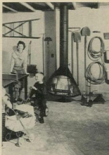
**Garage wall liner** adds storage to garages, storerooms, workshops, etc. Perforated hardboard is 4'x8'x1/4" with 9/32" holes. Sheets are prefinished in neutral driftwood and can be installed directly on studs.
