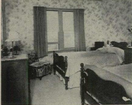
**SLIDING GLASS DOORS** opened this old-fashioned bedroom to the pleasant garden beyond, made the room seem bigger, and brought in quantities of daylight. Where big windows already exist, sliding glass doors can usually be inserted in the opening with minimum reframing, for the header is already in place, and only the windows and wall below must be removed. Designer: William Kipka, AIA. Builder: Ted Kirkendall. Location: Los Angeles.
