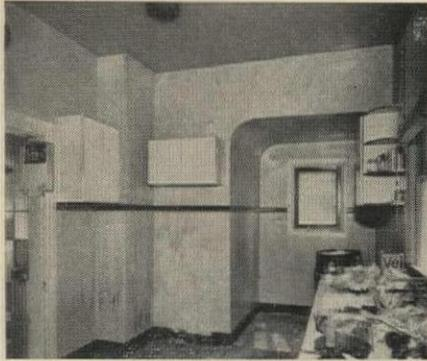
**INTRICATE PLANNING** was required to make a well organized kitchen of the jig-saw floor space in the old kitchen (above). Changes include walled-off laundry area in alcove, dropped ceiling over new cabinets and range. Builder: Wolf Supply Co, York, Pa.
