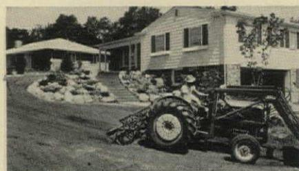
**TILLER RAKE** mixes topsoil and subsoil.
