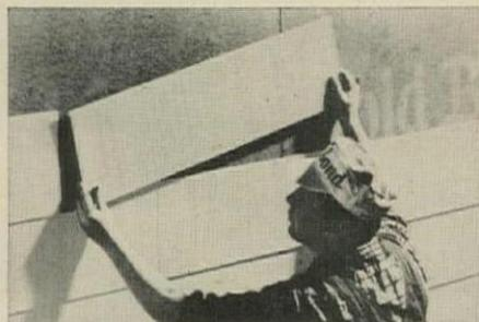
**Clapboard-style siding** is Gold Bond's latest asbestos-cement board. New 9"x32" size gives 8" exposure. Texture matches other Classic Shake Siding. Acrylic coated finish preserves color, is permanized for dimensional stability.
