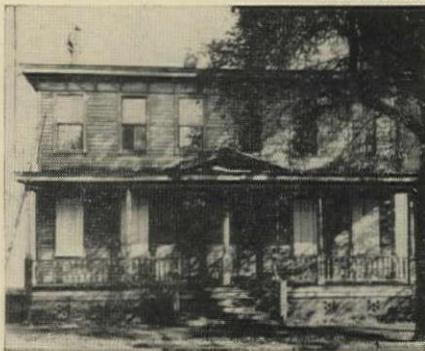
**FOUR DESIGN CHANGES**—removing the porch and false gable, adding new trim to emphasize the doors, running the siding down over a too-high foundation, and building a broad stoop to tie the doors to grade—simplified and greatly improved this exterior. This is an apartment building in Savannah. Builder: South Atlantic Gas Co.
