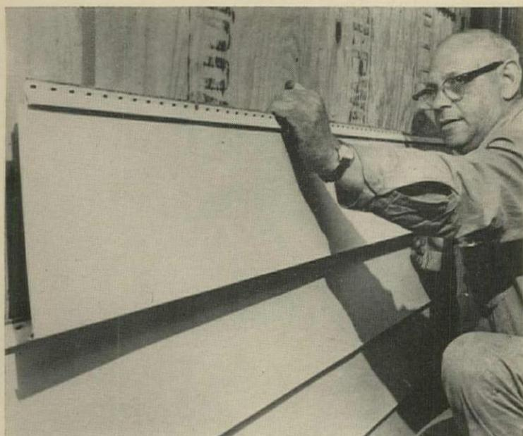
**Aluminum siding** is now being made by Johns-Manville. The 8" clapboard is sold with and without 3/8" backer board. Insulated boards are 10'8", uninsulated 12'6". Line also includes 12" vertical siding and all necessary accessories.
