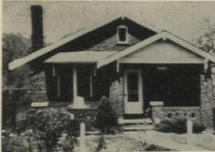
**NEW FACE AND NEW WING** combine to make this standard 1920 house into a trim-lined—though still modest—house. Heavy porch and superfluous roof lines were removed, a new wing added, and new siding installed. Builder: George Lewitt. St. Louis.
