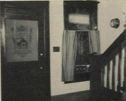
**NEW STAIRS** with wide treads, low risers, and no balustrade add spaciousness to this entrance hall. By adding a turn to the stairs, it was possible to change the stair pitch without altering the framing around the opening in the second floor. New single-pane window brightens the whole room, and flush door and closed up front window increase privacy. Architect: Fred Rogers. Builder: Maury Johnson. Bellevue, Wash.
