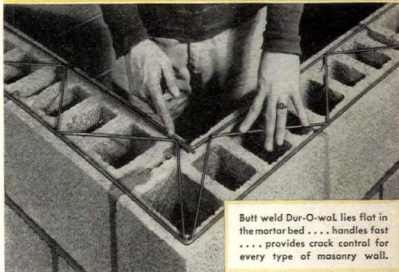
Butt weld Dur-O-wal lies flat in the mortar bed . . . handles fast . . . provides crack control for every type of masonry wall.
