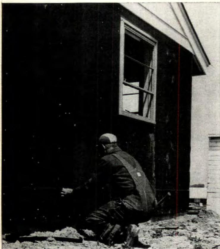
**1.** Workman checks level before installing first course. Duraply is exterior grade Weldwood Plywood with a permanent "CreZon" overlay bonded to its surface. "CreZon" (phenolic resins and cellulose fibers) is tough, weatherproof, supersmooth.
