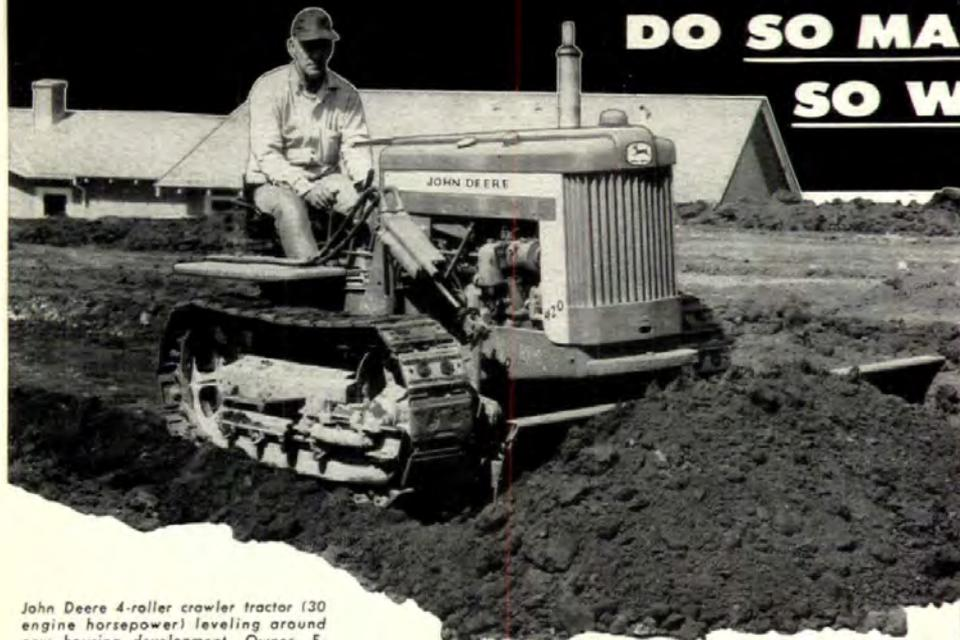
John Deere 4-roller crawler tractor (30 engine horsepower) leveling around new housing development. Owner: F. D. Sperry Co., Burlingame, California.
