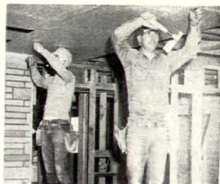
**6 Drywall nailers** wear helmets to hold wallboard against the ceiling joists while they are nailing it in place. When ceiling has been installed they move to the partitions, which are also covered with wallboard. Hammers used in nailing are rounded on striking face to dimple the board slightly around nail-head.
