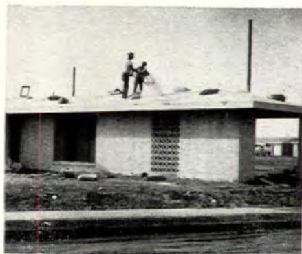
**4 & 5 Roofers** lay built-up roofs with gravel topping as shown in photo. Other crews lay asphalt or wood shingles. All materials are piled on sheathing in exact quantities for use. (Fifth step, not shown, includes plumbing, wiring, and duct-work. These jobs, which require special permits, are subcontracted.)
