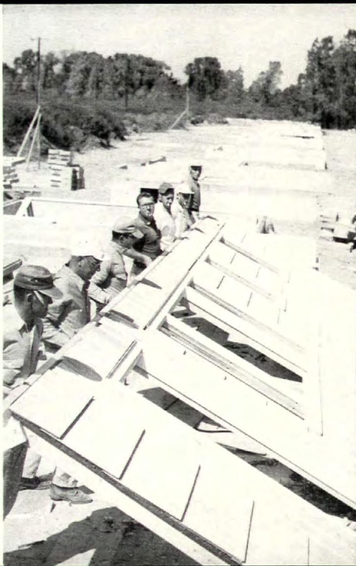
**First Step** in Dietrich's speedy system is completion of finished shingled sidewall sections lying flat. With strong, rigid Bildrite Sheathing applied to frame, carpenters can safely kneel, walk and work anywhere on surface. Insulite Shingle-Backer and cedar shakes are quickly applied, and wall section is ready to go into place.
