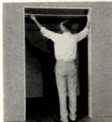
Kenna-pak steel header takes minimum headroom. Eliminates fascia and cutting of doors—standardizes all door opening heights.
