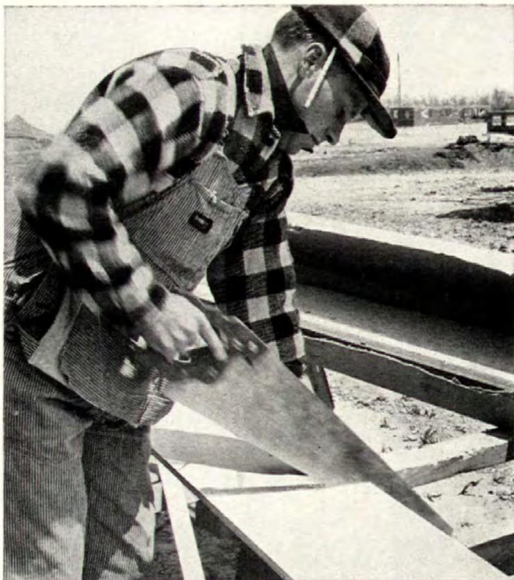
**2.** Duraply is easy to work... can be sawed with any hand or power saw used to cut plywood. Special tough overlay holds wood fibers tight—reduces edge-splintering. Ten pieces of Duraply—pre-cut for lap siding—come in each carton (in back of workman)... make stocking easy.
