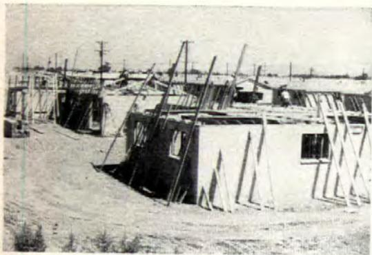
**3 Carpenters** install precut partition and roof framing, then the roof sheathing. Lumber is stacked against building within easy reach. Because he uses so many hip roofs, and because his shop-cutting is so efficient, Long feels that rafters are a better bargain in his roof construction than roof trusses would be.
