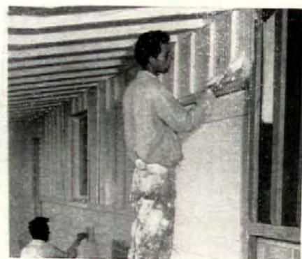
**13 Painters** work entirely with brushes. Flat finish paint is used everywhere except in baths and kitchens (and on soffits of flat-top house), which get high gloss enamel. Block walls are painted inside and out except in the kitchen, where the outside walls are furred and lined with hardboard, before being painted.
