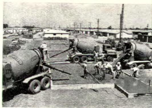
**1 Concrete crew** places transit-mix for slabs and driveways, returns few hours later to finish it. Foundations were poured the day before by the same crew. Concrete crews also pour curbs along streets. (Earlier, Long's excavation crews prepared the site and dug footing trenches with power equipment.) Plant-mixed asphalt road is also laid by Long's own crews.
