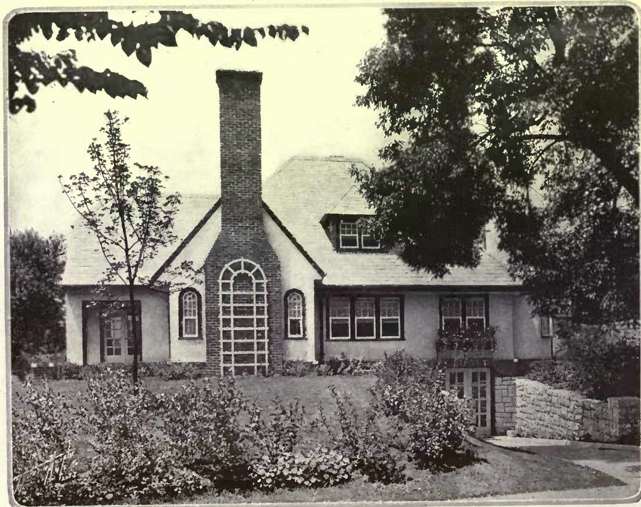
On a fairly level plot the garage entrance may be excavated to the cellar floor level, and supported by walls, as in the home of J. C. Shapiro, Kansas City. Van Brunt & Hertz, architects
