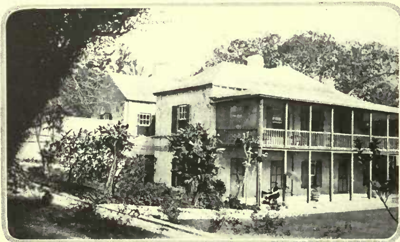
"Par la Ville," one of the old buildings of Hamilton, now used as a public library, has wide verandahs running around three sides
