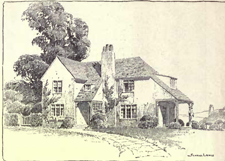
The English cottage type has no particular locality. It lends itself to stucco over hollow tile, expanded metal or wood lath. The interesting roof can be of shingle, tile or slate
