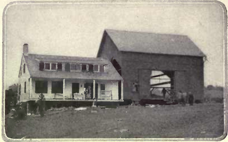
The barn and the cottage, after sliding on skids for a quarter mile and a half mile respectively, met happily on the foundations of the house destroyed three or four years previously by fire.
