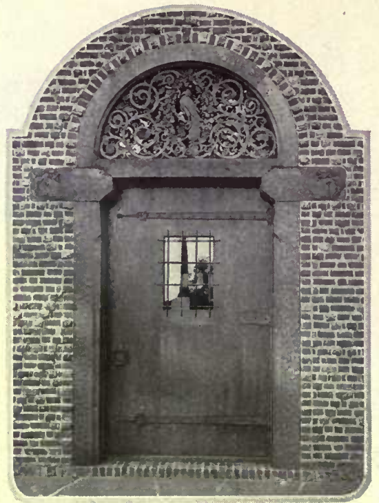
The overdoor in the residence of Frederick Humphries, Morristown, N. J., is an intricate design of birds, flowers and scrolls. H. T. Lindberg, architect; Oscar Bach Studios, craftsmen
