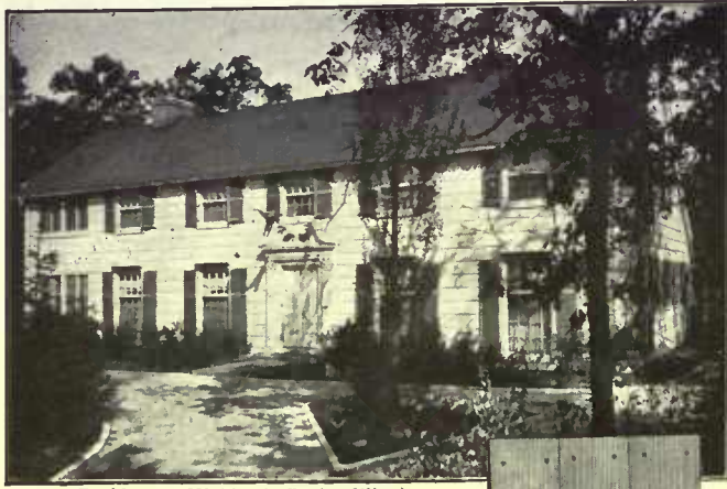
Residence, Highland Park, Illinois Robert Seyfarth, Architect, Chicago Exterior of Redwood Sawn Shingles
