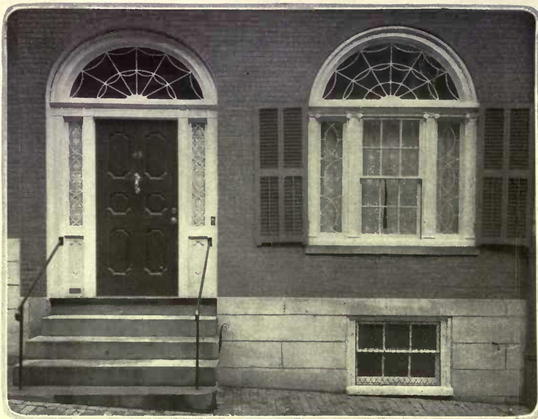
Sometimes the fanlight of the door is repeated in windows on the same façade. This early 19th Century example from Beacon Hill, Boston, has iron radiating lines with molded lead rosettes at intersections
