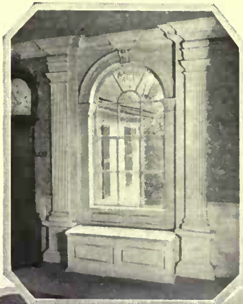
(Below) A richly designed Palladian window in the Kitt-ridge house at Andover, Mass. Built in the year 1784
