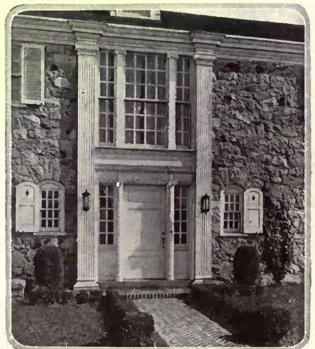
Finish is given the little windows on each side this entrance by the small pierced shutters. From the home of P. J. Gossler, New Canaan, Ct., Frederick Sterner, architect
