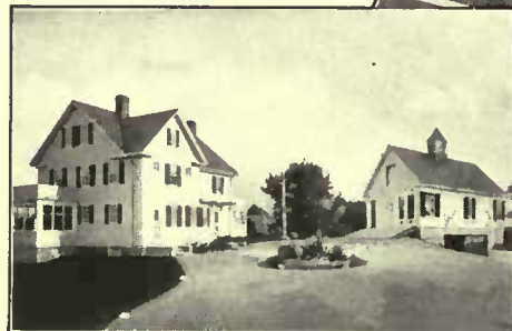
Residence and Garage at Belmont, Mass. Redwood Siding, painted white. Built by George Almgren. George Reid, Architect.
