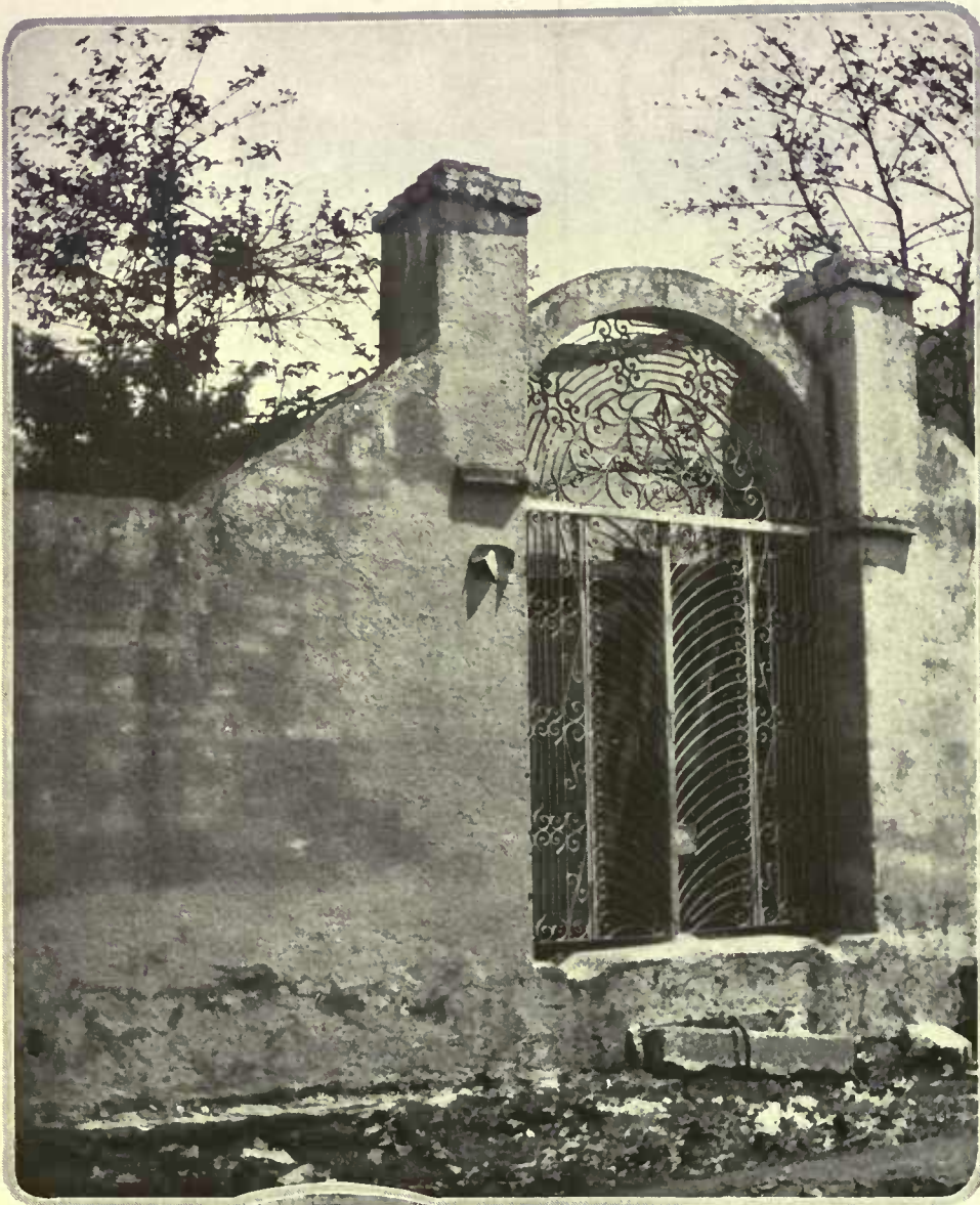
Flat iron strips were used in creating the garden grille of this gateway at Quianabacoa, Cuba
