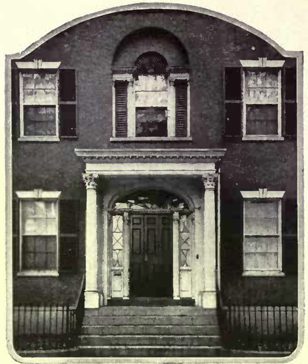
Shutters filling the side lights of the Palladian window over this Colonial entrance in Salem, Mass., are in pleasing harmony with those on the windows
