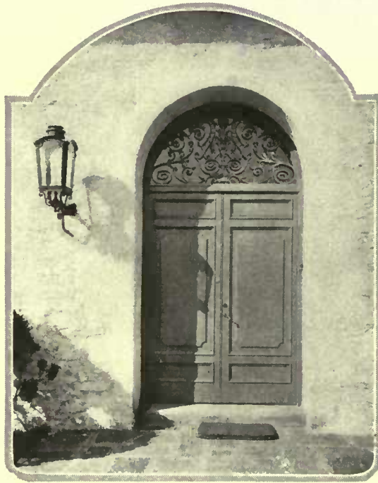
The entrance door is painted a luminous green and is surmounted by a wrought iron grille painted the same color. The arch is of stone
