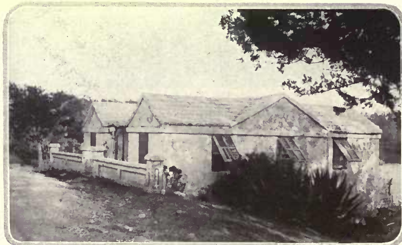
Many Bermuda houses built on a slope have the entrance on the upper story, the living quarters facing the water. These houses are of native stone
