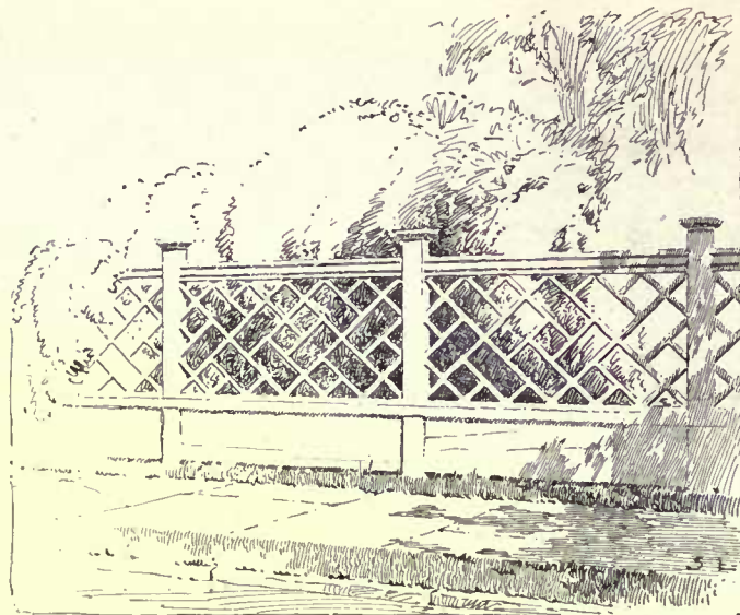
This fence from Longfellow's house in Cambridge, Mass., shows an interesting diagonal design, with a nicely made rail, and a panel below of solid planking
