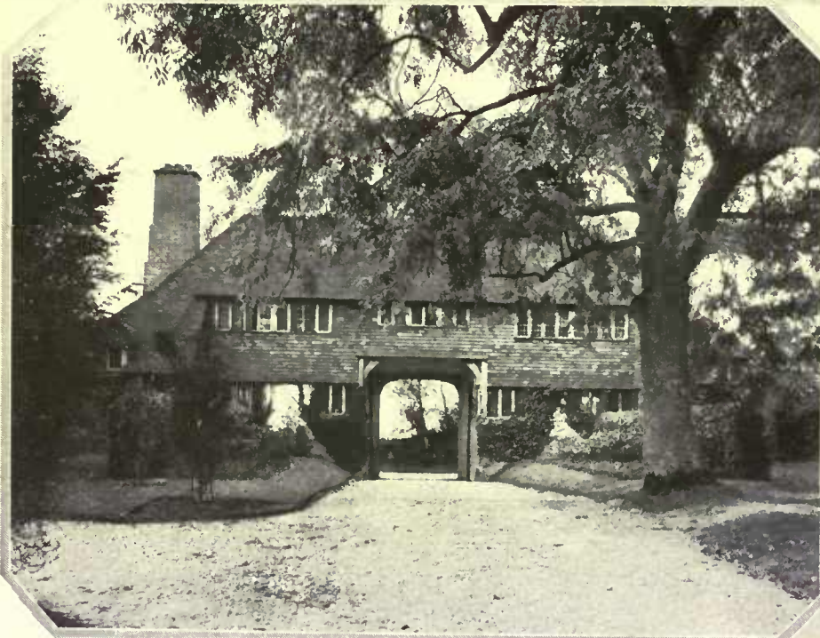
One of the most delightful entrance treatments for the large place is the lodge gate through which the approach is made to the estate. This one, on an English estate, was designed by Sir Edwin Lutyens for one of his best country house schemes
