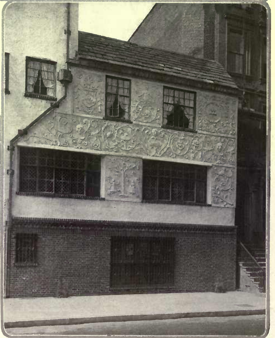
"Parge House" was so named because of the English parge work used on the extension. Leaders and gutters are of decorative cast lead. Variegated colored slate was chosen for the steep, effective roofs
