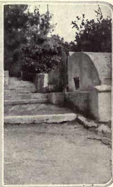
The large cistern, half sunk in the ground, is a prominent feature of most gardens. Many of them have barrel-shaped roofs
