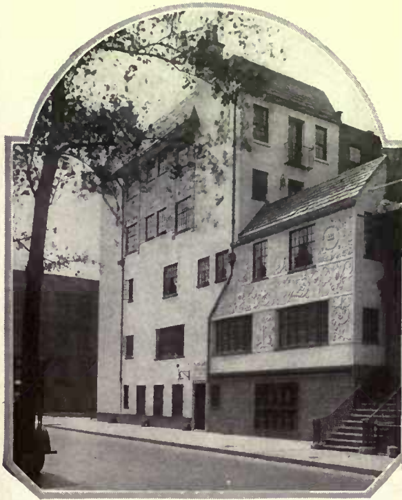
A combination of red brick, white stucco and pargetry are used in the finish of the walls. Wrought iron grills and balconies and window wood trim in green make this a colorful exterior
