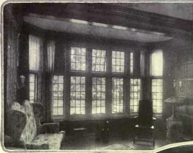
A bow-window composed of fourteen casement sash swung from various angles. From International Casement Co.
