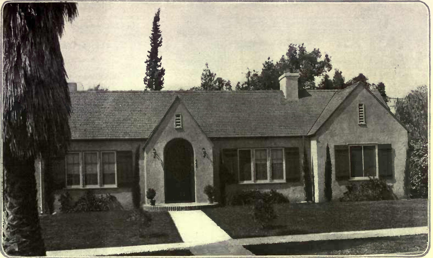
California appears to accept all types of architecture, even the small house of English antecedents. This English house at Pasadena is executed with a high pitched shingle roof and plaster walls. J. H. Woodworth was the architect
