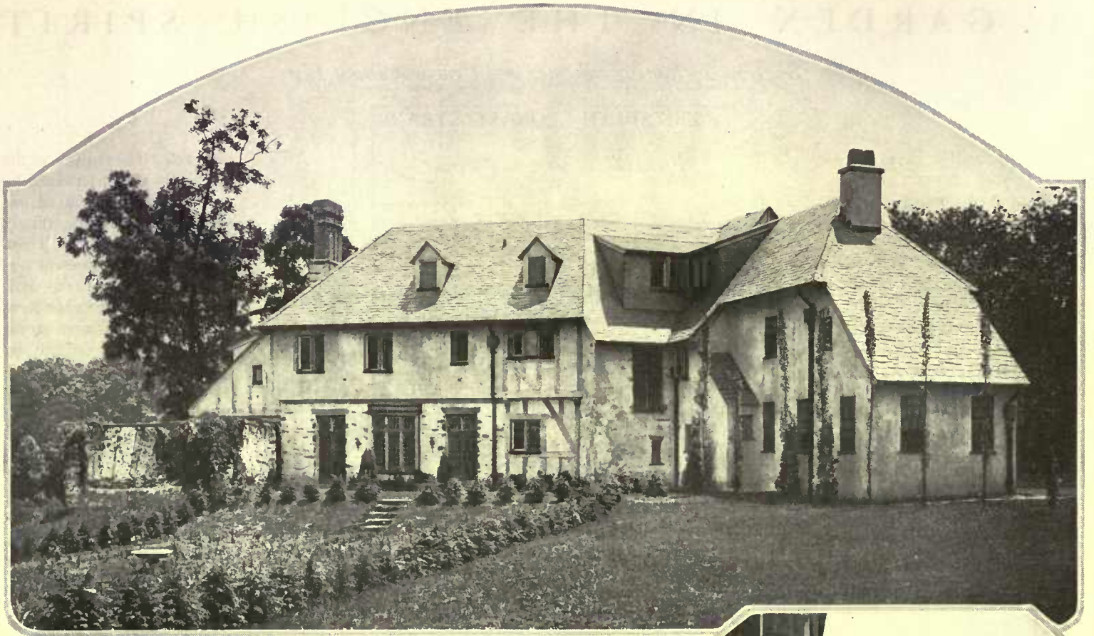
The garden is laid out in the rear of the house, on a level below the rear terrace. Among the buildings found on the place was an 18th Century Colonial residence. Part of its wall was retained to form a pergola off the living room porch. The half-timbering was built with lumber taken from dismantled barns
