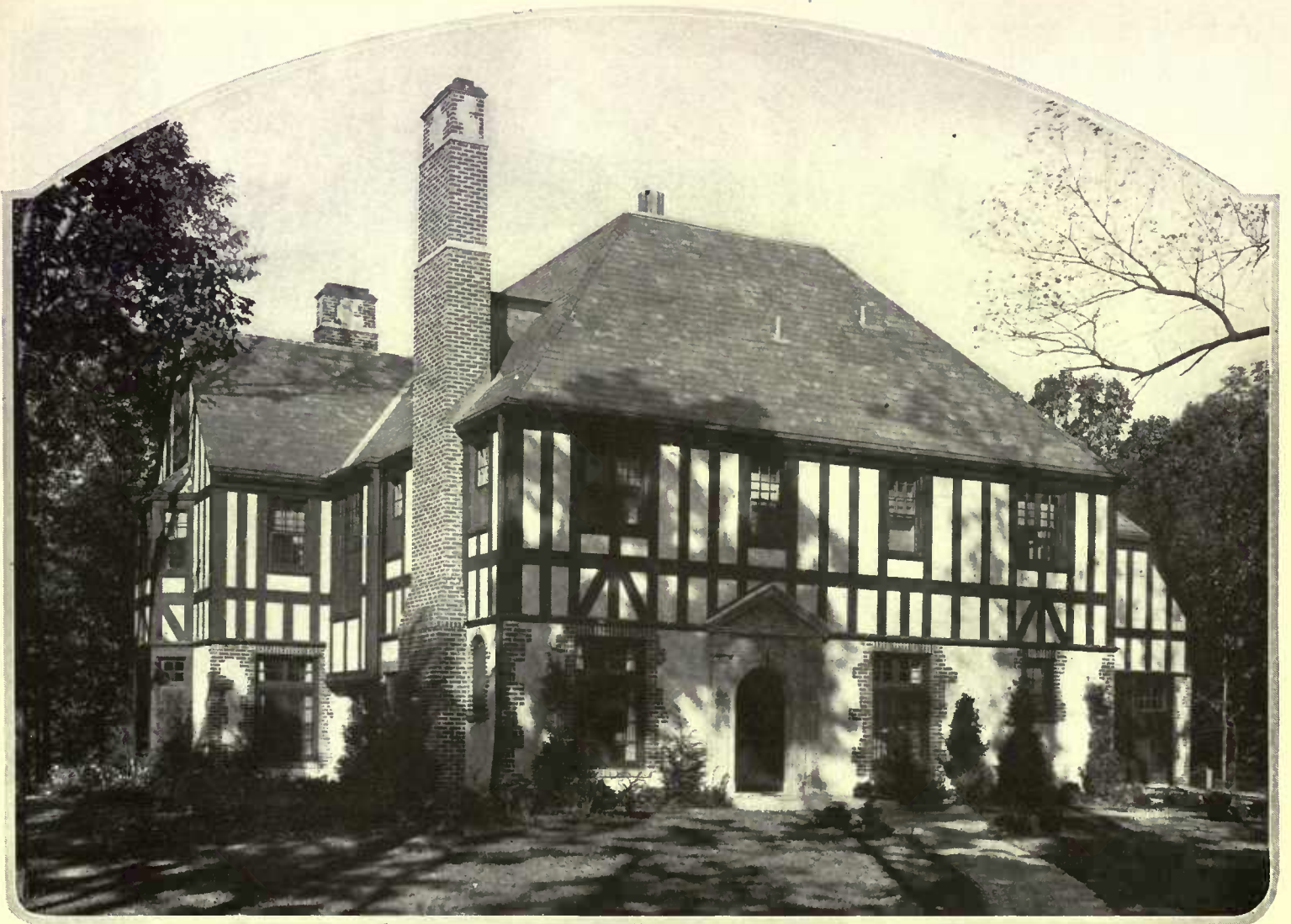
In designing the home of Henry Stanton, Winnetka, Ill., the architects, Clark & Walcott, drew on Norman and English sources for their inspiration. The combination of brick, stucco, stone and half timber makes a lively façade
