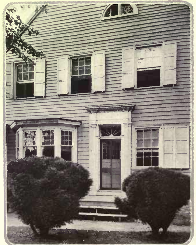
In early 19th Century work one often finds the fanlight set in a rectangular overdoor opening. This example is from a house in Salem, N. J.
