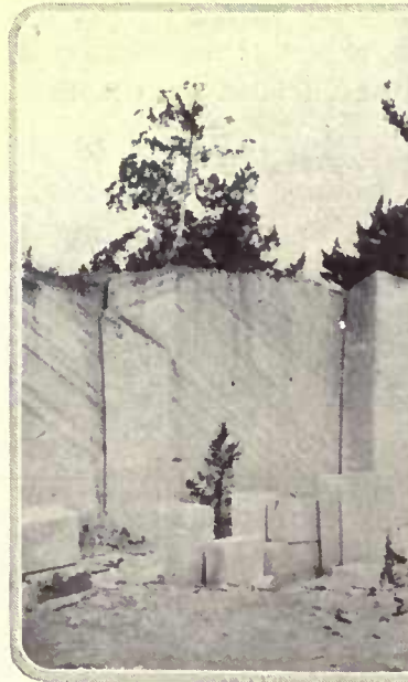
The native stone is found in large quantities, thick, of even texture and easy to cut. It soon weathers to a cool gray
