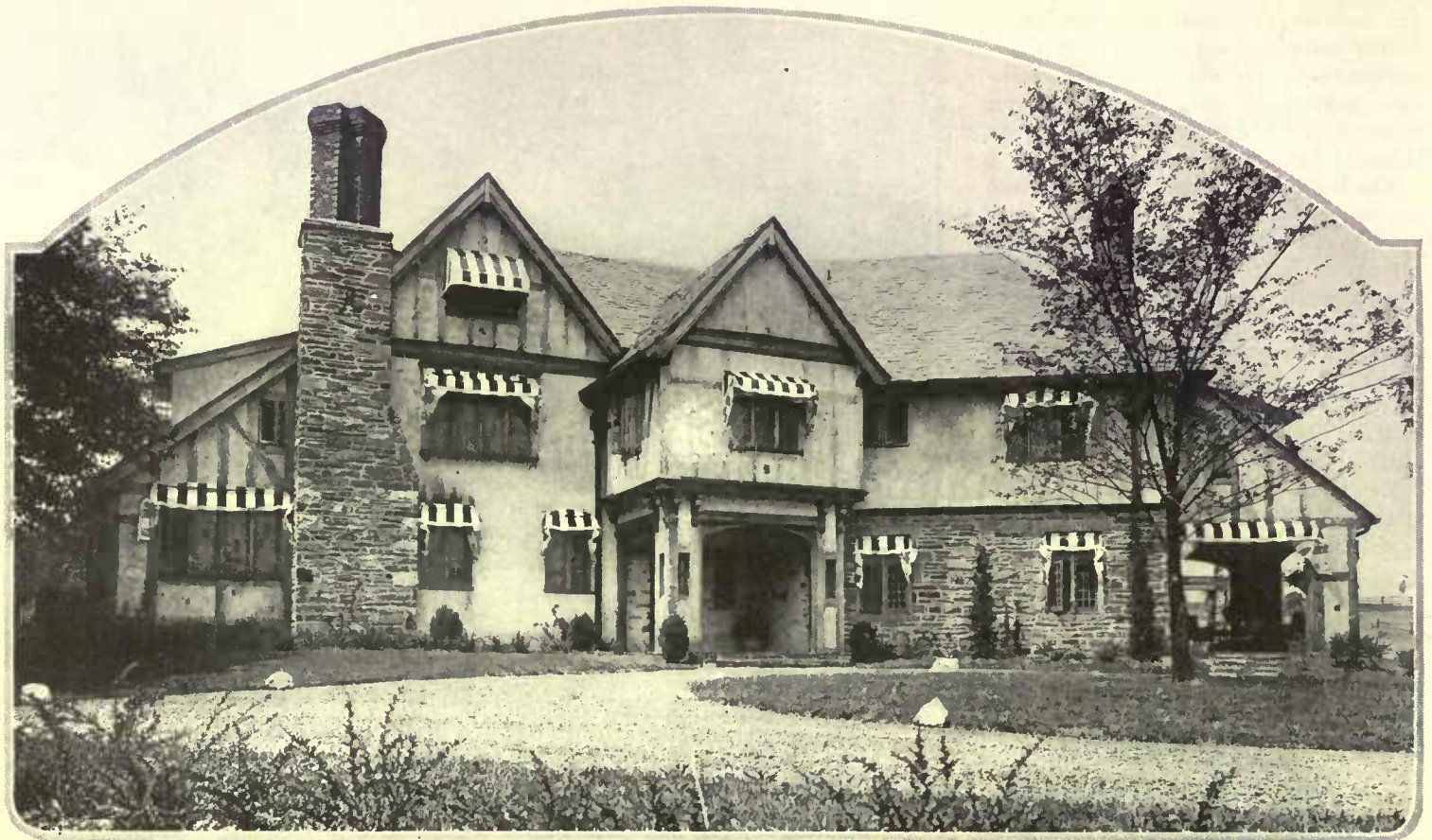
American architects do not follow traditional styles slavishly. They interpret the styles in the American architectural dialect. This residence in Pennsylvania, for example, has many characteristic English cottage elements,—the brick chimney stacks, the half-timber, the casement windows and the general feeling of the design. On the other hand, rough stucco and the stone laid up at random with wide joints in the style of the early Pennsylvania farmhouse, are local expressions
