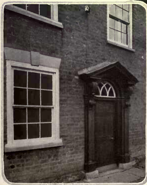
An early 19th Century doorway in the Greco-Roman mode, found in Philadelphia, has radiating scrolls approximating the fan motif
