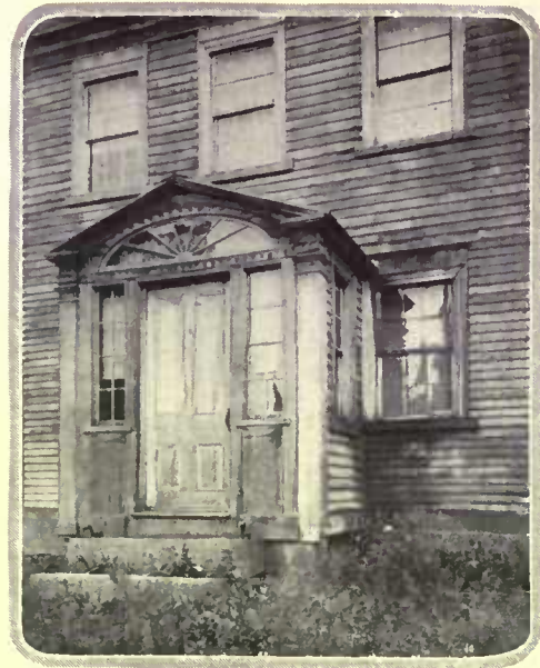
A semi-ellipse overdoor opening, found in a late 18th Century house at Marblehead, Mass.
