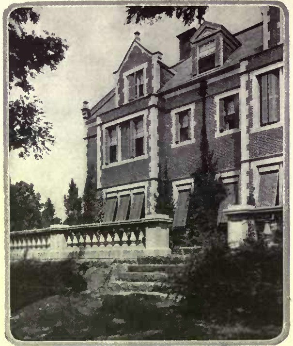
On Tudor houses shutters are out of place. Protection is given the windows by Venetian blinds or folding shutters placed inside the window casing
