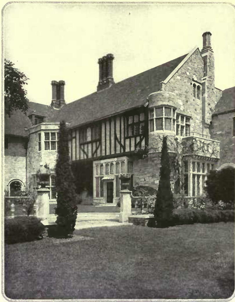
Circular Tudor chimney stacks that embellished some of the finest old 17th Century English houses are equally appropriate to the type of architecture embracing half-timber construction combined with stone, as employed by Walker & Gillette in W. R. Coe's Long Island residence
