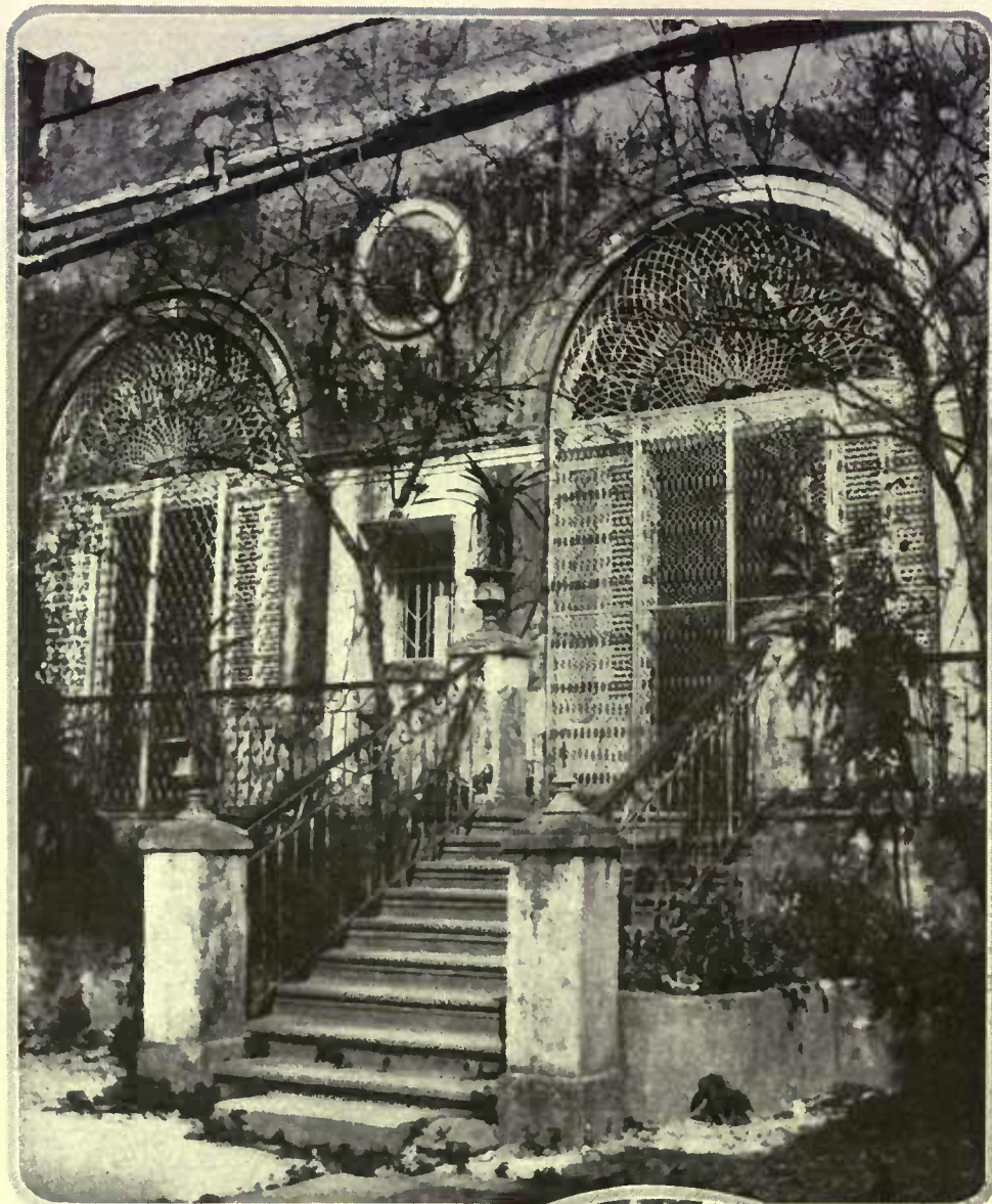
Drawn wire grilles and wrought iron balustrades are combined in this house at Matanzas, Cuba
