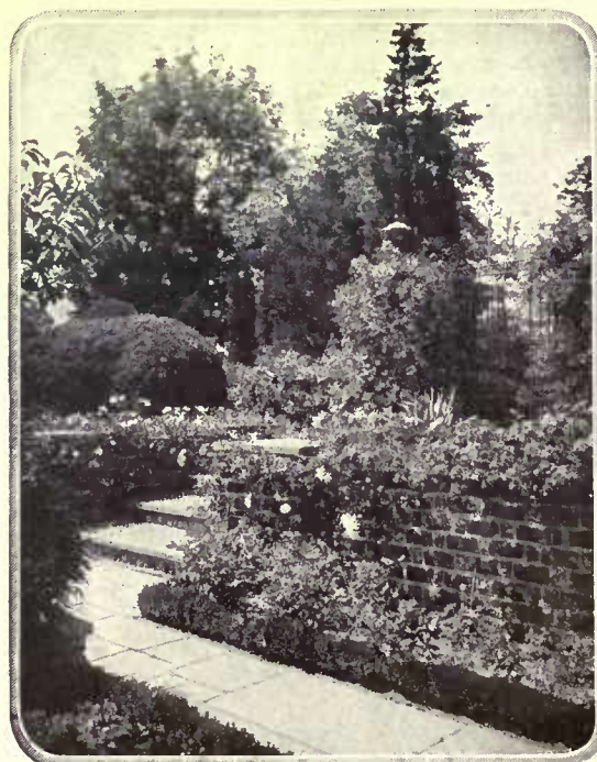
Garden roses edge the lower level of this retaining wall and creeping roses fall over from above. The step risers are of brick on edge to match the wall, and the treads are of slate
