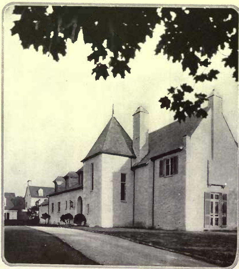
An agreeable texture is given the walls by the plaster being roughly floated over rubble. The shutters are painted a light green. The corbelled chimney base in this end indicates the position of a bedroom fireplace
