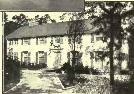
Residence at Highland Park, Ill. Redwood Special Sawn Shingles, painted white. Robert Seifarth, Architect.
