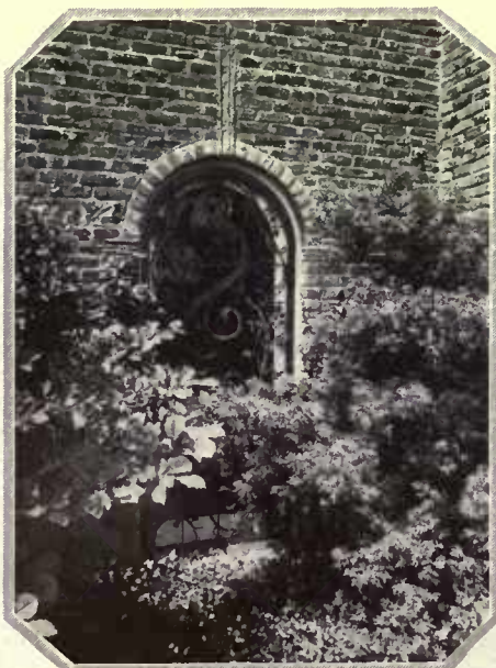
The peacock window grille designed by H. T. Lindeberg, architect; Oscar Bach Studios, were the craftsmen
