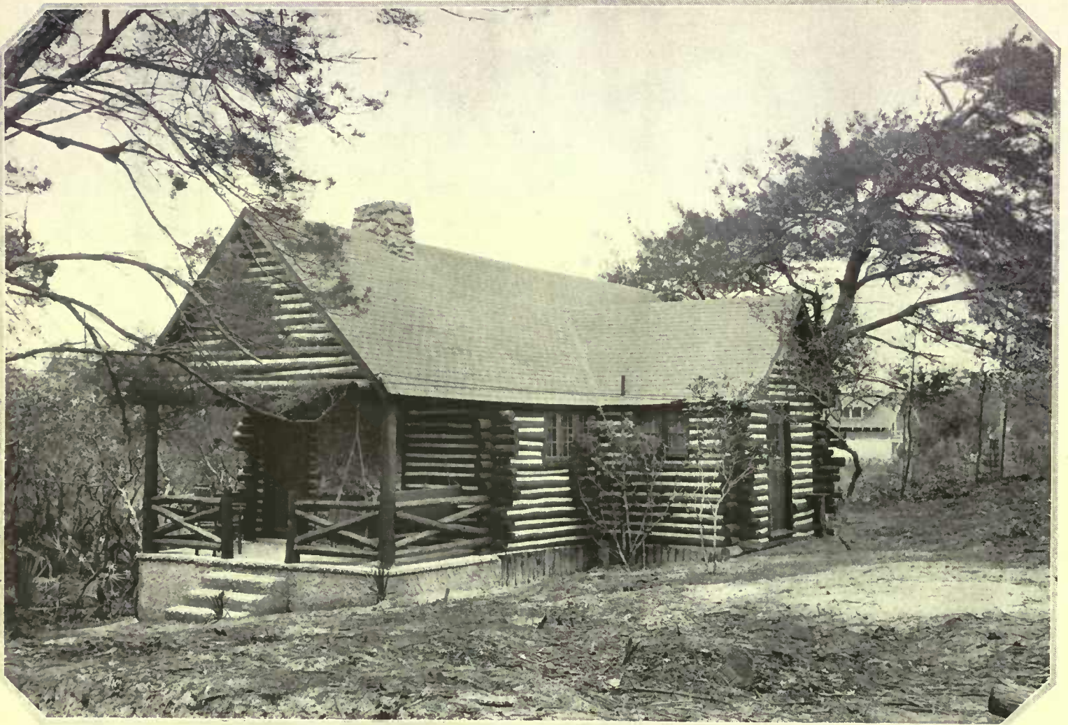
Cement caulking was used in this log cabin in Sea Breeze, Florida, designed by Frank J. Forster, architect. The doors are batten, windows are casement
