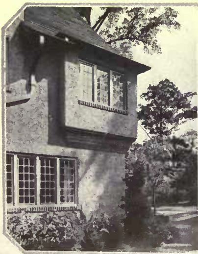
A variation of the bay window in a house at Spuyten Duyvil, N. Y., designed by Julius Gregory
