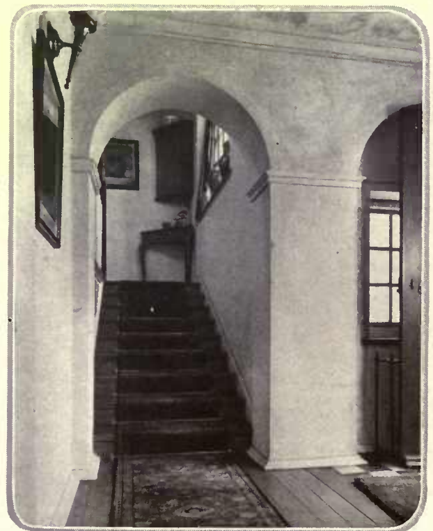
In developing the open first floor plan, which is found in many sections, the arch supplants the door. It is effectively employed here to give access to the stairs and to repeat the arch motif over the adjoining window
