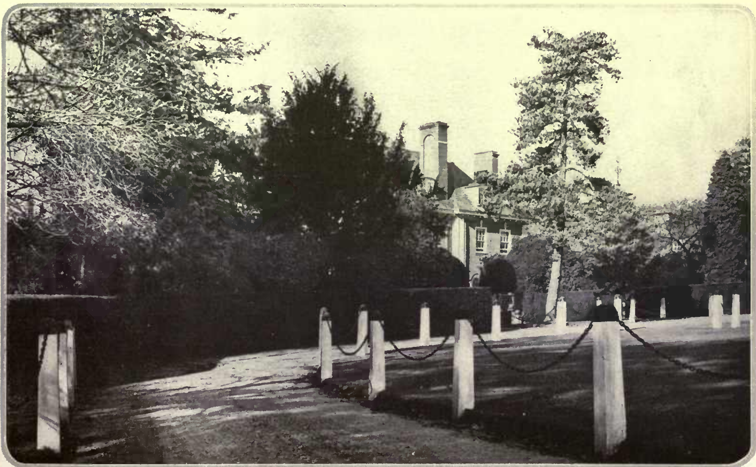
In the approach to this English country house the entrance drive as it skirts the lawn in front of the forecourt is flanked by a popular British device—the post and chain fence; an arrangement at once serviceable
