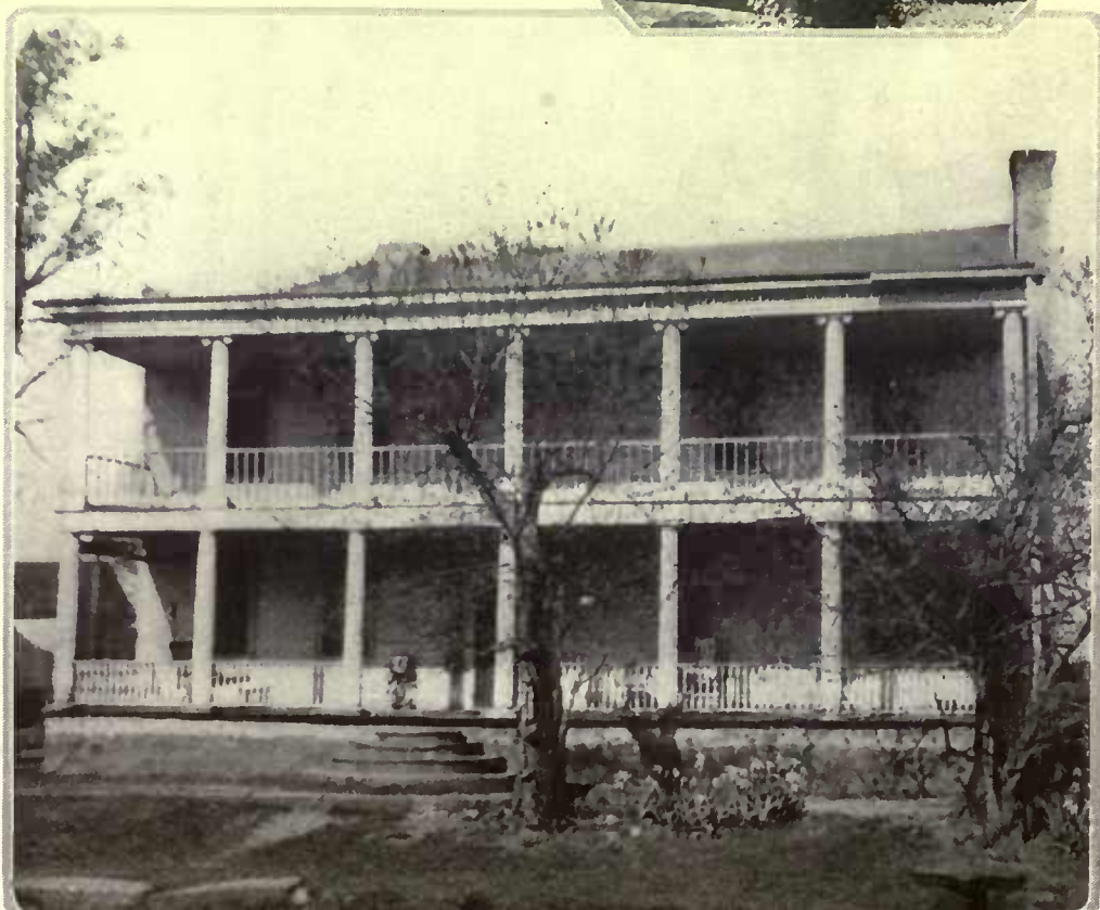
This house in Clinton is interesting for its two story porches of super-imposed orders, delicate cornice and steps of old millstones
