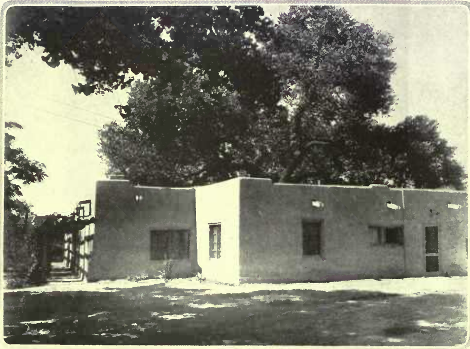
This old adobe house, modernized inside, has just been freshly coated by the Indian women with salmon coloured plaster. The walls are 3' thick, allowing deep window ledges. Spanish gutters drain the roof
