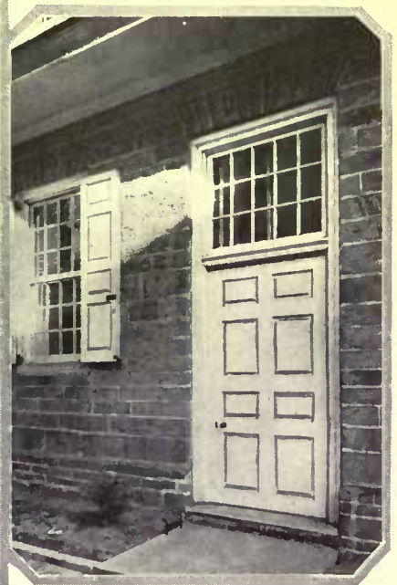
This sturdy, well proportioned entrance of the old courthouse at Chester, Pa., is typical of the best 18th Century paneled door
