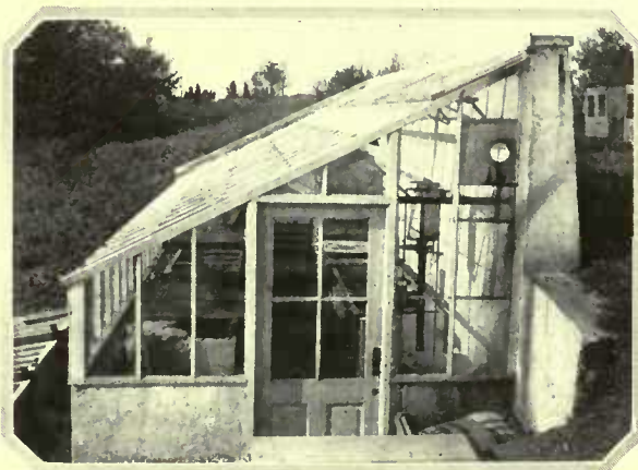
Where the side of an existing building is not available, a back wall for the lean-to greenhouse may be constructed of concrete. In this case the partial sinking of the house lessens the amount of artificial heat required.
