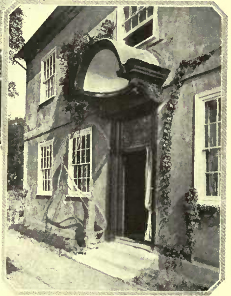
The doorway to this house, built in 1690, depends for its distinction upon the hood. It is painted dark brown, the plaster cove white and the wall stucco
