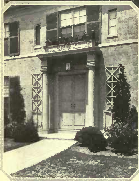
Flanking lattices and slender cedars set off the entrance whose classical feeling is continued into the flower box above. Perfect balance obtained throughout
