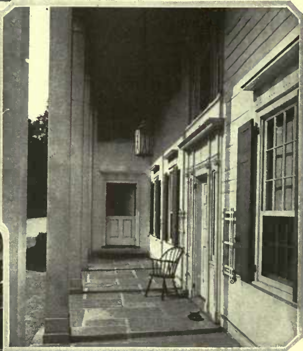
The veranda is a feature of Southern Colonial architecture. As shown here, it is made by recessing the middle unit of the house and supporting the roof on tall columns. Dwight James Baum, architect
