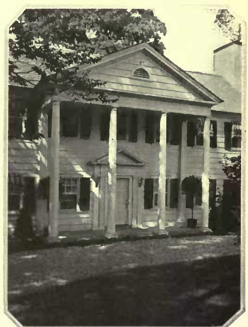
A high porticoed entrance gives the front façade fine dignity besides creating a brick porch and approach to the entrance door
