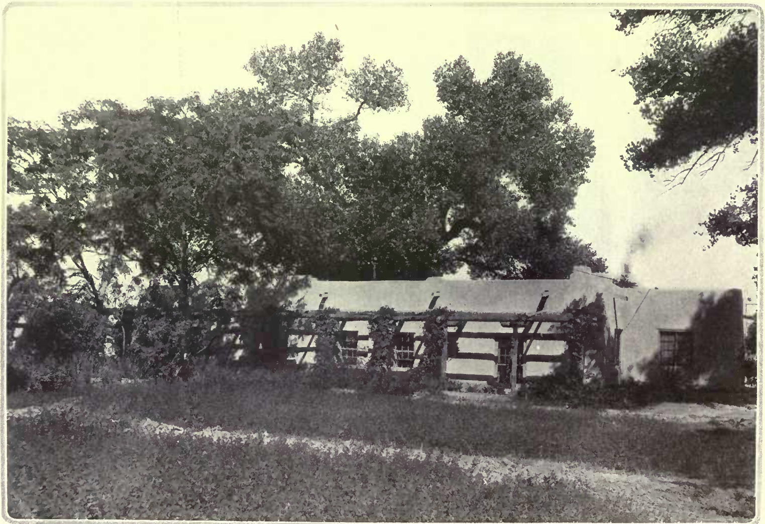
This old adobe house, modernized inside, has just been freshly coated by the Indian women with salmon coloured plaster. The walls are 3' thick, allowing deep window ledges. Spanish gutters drain the roof
