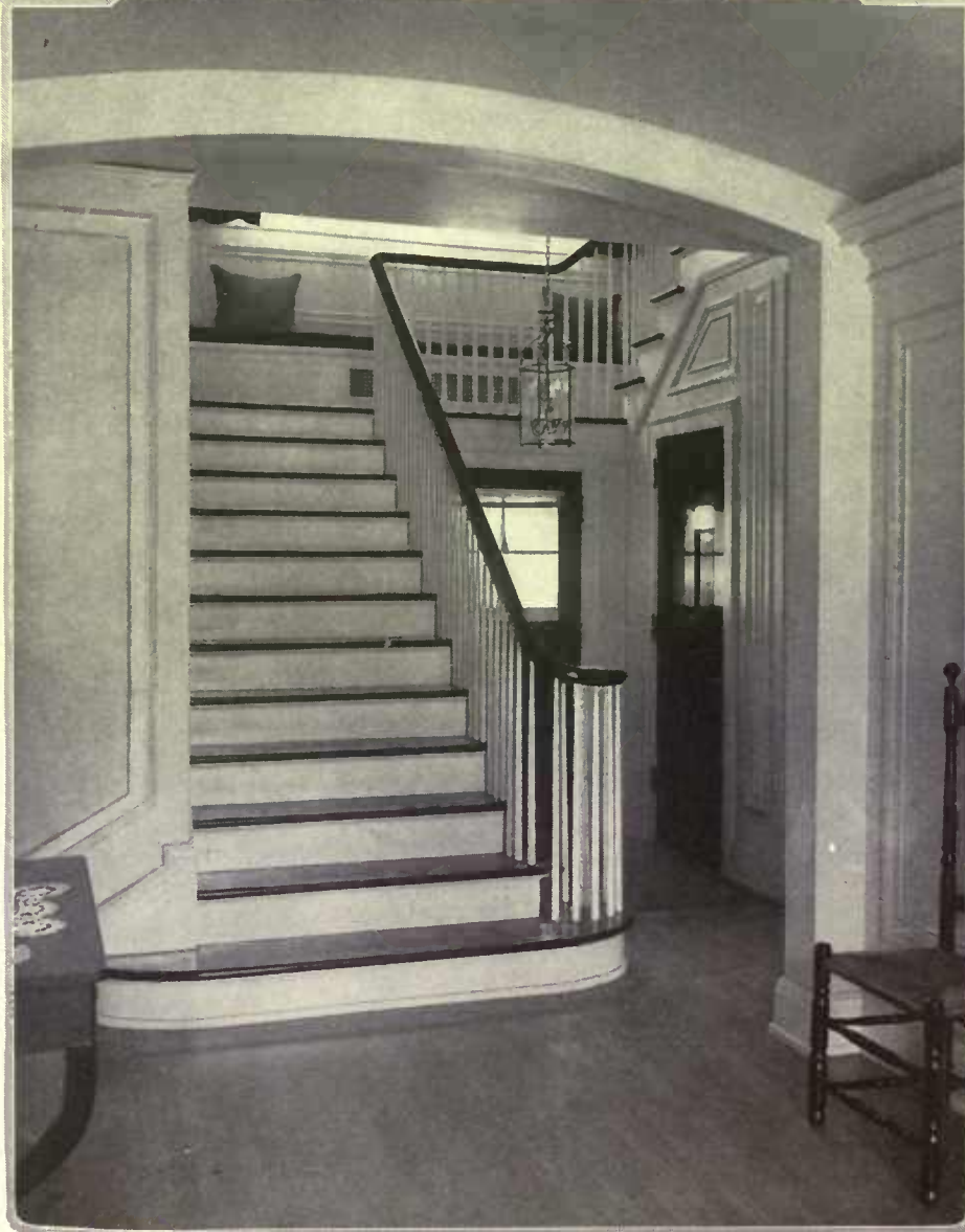
Stairs should be easy to ascend. This ease depends upon the height of the risers, the width of the treads and upon the position of the landings. All three are excellent in this example
