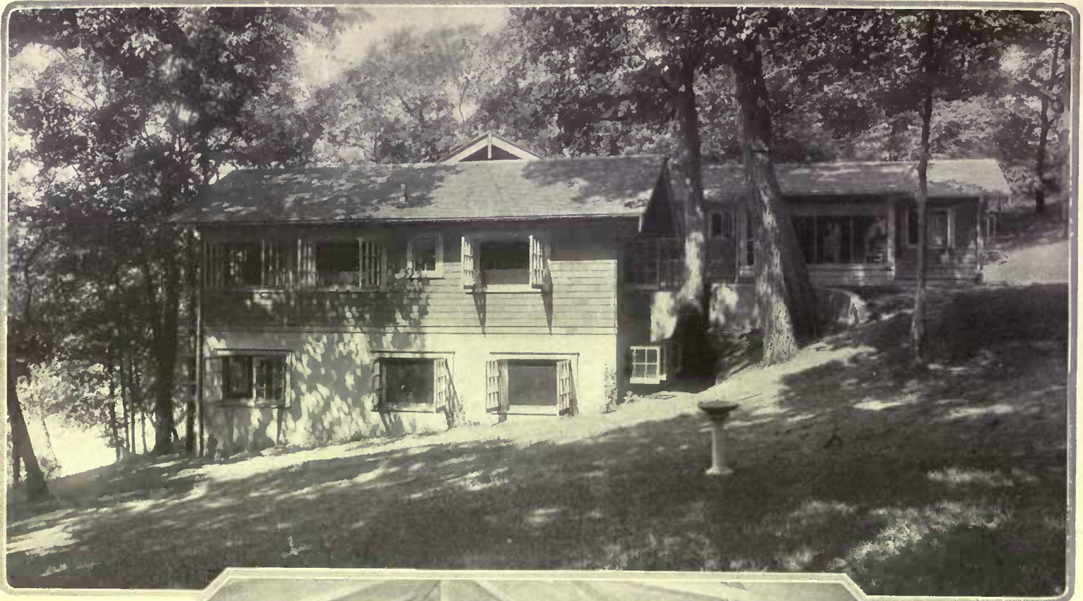
The slope of the land permitted two levels, the lower built of concrete, the upper shingled. A retaining wall protects the old trees that shadow the house on this southern exposure
