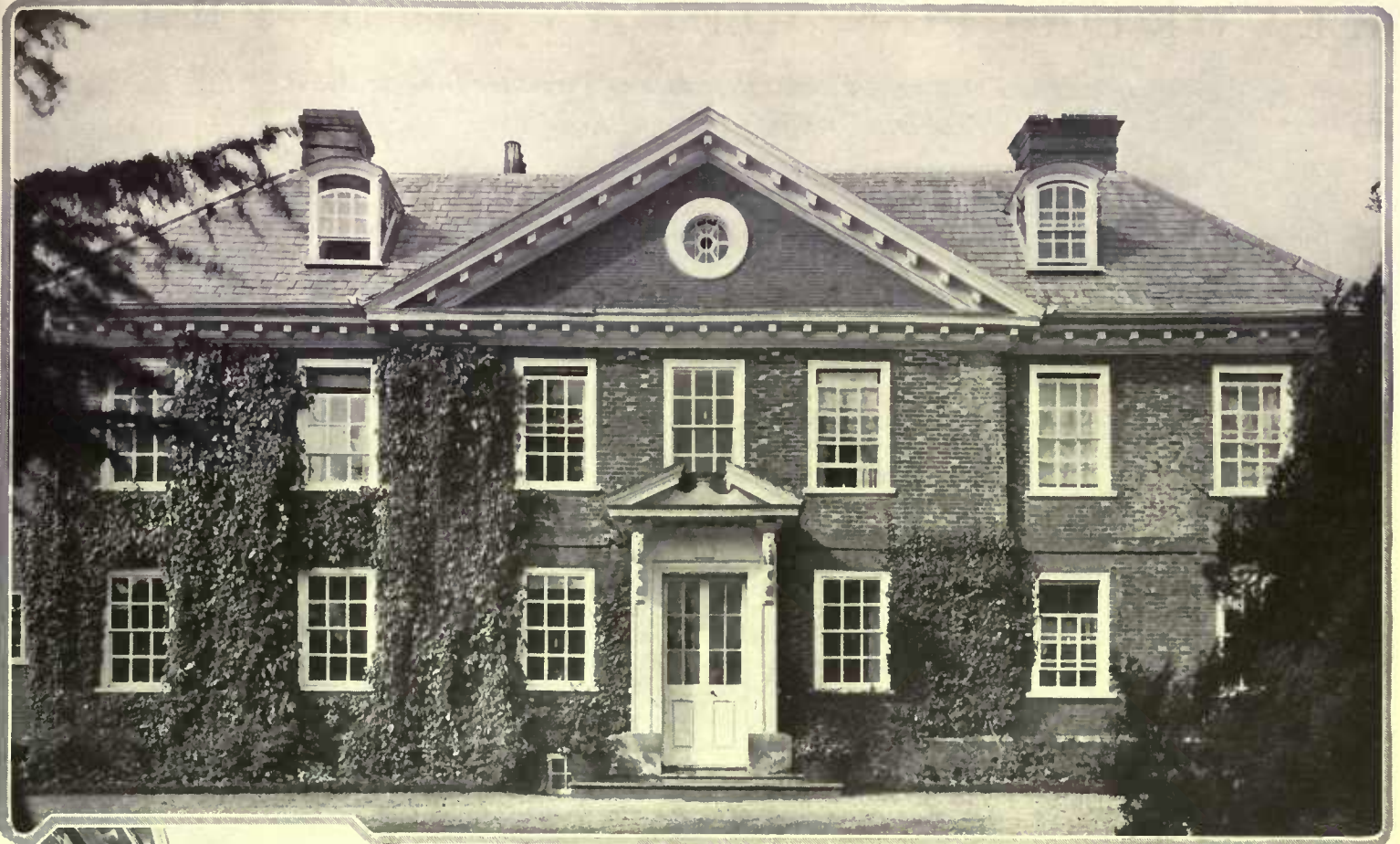
The entrance side is quite different from the garden front. The brick is laid in Flemish bond, the central projection is wider, and there is a belt course between the first and second floors
