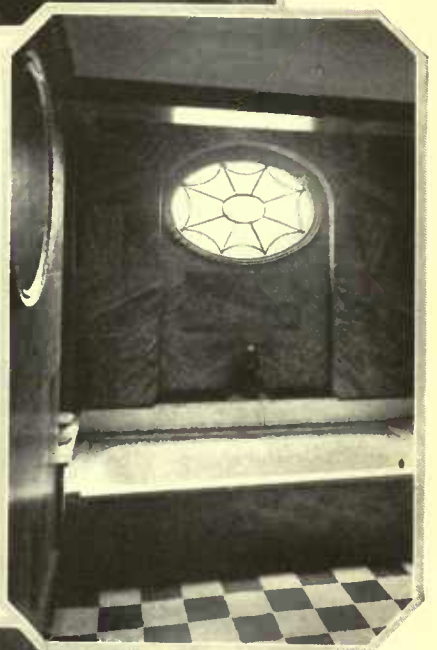
The tub can be partially sunk, as in the room to the right. The floor is covered with composition tiles and the walls with composition stone
