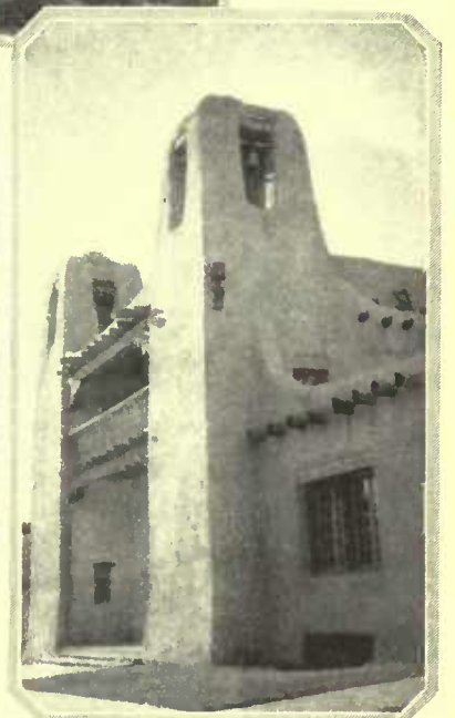
The buttressed towers, projecting roof beams or vigas and rounded walls are pueblo features reproduced in this modern building
