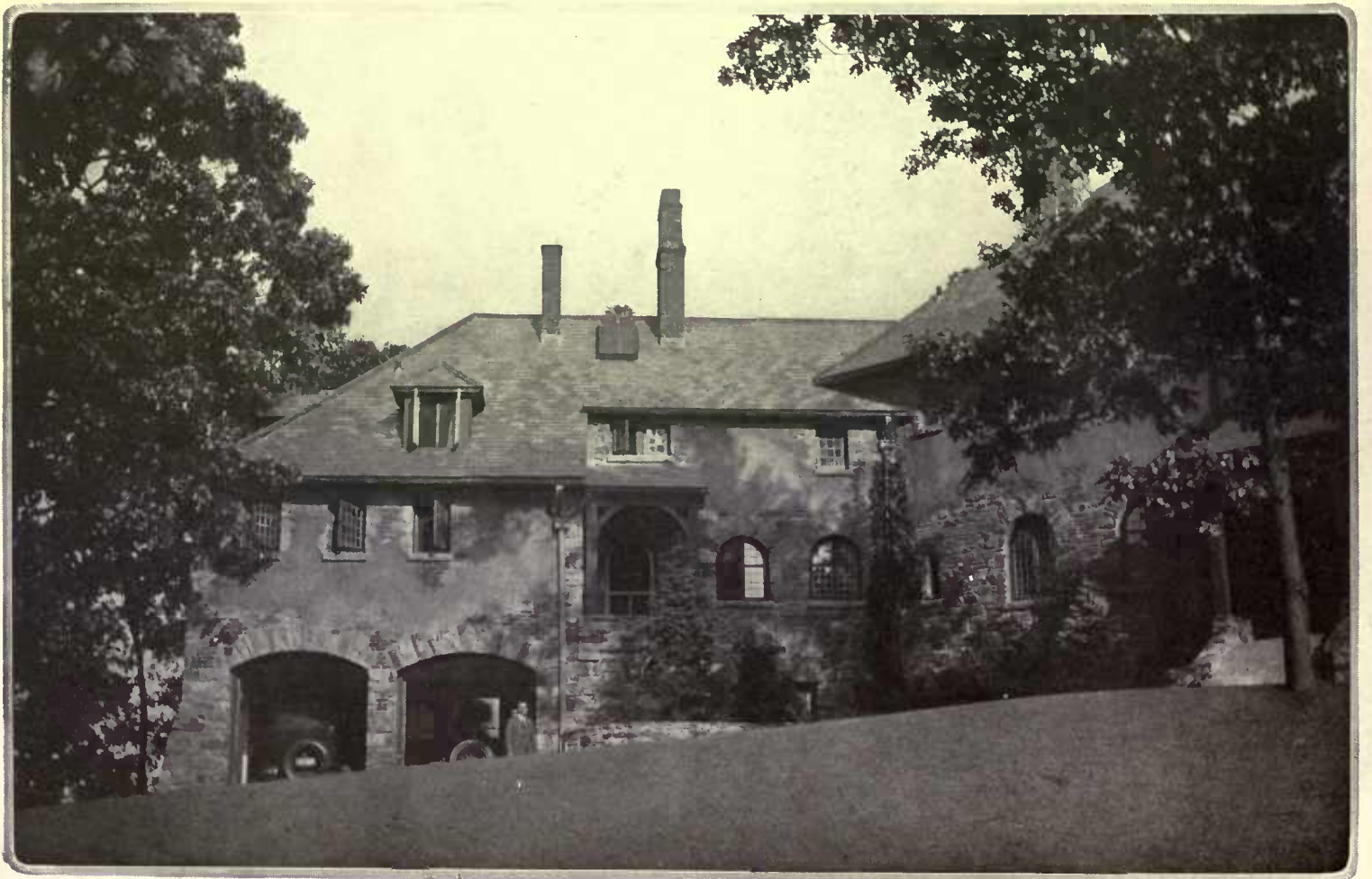
(Above) On the northwest side one can see indications of Tudor influence in the detail of the house—the oriel window, for example, and the overhang of the sleeping porch. Although the roof appears complicated, it is really massed for climax, in a steadily mounting series of hips and ridges
