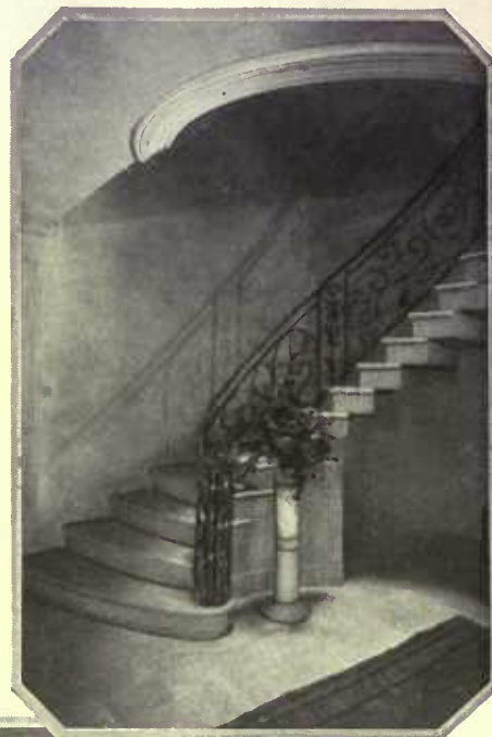
Curved free standing stairs or stairs supported on only one side have an undeniable lightness and grace. In this example from a New York house the stone steps are surmounted by a wrought iron balustrade and railing of great delicacy. William F. Dominick, architect
