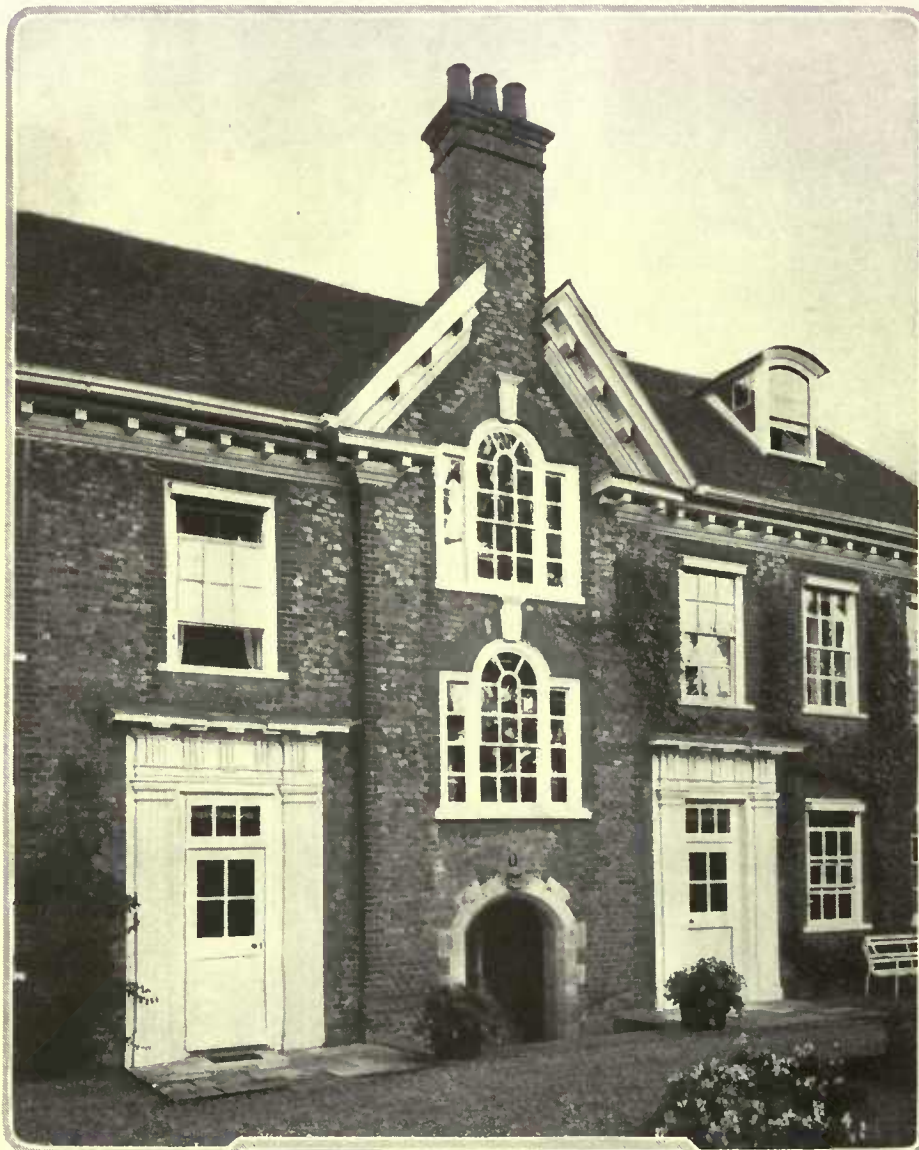
An arched cellar entrance, superimposed Palladian windows, brick laid in header bond and glass-cheeked dormers are among the unusual features of the garden front
