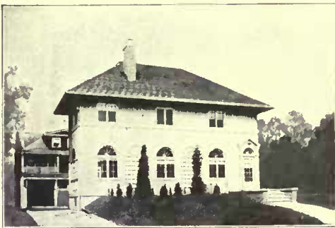
Residence—1839 Farrington Rd., E. Cleveland, O. Owners, Arc'ts and Bldrs.—The Joseph Larong Co. Bishopric used on all exteriors or interiors
