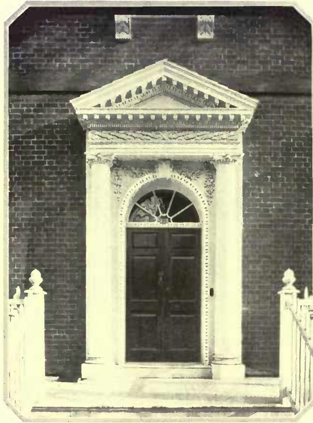
This severely classic old Annapolis doorway combines with its pure Greek pediment and elaborated Doric columns an unusual decoration of swags on the doorhead
