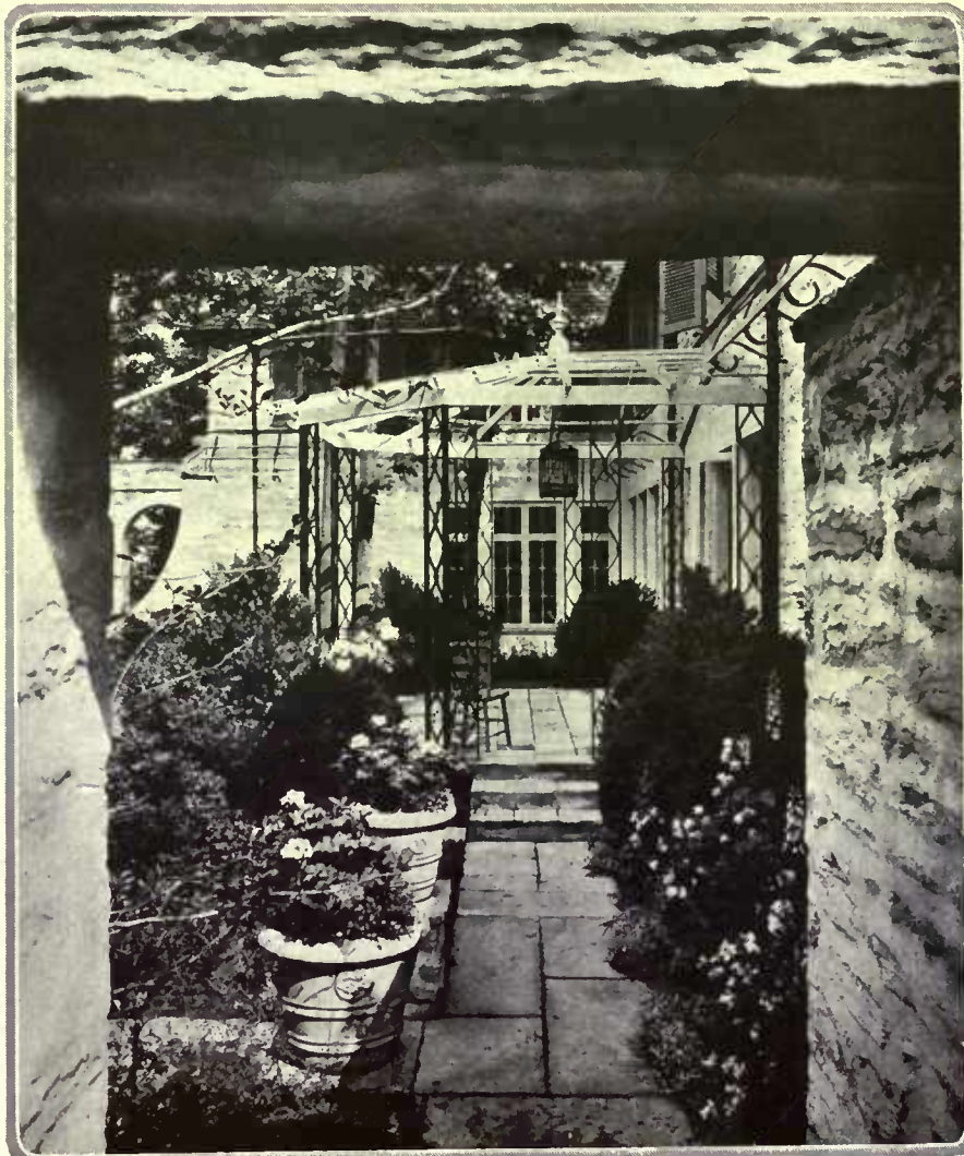
The combination of decorative black wrought iron standards and white wooden open roof creates an atmosphere of airy grace in this porch on the residence of Mrs. B. F. Pepper at Chestnut Hill, Pa. A stone floor continues the stone of the garden paths. Willing & Sims, architects
