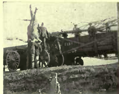
Loading a 20 year old shade tree
