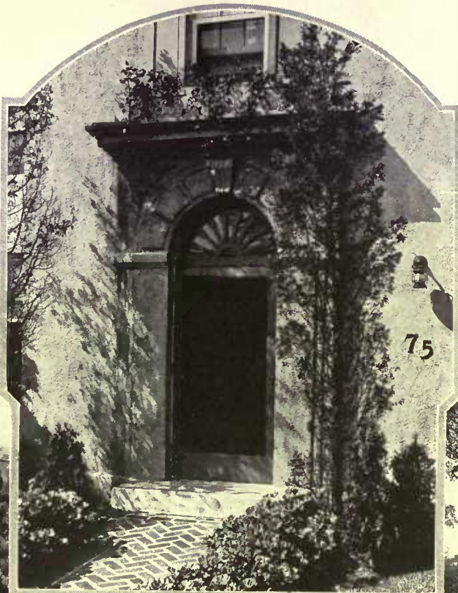
A sympathetic adaptation of a romantic Italian doorway for a modern house is of plaster, moulded into decorative effects. The half circle light and the wide moulding above make a dignified finish for the design
