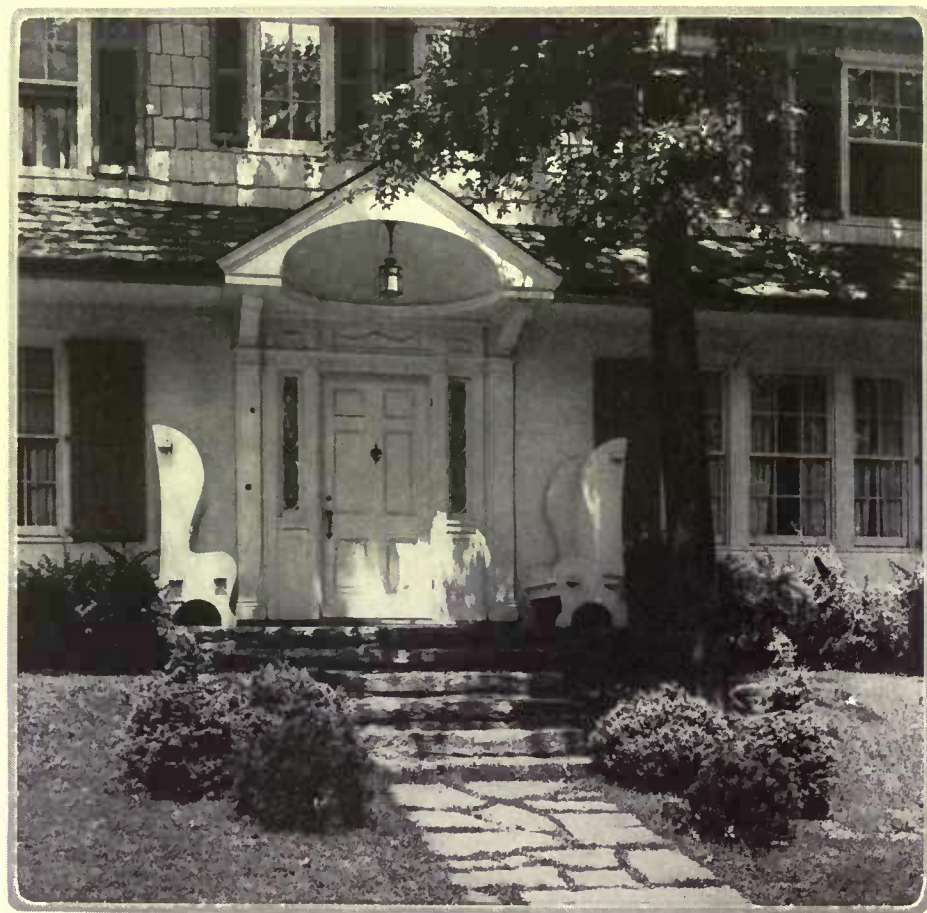
The pent house and Germantown hood are merited revivals of a Colonial style. Adapted here to a modern house, the hood is well placed in relation to the windows, projecting roof line and open porch. The hospitable high-back settles are architecturally important to the house design. Tooker & Marsh, Architects
