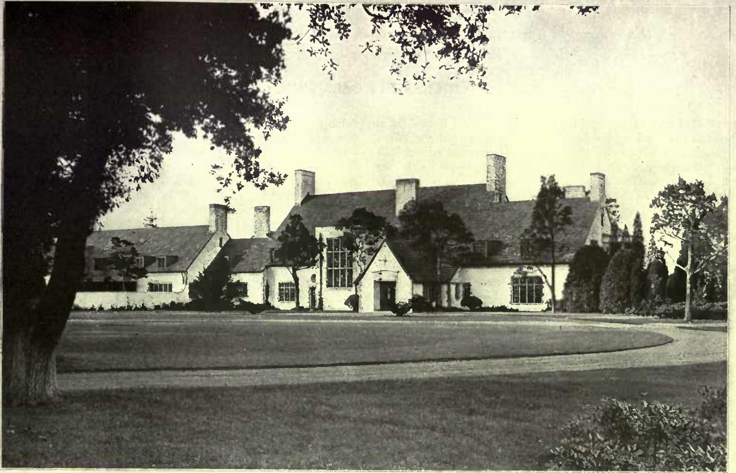
A long, low roof line has been created by attaching the garage and servants' quarters to a wing of the house. A brick wall separates the service yard from the entrance. An unusual feature of this front is the square stair well
