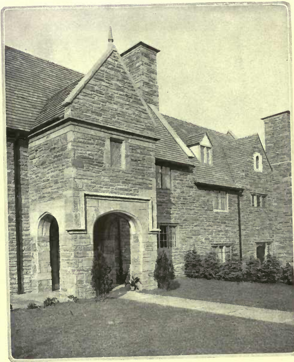
Both the porch and the chimneys of this house at St. Martins, Pa., are made effective by a careful disposition of moldings. They create shade and are a relief to the flat surface of the wall
