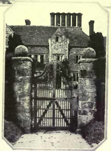
A view of the house from the front. Though seeming old the gates and posts are modern and were designed by the architect, who made considerable alterations to the house and also laid out the formal rose garden illustrated above
