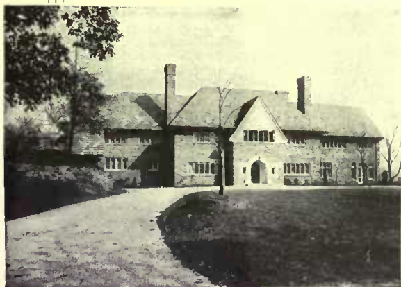
The H. S. Pogue Residence, Cincinnati, Ohio G. C. Burroughs, Cincinnati, O., Architect
