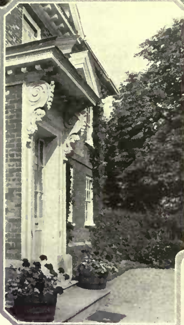
Apart from the round window in the wall of the pediment the entrance front is soberly devoid of decorative detail, except in one instance—the carved brackets of the door, depicting cherubs
