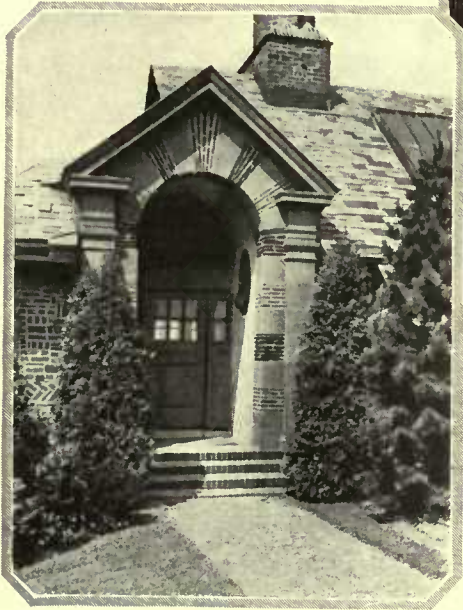
An unusual doorway designed by Donn Barber suggests Greek inspiration, with its Doric pilasters and pointed hood. A frame of plaster has inserts of brick
