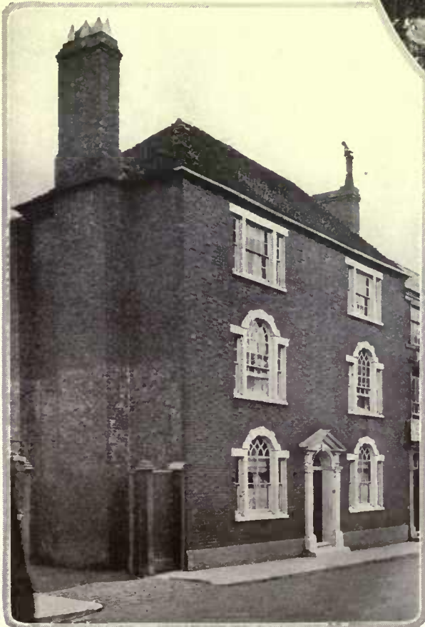
(Below) Proper glazing is a requisite of Palladian windows. Compare the modern large and ugly panes in the first floor with the small panes on the second
