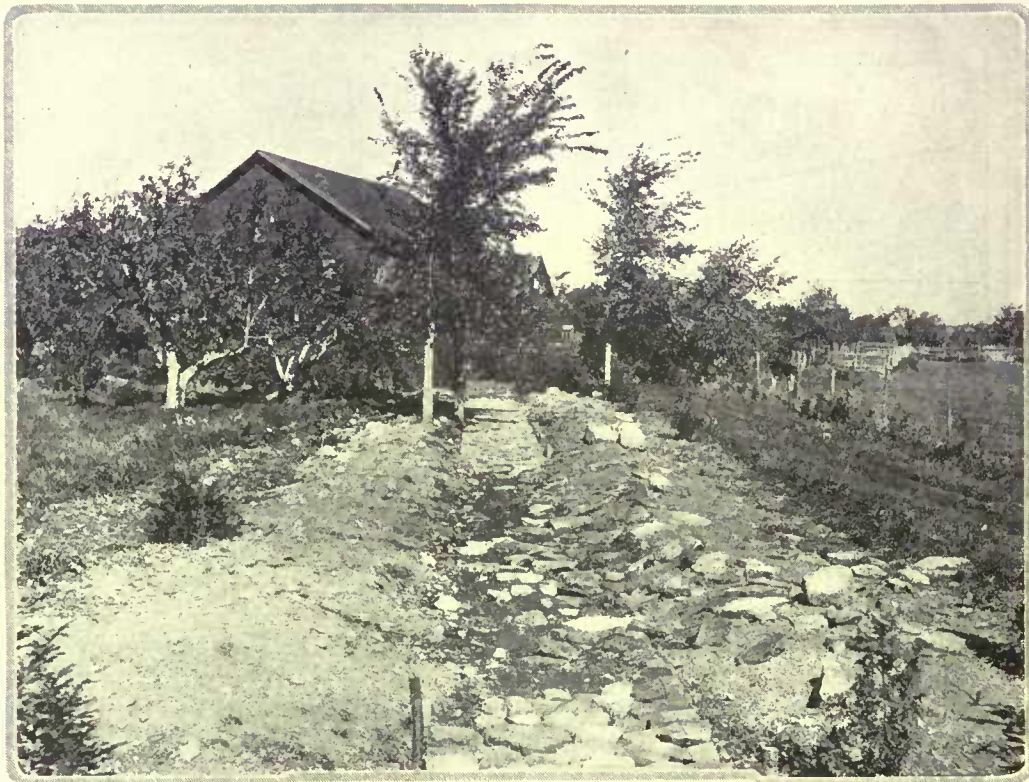
Early the following spring the site was plowed, harrowed and leveled. By September a number of evergreens had been set out, and a shallow trench the width of the proposed walk partly paved with flat field-stones gathered from walls, lanes and pastures
