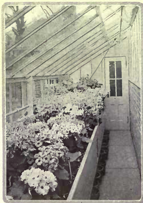
The lean-to type, which utilizes the wall of an existing building for its back, is practical and inexpensive. A southern exposure is best. Courtesy of Lord & Burnham
