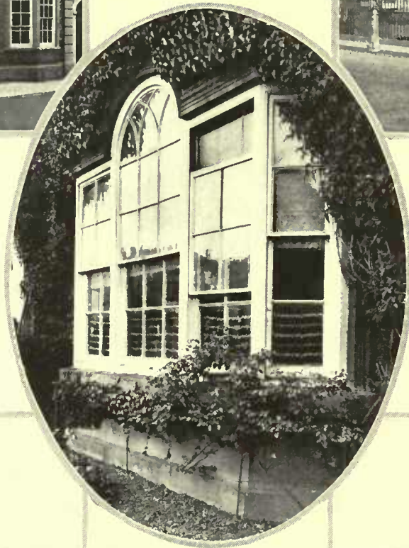
An ingenious application of the Palladian motif to a bay window is seen in this house at Buckingham. Additional flanking lights make the window a five-light composition
