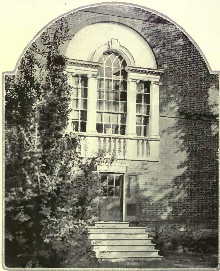
On the garden front of the Chase House, Annapolis, Md., the Palladian window is the central feature. The window is set in an arch and supplemented at the bottom with a balustrade
