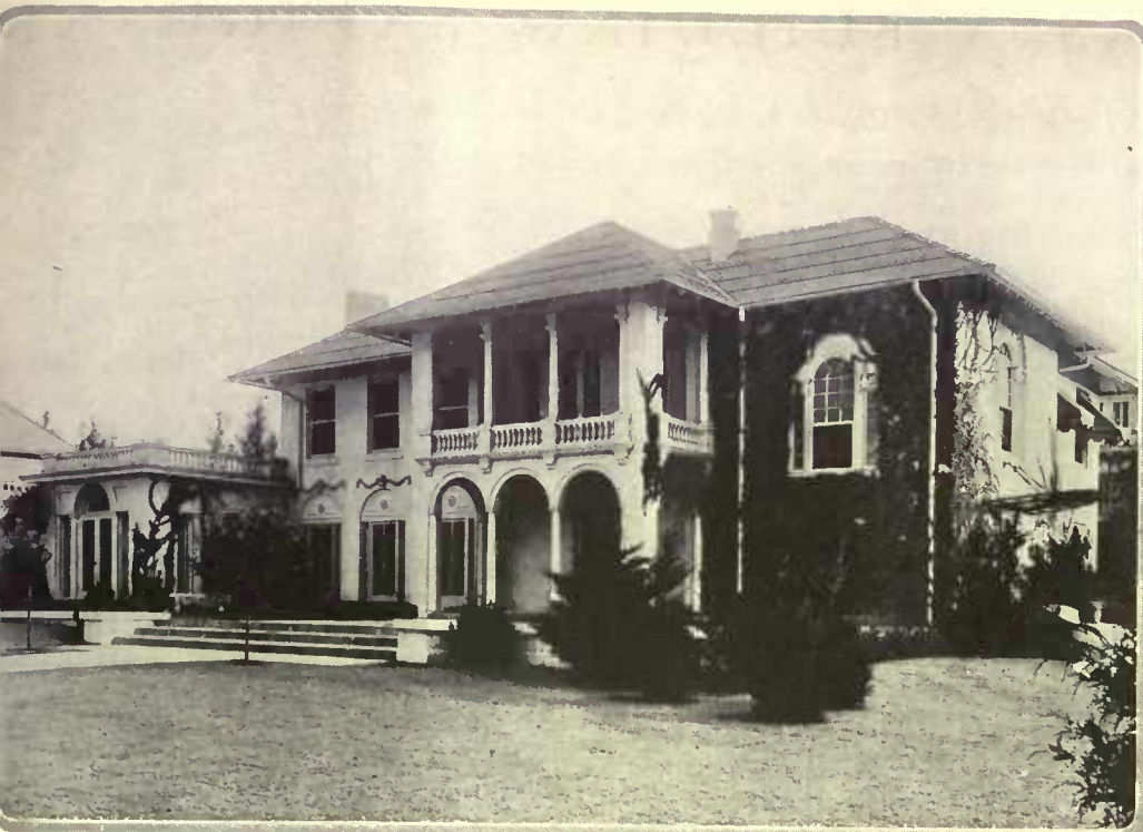
Climate is often a deciding factor in architecture. Designs are adapted to suit local climatic conditions. Thus, in this home of Edgar L. Flippen, at Dallas, Texas, the Italian style has been used with local modifications. It is stucco over hollow tile. H. B. Thomson, architect
