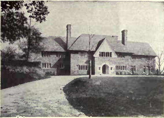
The H. S. Pogue Residence, Cincinnati, Ohio G. C. Burroughs, Cincinnati, O., Architect
