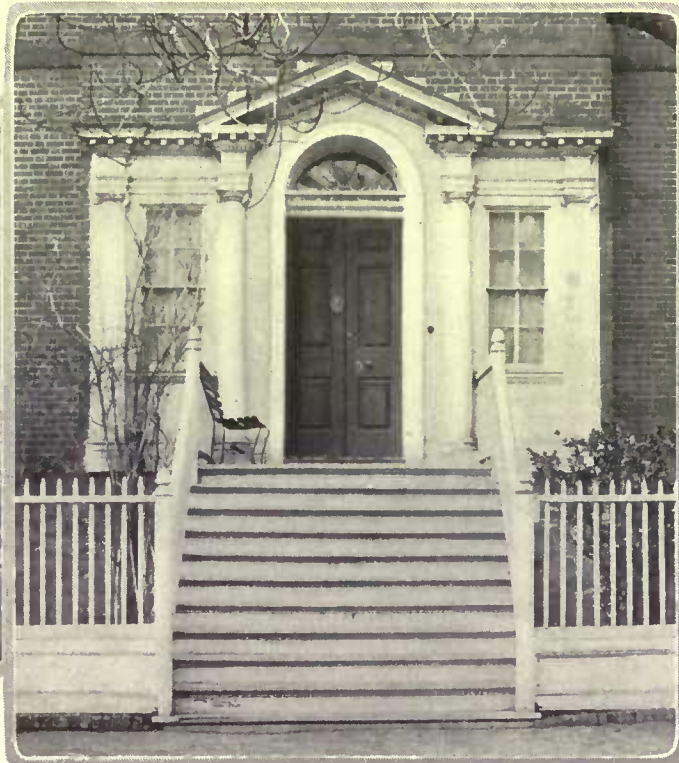
Great distinction is achieved in the richly designed doorway of the Chase House at Annapolis, Md. The Palladian motif appears in the combination of windows and door, bringing spacious beauty to the entrance
