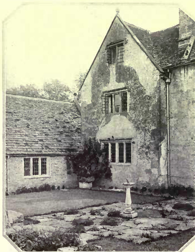
Stone window frames with leaded casements is the traditional style in England. This example from Biddesdon Manor, Wilts, shows a graduation of sizes toward the gable
