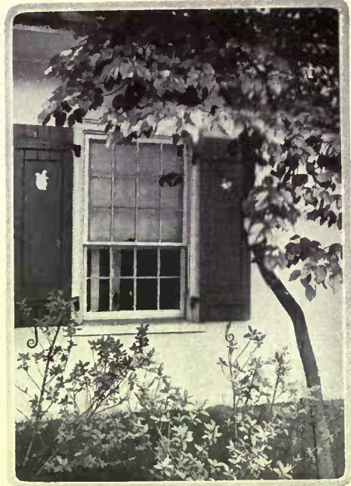
Gillies The interesting feature of this double hung sash window, by Dwight James Baum, is the smaller lower sash
