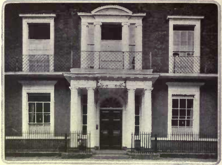
The central window and entrance of the Friends School at York, England, designed by John Carr, both show evidences of Palladian adaptation to their designs
