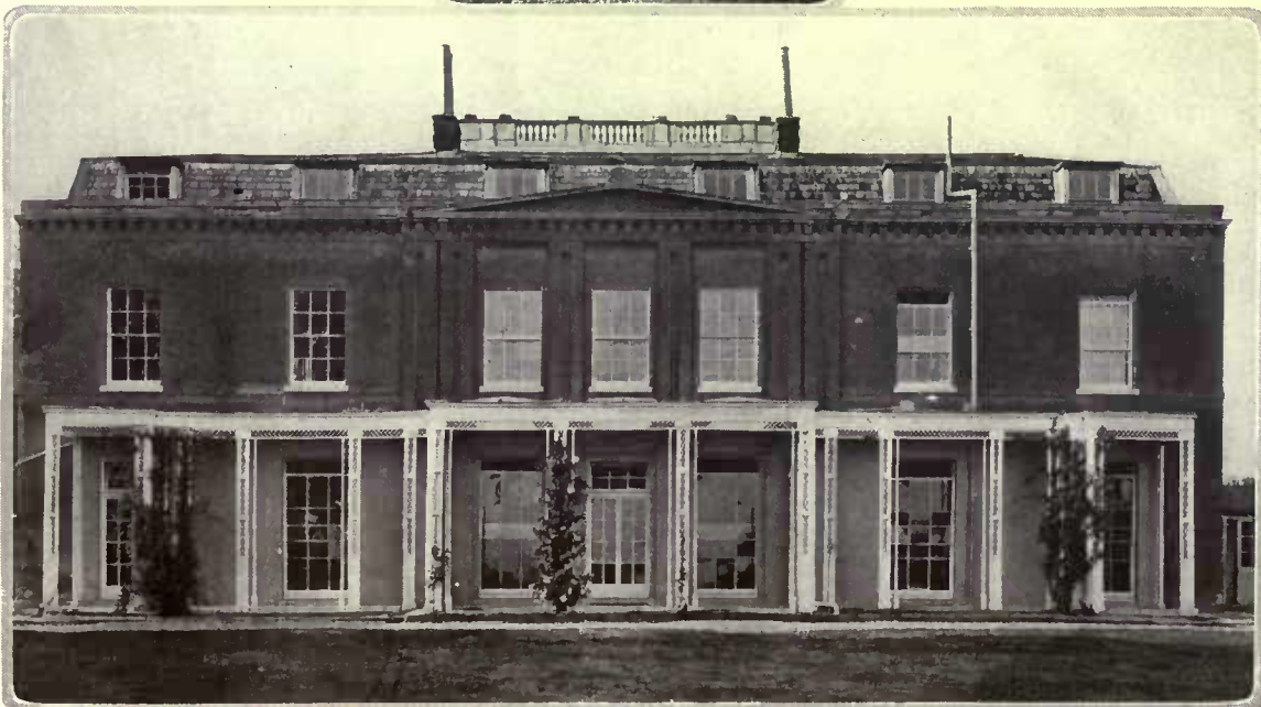
The veranda is a feature of Southern Colonial architecture. As shown here, it is made by recessing the middle unit of the house and supporting the roof on tall columns. Dwight James Baum, architect
