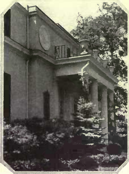
Wrought iron, classical urns, Doric columns and circular medallions have been effectively used in the treatment of the entrance portico. A planting of evergreens gives the house comfortable relation to its site
