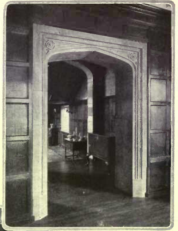
This carved sandstone Tudor door derives its character from the quality of the moldings and their arrangement. Its air of strength is due to the juxtaposition of light and shade created by its vigorous members
