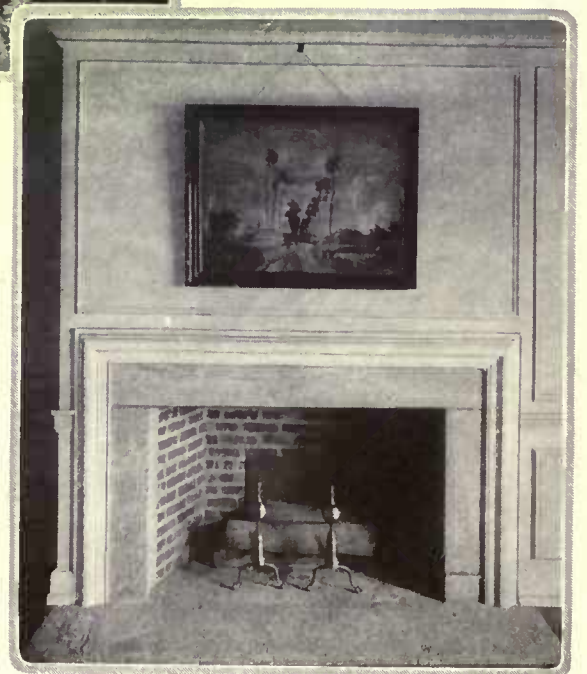
An apartment living room otherwise lacking in architectural interest was transformed by a fireplace faced with brass and studded with nails and surrounded by an architectural frame consisting of two series of stock moldings
