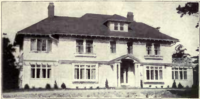
Lunken Windows Installed in Residence Mr. T. Melbye, Wellesley Hills, Mass. Architects: Blackall, Clapp & Whittemore, Boston, Mass.
