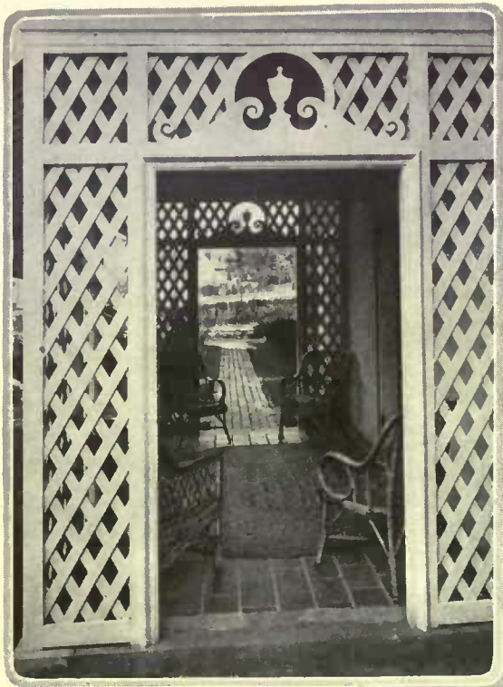
Elegance and interest are given the door of this latticed garden porch by the simple molding, consisting of a fillet around the door, a boldly flowing cyma next to that and a small quarter-round on the outside
