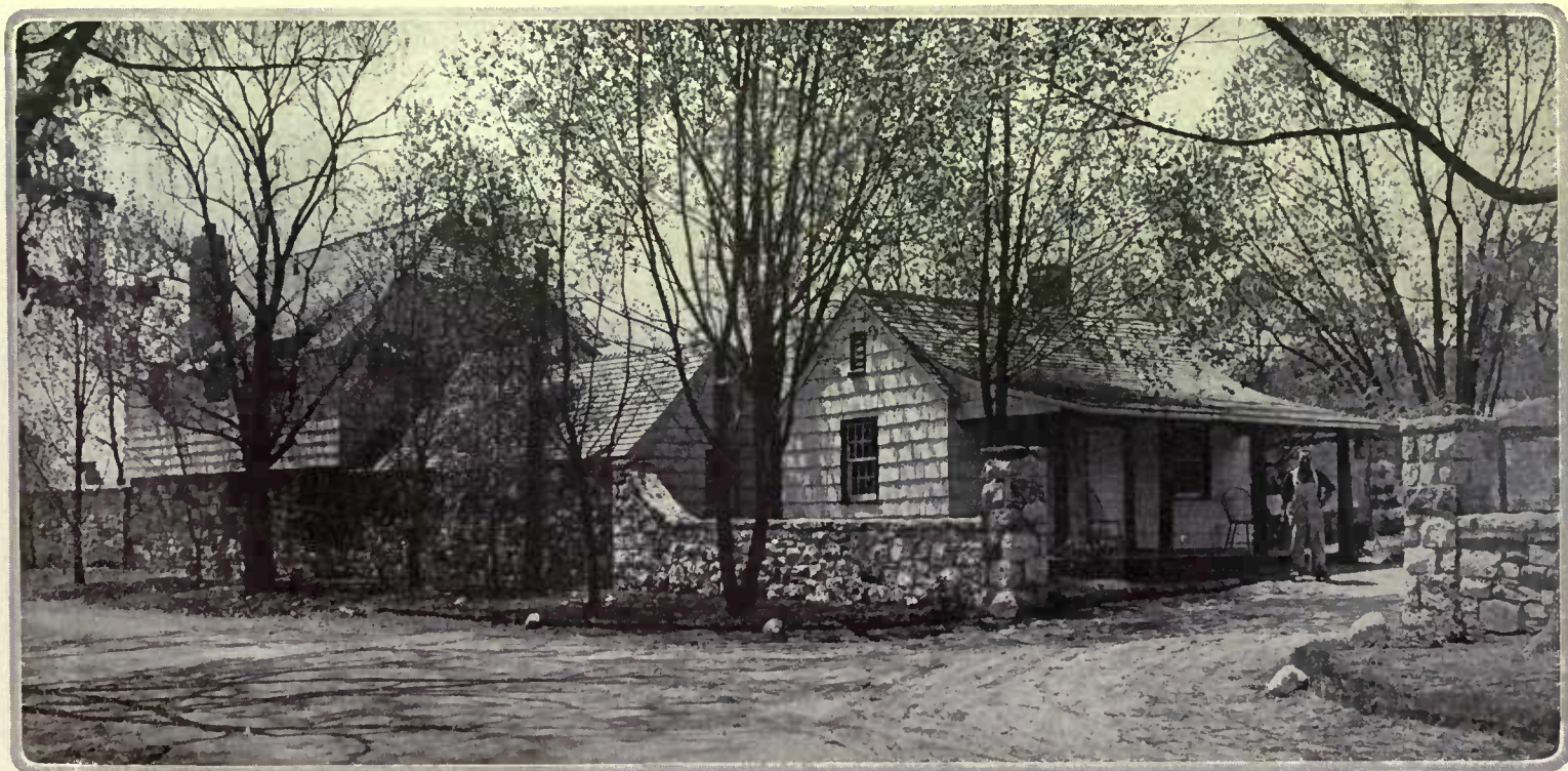
As originally found, this gateside group on the country place of William F. Dominick at Greenwich, Ct., was a barn, shed and milk house. By adding a porch in front and a small wing in the rear for a bath,
