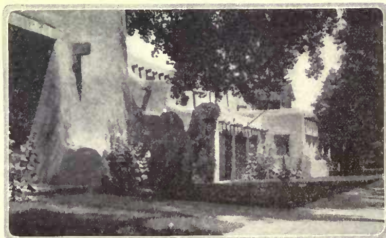
Even so prosaic a structure as this apartment building has been fashioned into a presentable pueblo type with rounded corners, rough surfaces and the exposed roof beams
