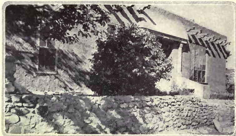
Into this purely modern home have been incorporated some of the pueblo traditional devices, especially the carved roof beams, the rough adobe wall and the flat roof
