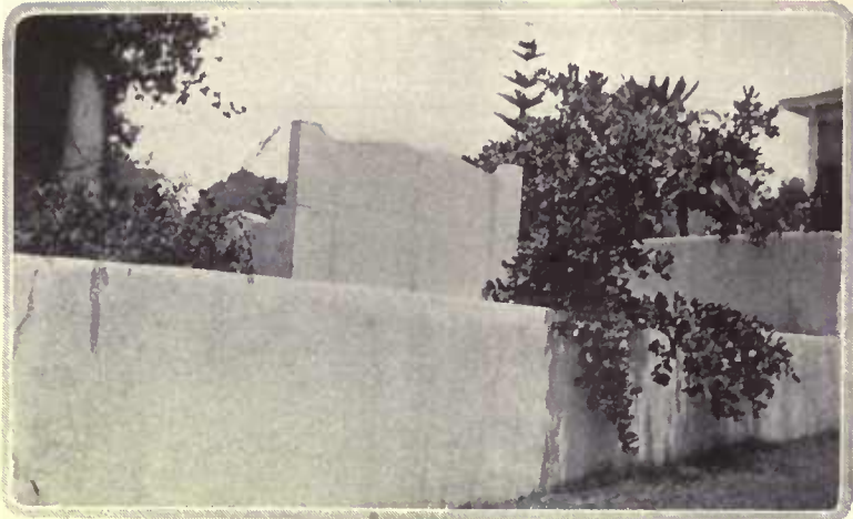
A retaining wall like this calls for the softening effect of fine leaved vines growing up from its foot. Well selected shrubs along its top would add privacy and improve the appearance of the wall
