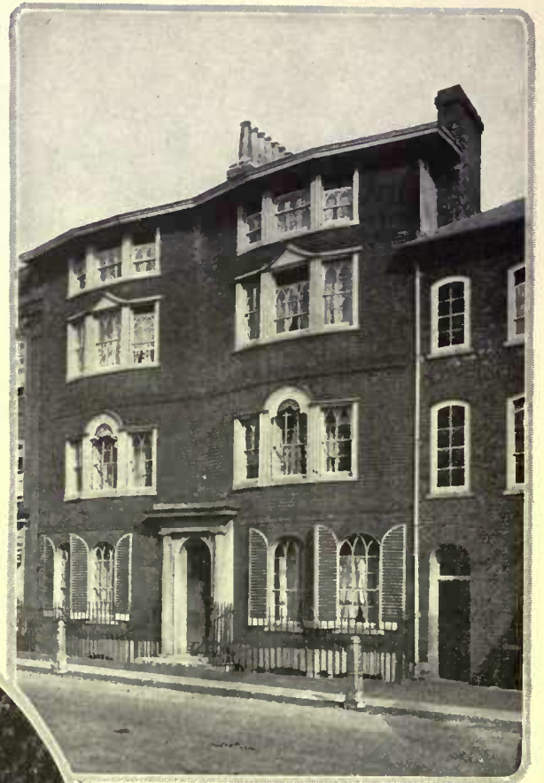
A strictly Palladian interpretation is found on the second floor of this 18th Century house, and, on the third, a Chinese version, with peaked middle lights
