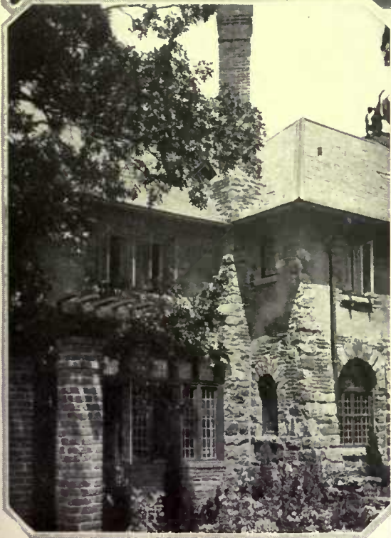
This sunny corner of the garden is flanked by a brick pergola and dominated by the chimney. The interesting character of the masonry and the varied and colorful treatment of the stucco are clearly suggested here
