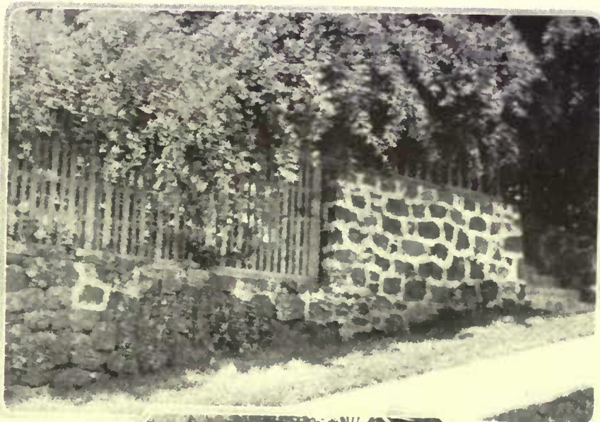
Local sandstone in varying shades, topped by flowering shrubs drooping over a picket fence, forms a retaining and garden wall
