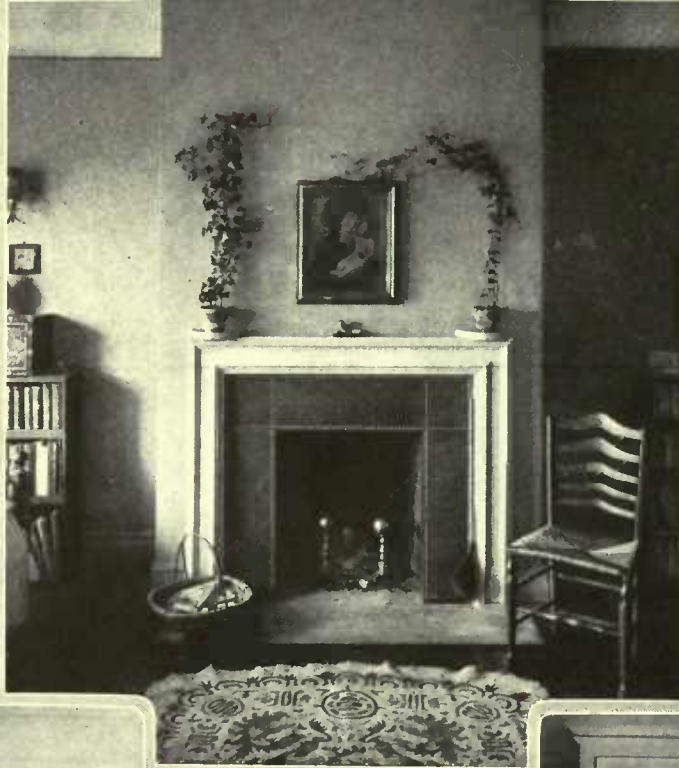
An apartment living room otherwise lacking in architectural interest was transformed by a fireplace faced with brass and studded with nails and surrounded by an architectural frame consisting of two series of stock moldings
