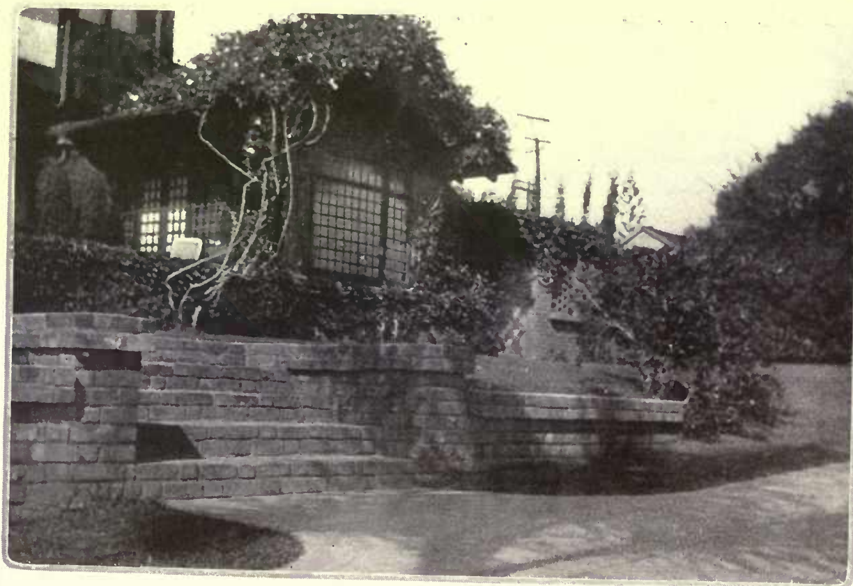
The problem of incorporating steps in a retaining wall is well solved here, where the whole arrangement is simple and unadorned and blends easily into the grassy slope at one side
