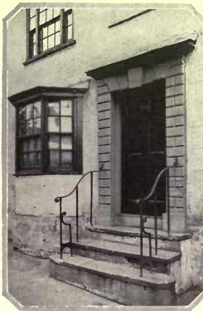
Dignity and style are combined in this doorway of the 18th Century, at Suffolk, England. Pointing gives decorative interest
