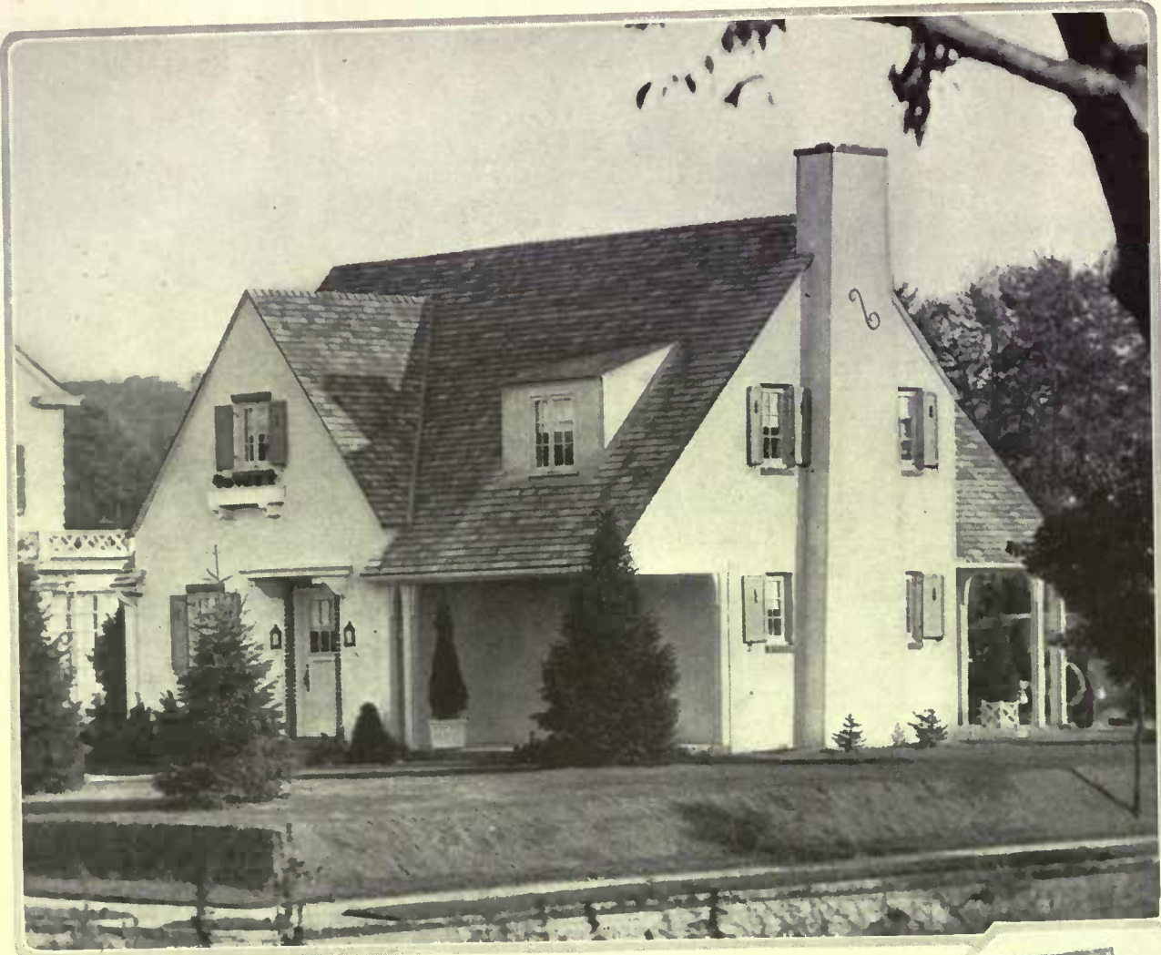
The adaptability of English cottage styles to the American suburban house is proven in the home of G. W. Warhurst, at Philipse Manor, N. Y. It is of cream-colored stucco on hollow tile with red brick sills and borders around the doors
