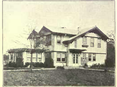
Res.—W. H. Brooks, Sect'y. Standard Fuel & Material Co., Birmingham, Ala. Archt.—Harry B. Wheelock—Birmingham, Ala. Bishopric used on all exteriors or interiors
