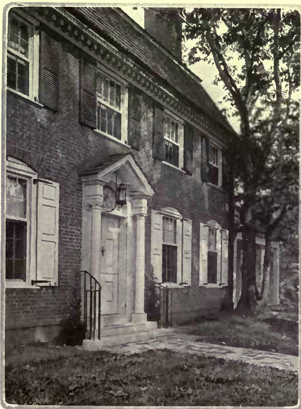
An unusual doorway designed by Donn Barber suggests Greek inspiration, with its Doric pilasters and pointed hood. A frame of plaster has inserts of brick
