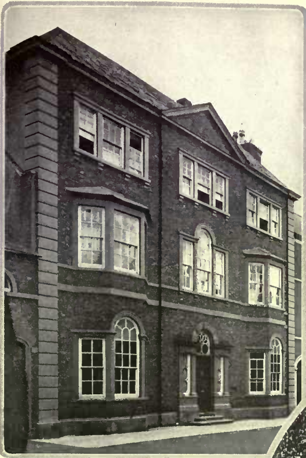
In the doorway, the two flanking bay windows and the window above the door of this house at Pershore, Worcestershire, three different Palladian interpretations are used
