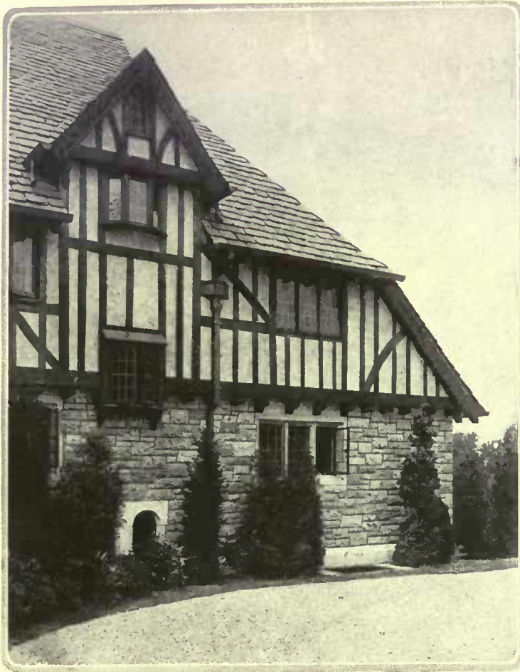
Casement windows are especially appropriate for half-timber houses. Here they are used in a bay, singly, in a row and with stone and timber frames. W. T. Dominick, architect
