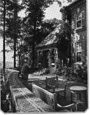
As the place is largely a summer home, the terrace and porch are designed for outdoor living. The brick of the walls is used for the terrace pavement. The heavy slate house roof, purple and green in color, is repeated on the living porch. Copper rain pipes lend their air of permanence. The terrace commands a view of some thirty miles
