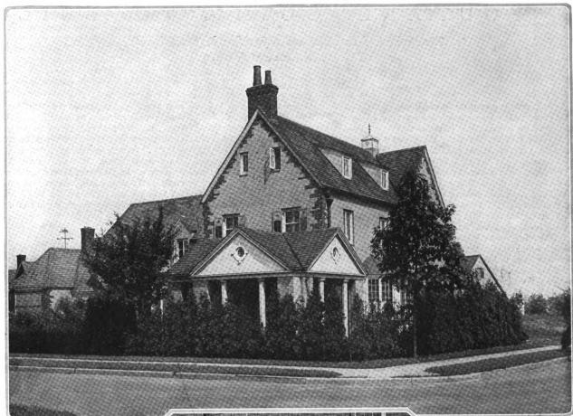
Elements in the home of J. A. Kienle, Forest Hills, L. I., were drawn from smaller English manor houses. Brick walls are painted a warm gray with the corners laid up in natural colored brick projecting slightly from the main face of the wall. The roof is red tile, surmounted by chimney tops and a dove-cote placed at the intersection of the wings
