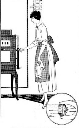
The heat regulator is a simple device placed on the side of gas ranges whereby the housewife can control the temperature for various dishes. Courtesy of American Stove Co.
