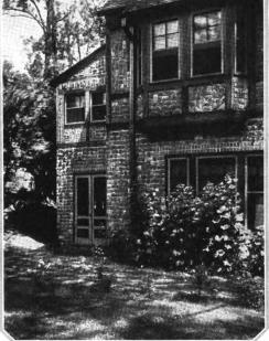
Genuine half-timber, of which this is a good example, consists of the exposed beam frame with brick or cement nogging. The brick can be laid in different designs that give an amusing variation to the wall surface. Instead of the usual casements double sash windows are used
