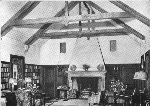
In the home of George H. Doran at Ossining, N. Y., the first floor is simplified by using one large room for living and dining purposes. The woodwork paneling is walnut, above which is rough plaster with the old, hand-adzed ceiling beams exposed
