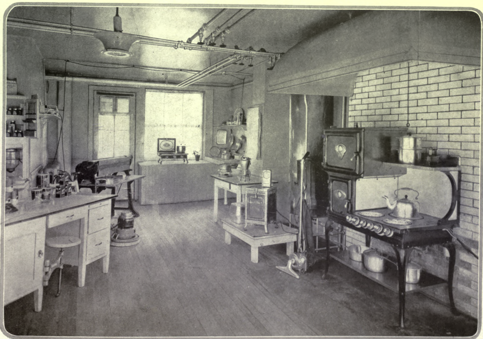
The all-electric kitchen offers the most convincing solution for the problems of domestic management that thousands of housewives now face. It requires intelligent handling, but less actual labor. Its cost of maintenance and its general convenience more than compensate for the initial cost of installation. In this all-electric kitchen the equipment includes a range, fireless cooker, percolator, grill, ovenette, vacuum cleaner and ironing machine. Courtesy of the New York Edison Co.
