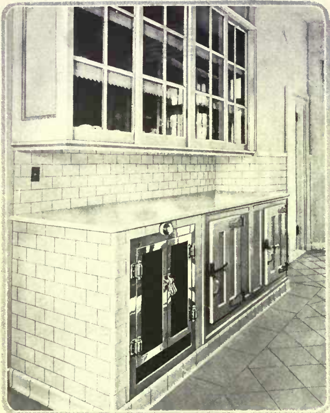
The plate warmer and refrigerator are in non-interfering proximity under the steel shelves of this kitchen dresser. C. P. H. Gilbert, architect. Bramhall, Deane Co.
