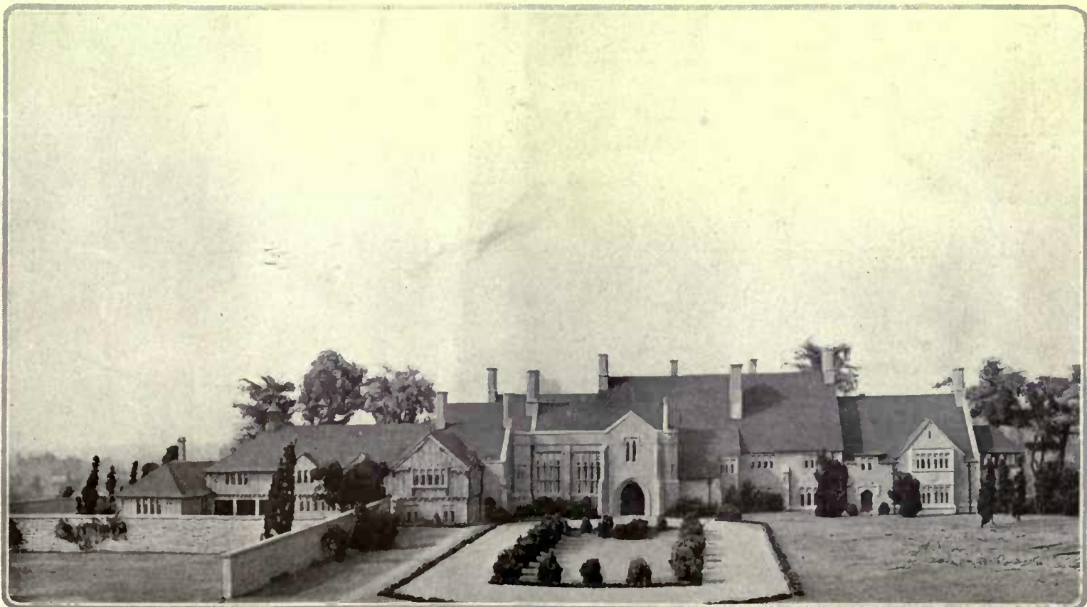
In the more elaborate models, every detail is shown to scale. Nothing is left to conjecture—even leader heads and curtains are put in. The representation is so complete that one can scarcely believe the photograph is not one of a real house. This model of the Philip D. Armour residence is on the scale of 1/8" to 1'. H. T. Lindeberg, architect
