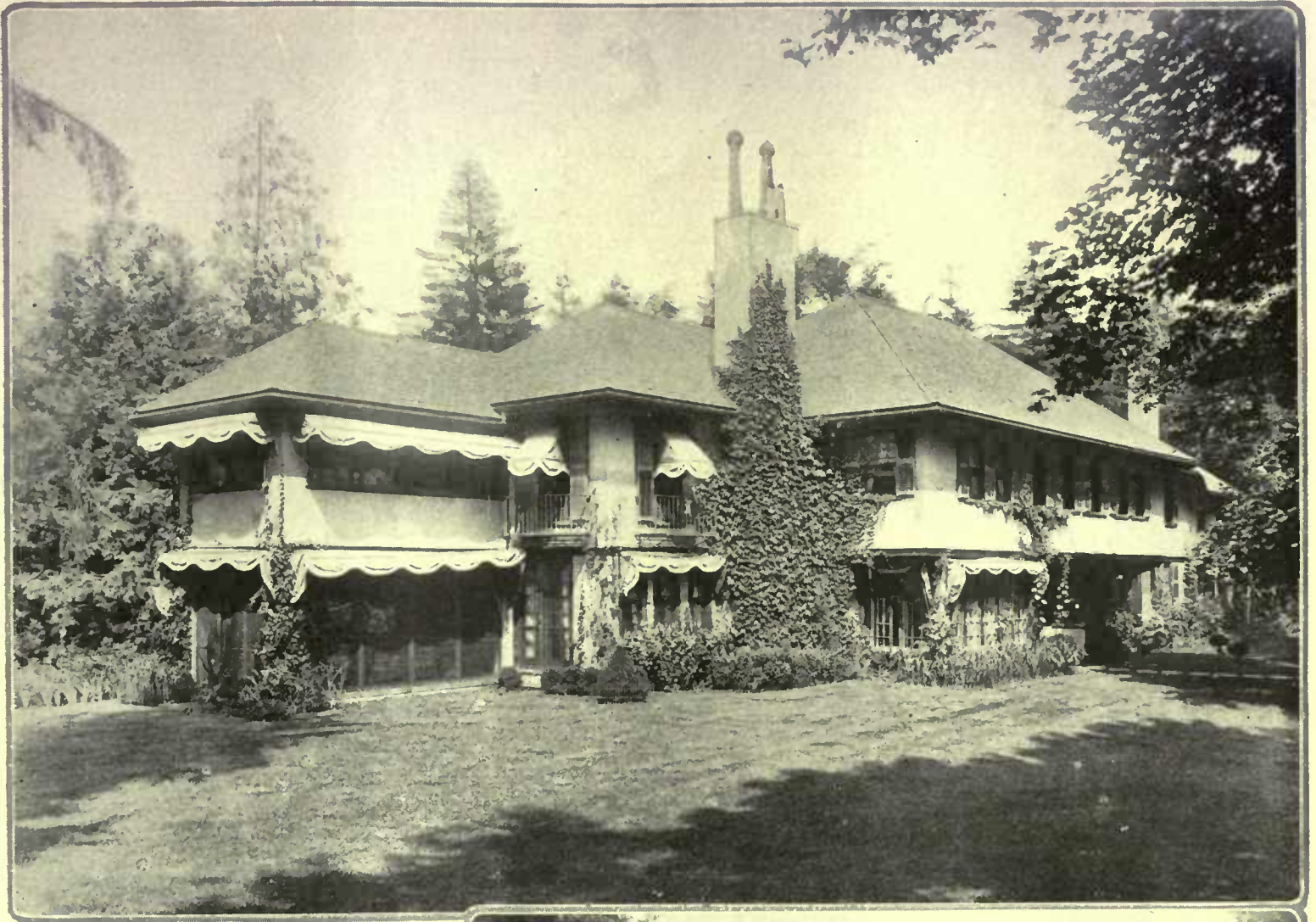
The absence of visible foundation does much to tie the house to the ground and, incidentally, makes easier the arrangement of the plantings. Wide projecting eaves cast relieving shadows. French doors and tall windows admit abundant light and air on the lower floor
