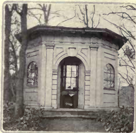
At the end of a long walk on the grounds of Avenue House is a white Georgian gazebo set among trees. It is painted, and its wooden sides are rusticated in imitation of stone
