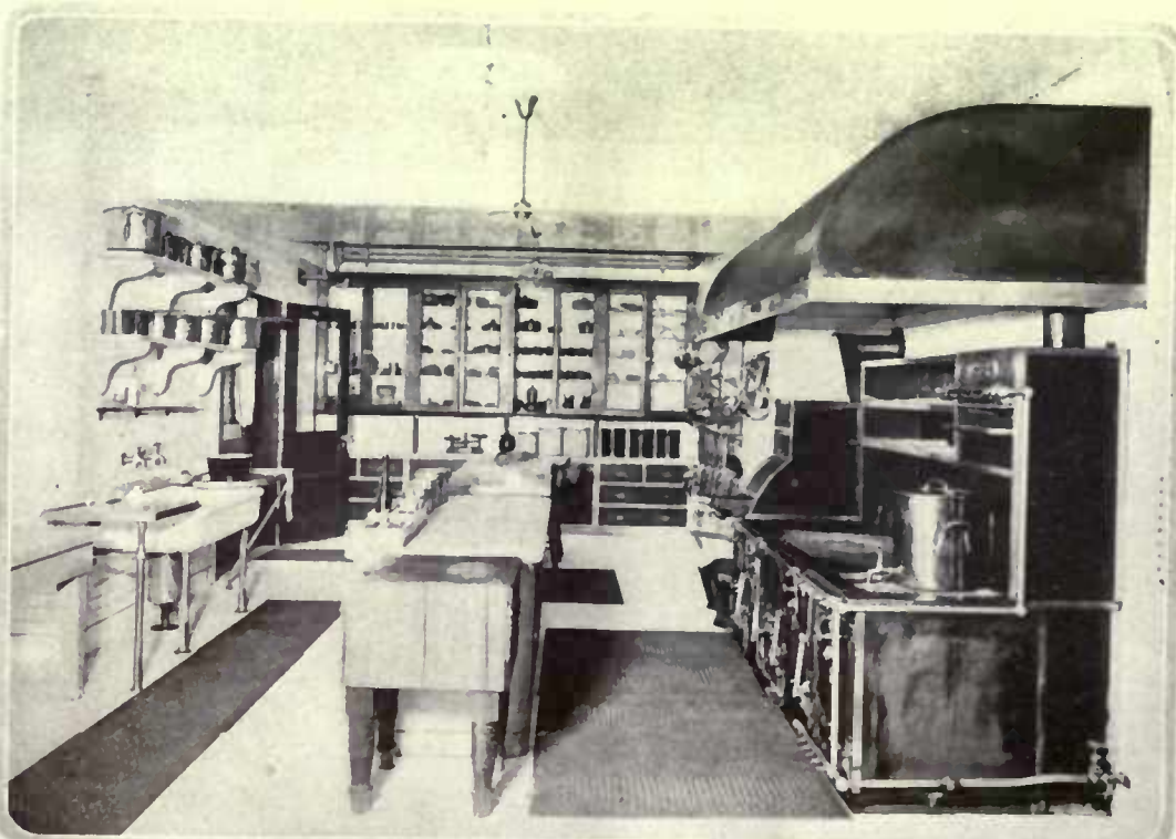
Here is a kitchen that is very much "tabled"—a butcher's block, a pantry table, and composition top tables opposite the range. Note the rubber mats and the interesting shelving. Courtesy of Duparquet, Monet & Huot
