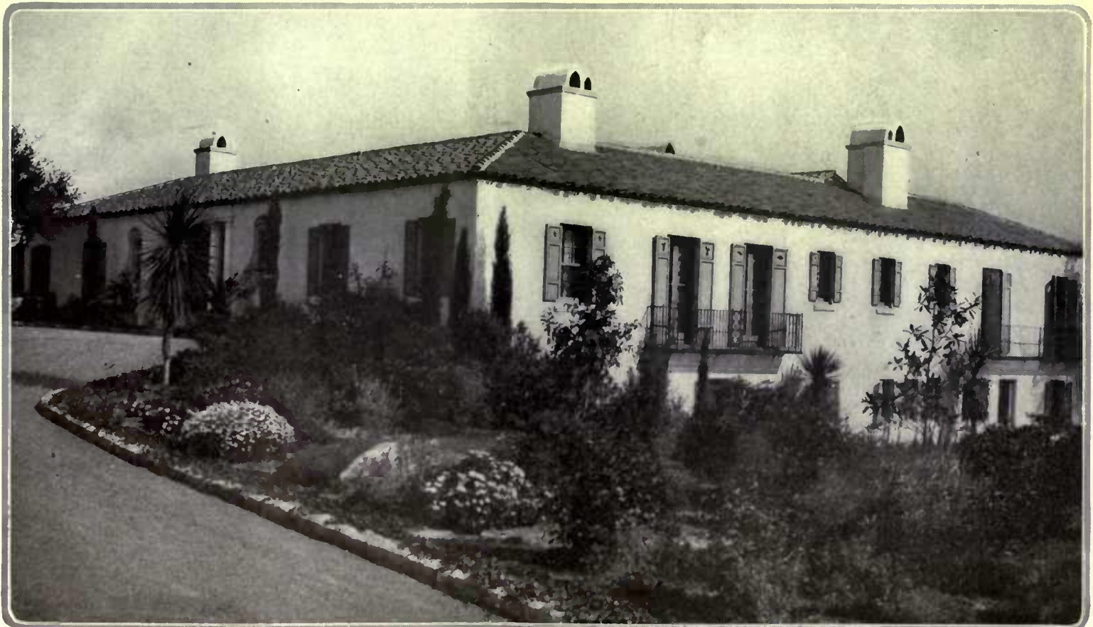
On the entrance side the house appears low, a characteristic which the view on page 19 belies. The roof is of hand-made variegated tile, the woodwork, trimmings and flower pots are blue, and the stucco is white
