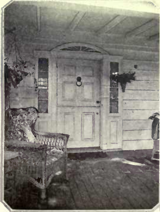
The new Dutch door was especially designed for the house. The shallow fan light is in proportion with the low ceiling of the porch
