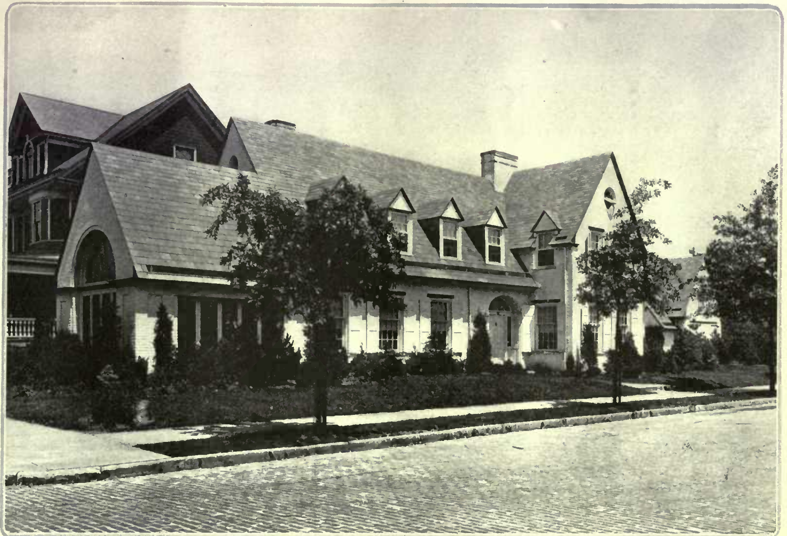
The architect was faced with the problem of a long, narrow lot on a street with houses in close proximity. Consequently a long, narrow house was designed. The general style is Colonial, executed in brick painted white and with a slate roof. Interest is given the design by the number of gables, the small paves and the range of dormer windows
