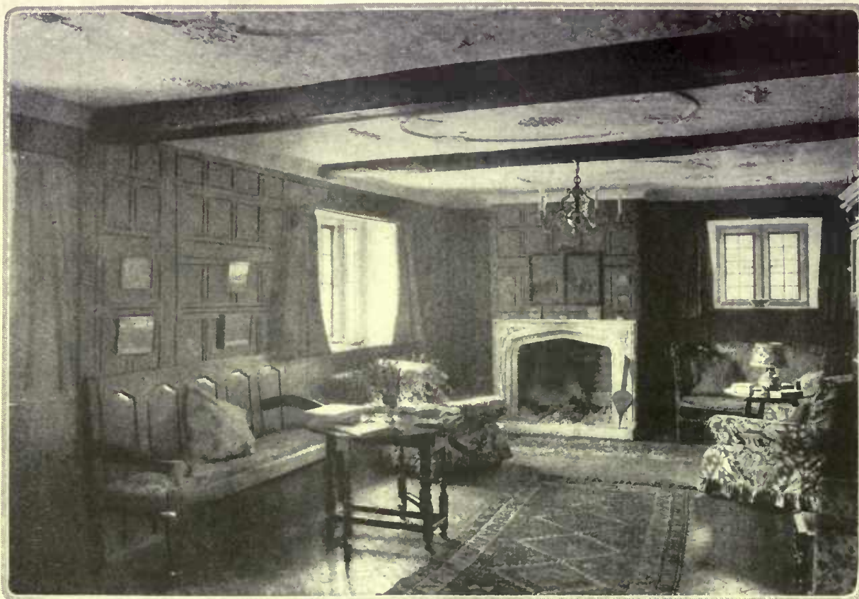
Decorative designs in parge may be used appropriately on ceiling surfaces in conjunction with exposed beams, oak panelling or other treatment of the room which harmonizes with the sturdy character of the material
