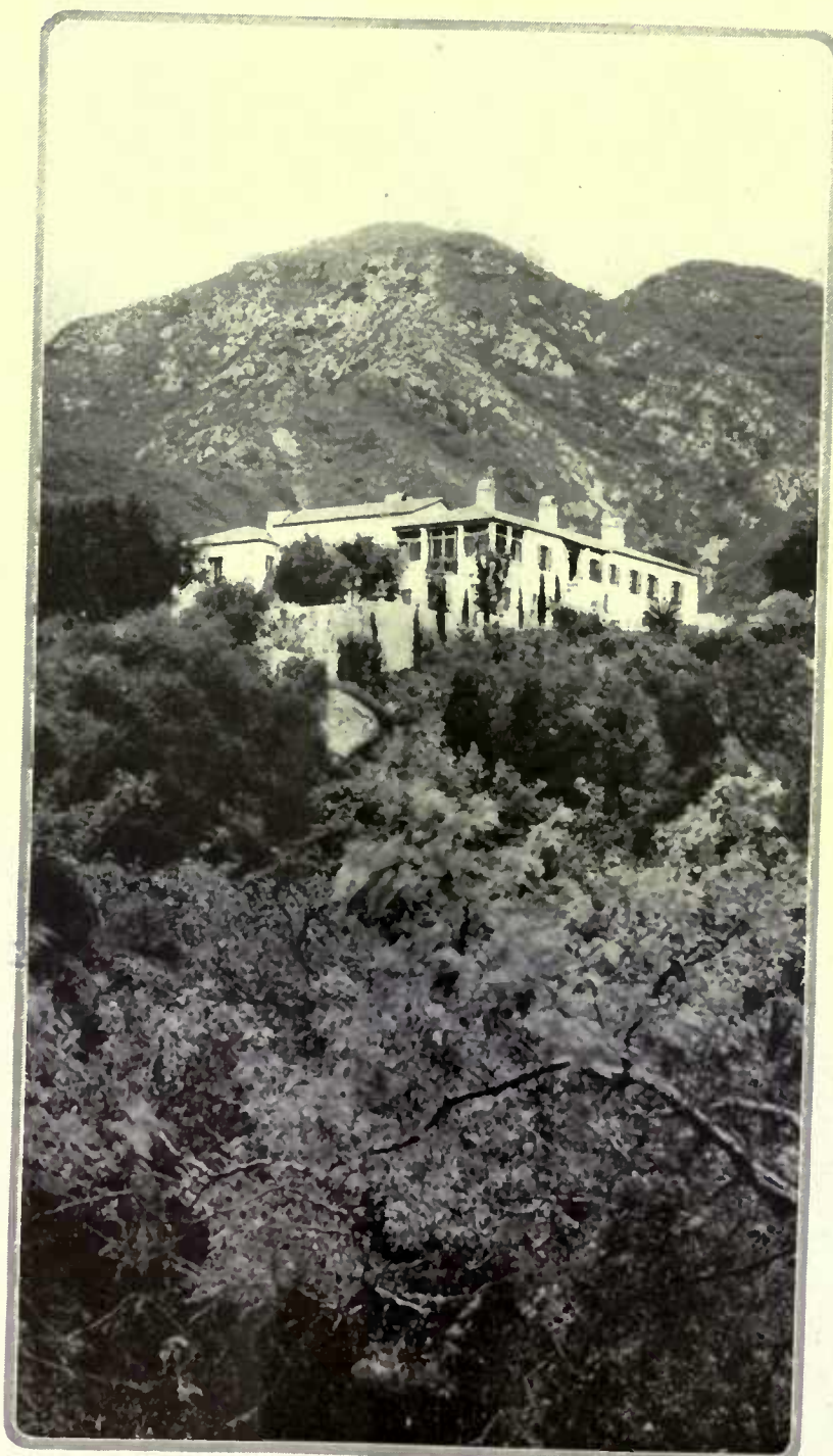
Nothing could be more Italian than the way the house sets on the hillside above the canyon, with the sparsely wooded mountains behind it. The mass of the house shows the variety of levels so often seen in the architecture on Italian hillsides. Guy Lowell, architect
