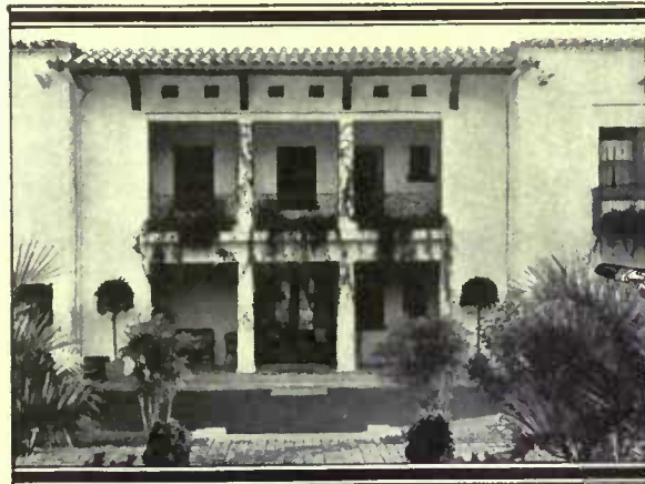
Residence of G. W. Wattles, Garden Front, Hollywood, Calif. Myron Hunt & Elmer Grey, Architects
