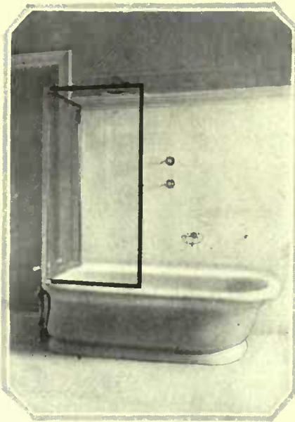
A bathroom in the residence of Mr. Felix Warburg shows an ideal shower arrangement for the shower
