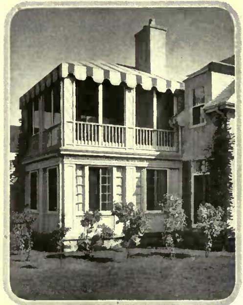
The porch can be roofed in tin cut to a scallop edge and painted to simulate awning
