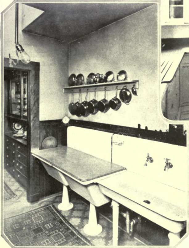
A pot shelf is a simple arrangement — the supporting board has hooks on which to hang the pots, the shelf takes the covers. Knives are stuck in a wooden groove back of the sink
