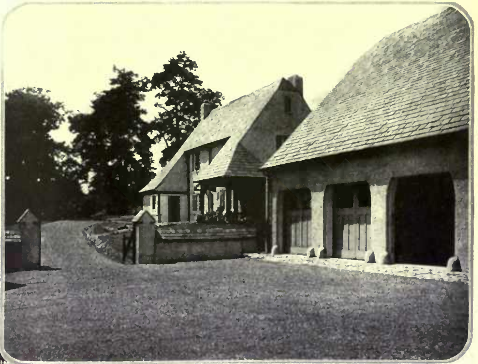
The gardener's cottage is a simple stucco house with steep roofs extended down to cover the porch and kitchen wings. An interesting feature is the way the stucco comes to the edge of the slate on the gable roofs without any woodwork
