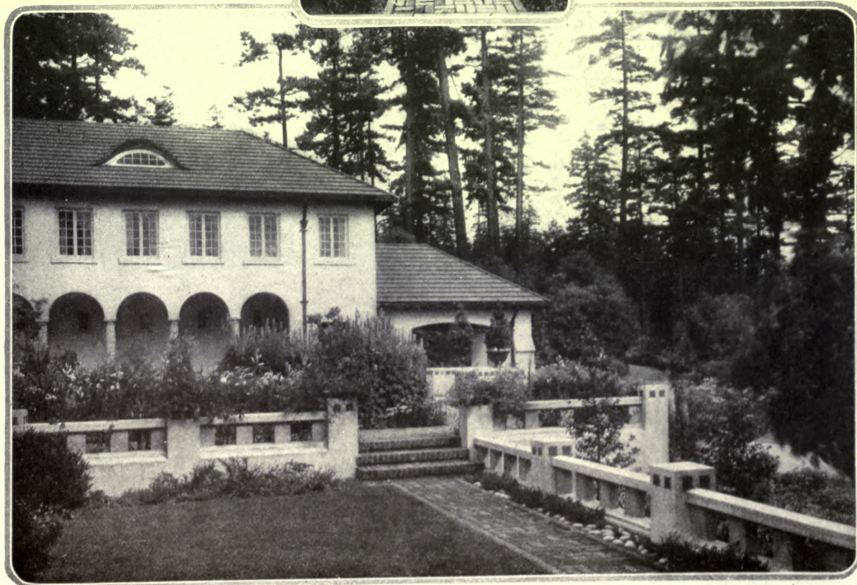
The various garden levels are marked by cement balustrades so that each level has its own personality and distinction
