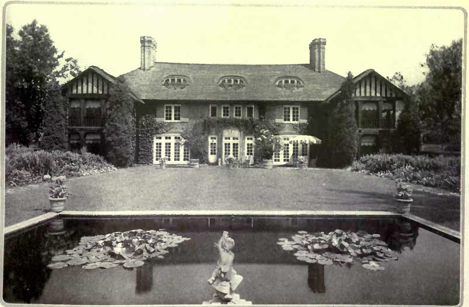
Because it commands the south view looking out over the garden, this façade of the home of Laurance H. Armour, Esq., at Lake Forest, Ill., shown below, has large windows in the living room, hall and dining room. The half-timber extensions have sleeping porches above
