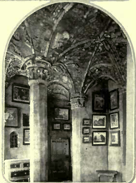
A curious treatment, not advisable in every instance however, is a vaulted ceiling with polychrome tile decorations embedded in the cement. This is from the residence of H. C. Mercer, Doylestown, Pa.
