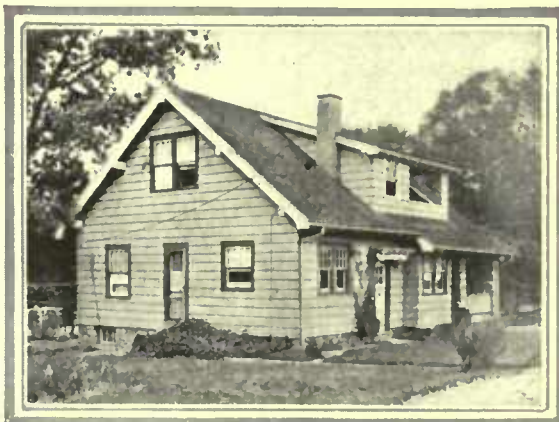
An Attractive Low Cost House of the Semi-Bungalow Type. Mr. Phillip Reanyk, Architect
