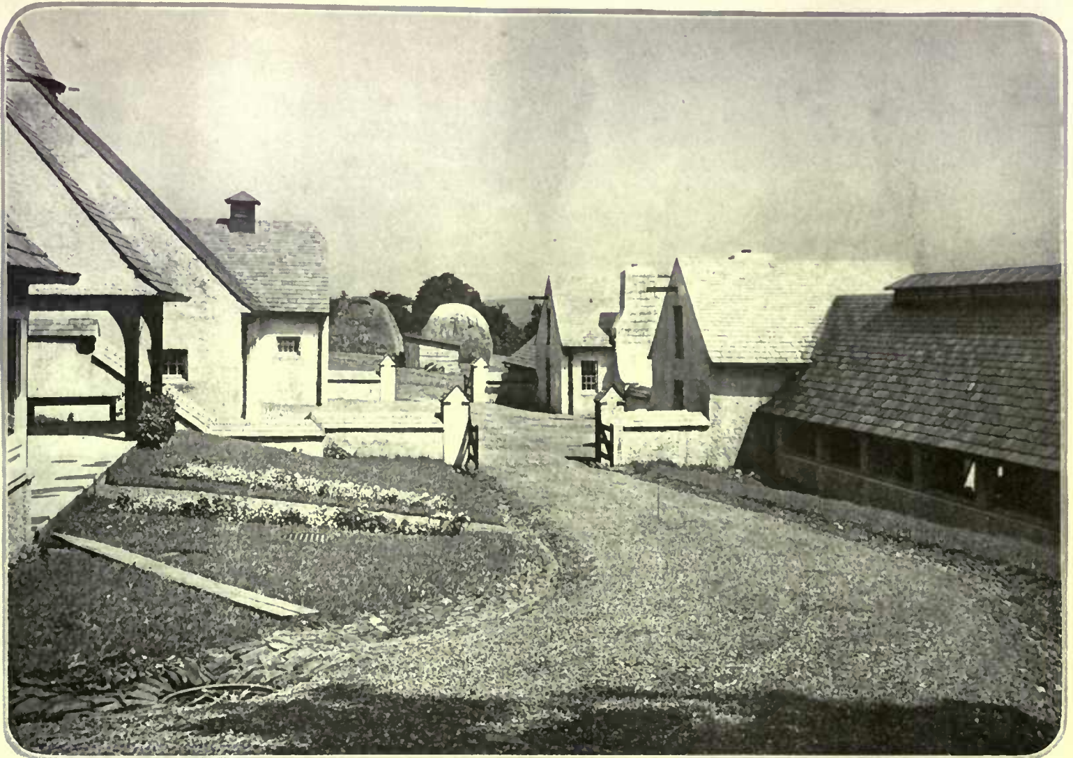
Beginning at the right you see the sheep fold and beyond that the piggery and the barns, with the hay ricks in the fields beyond. On this side of the gate is the gardener's cottage and on the other side the barns and wagon houses. The walks are warm, cream colored stucco. Roofs are gray, red and purple slate
