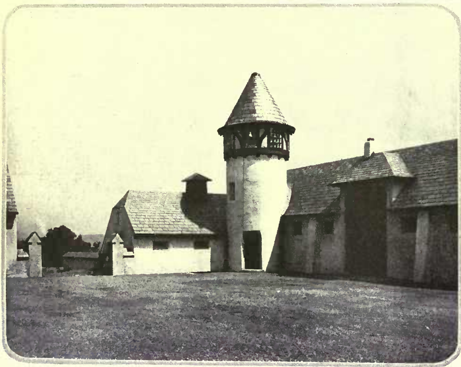
There is a touch of half-timber in the upper story of the tower. A decorative detail, this tower serves for dove cote and belfry; here hangs the bell that calls the hands to work. The buttressed walls are an interesting feature of this view
