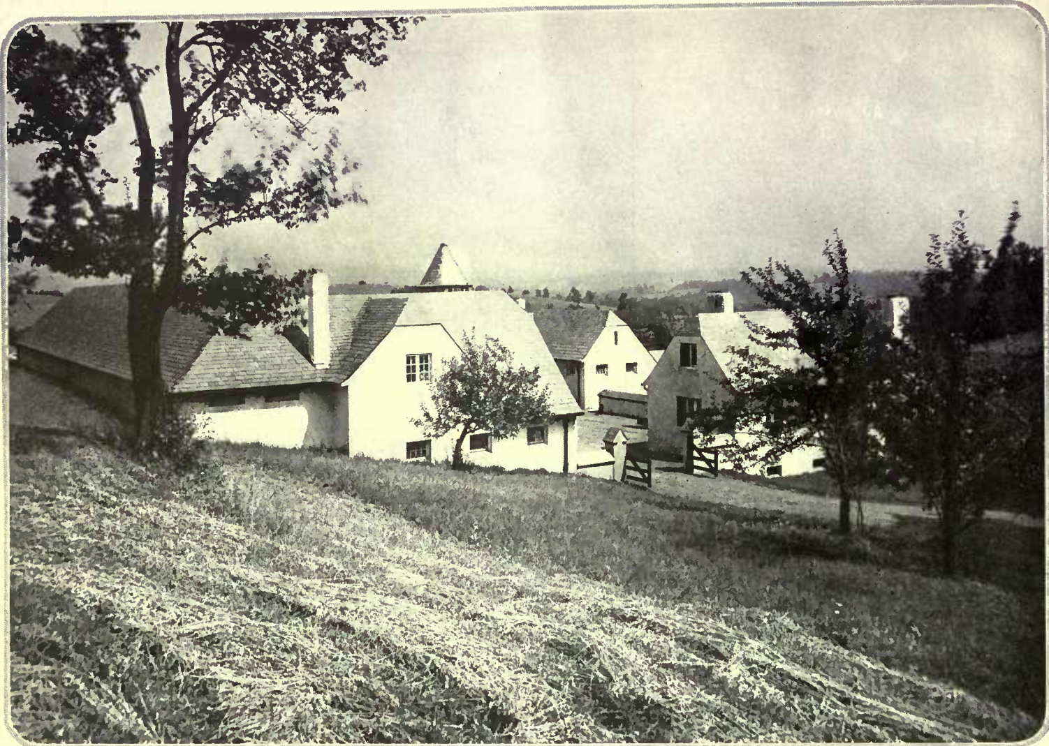
The buildings are on two levels of ground, on the shoulder of a gently sloping hill. They are grouped around a large yard with low fences and gates at each end. Architecturally, the buildings are a combination of French and English, and reminiscent of the picturesque old-world farms one finds in Normandy
