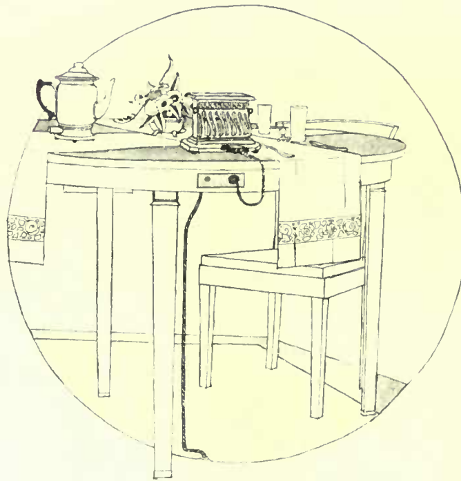
Instead of the unsightly wire dangling from a fixture, the central floor plug should be used in the dining room. The wire can be run through or between the rugs and attached to a box let into the apron of the dining table. It is a simple matter then to plug in the toaster or other electrical table devices
