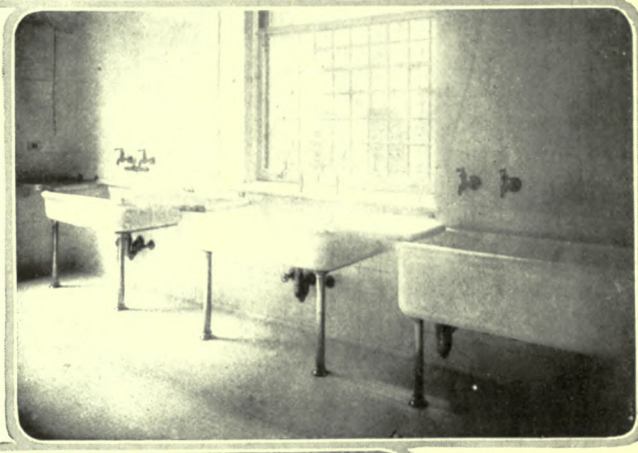
Sinks should be grouped according to their uses and placed in a good light. Open plumbing, compression faucets and roll rim sinks of English porcelain are found in the Frick group, which is shown above. Courtesy of Meyer & Sniffen
