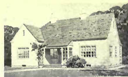
This five-room English cottage is built for comfort and follows the best traditions of English construction.
