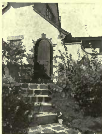
Hollow tile for steps and path— a view from the June issue
