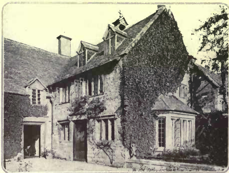
One of the old parts of the building was the chapel with its glass dormers, balanced rows of leaded casements and flagged courtyard
