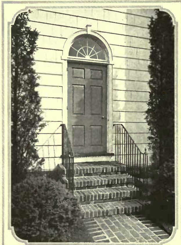
Simple elements, naturally combined, make up good architecture—the shingled wall, the ruddy brick, the unyielding wrought iron, the arch and its keystone, the fan light, the paneling of a door. Aymar Embury II and Lewis E. Welsh were the architects of this example
