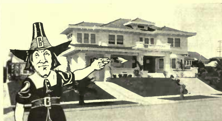
Residence of W. W. Orcutt, 405 So. Mariposa St., Los Angeles, Calif. H. F. Dierker, Architect
