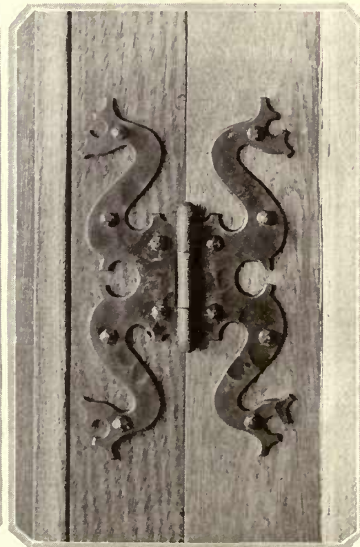
In the same house is found this hinge, an unusual modification of an old design done in wrought iron
