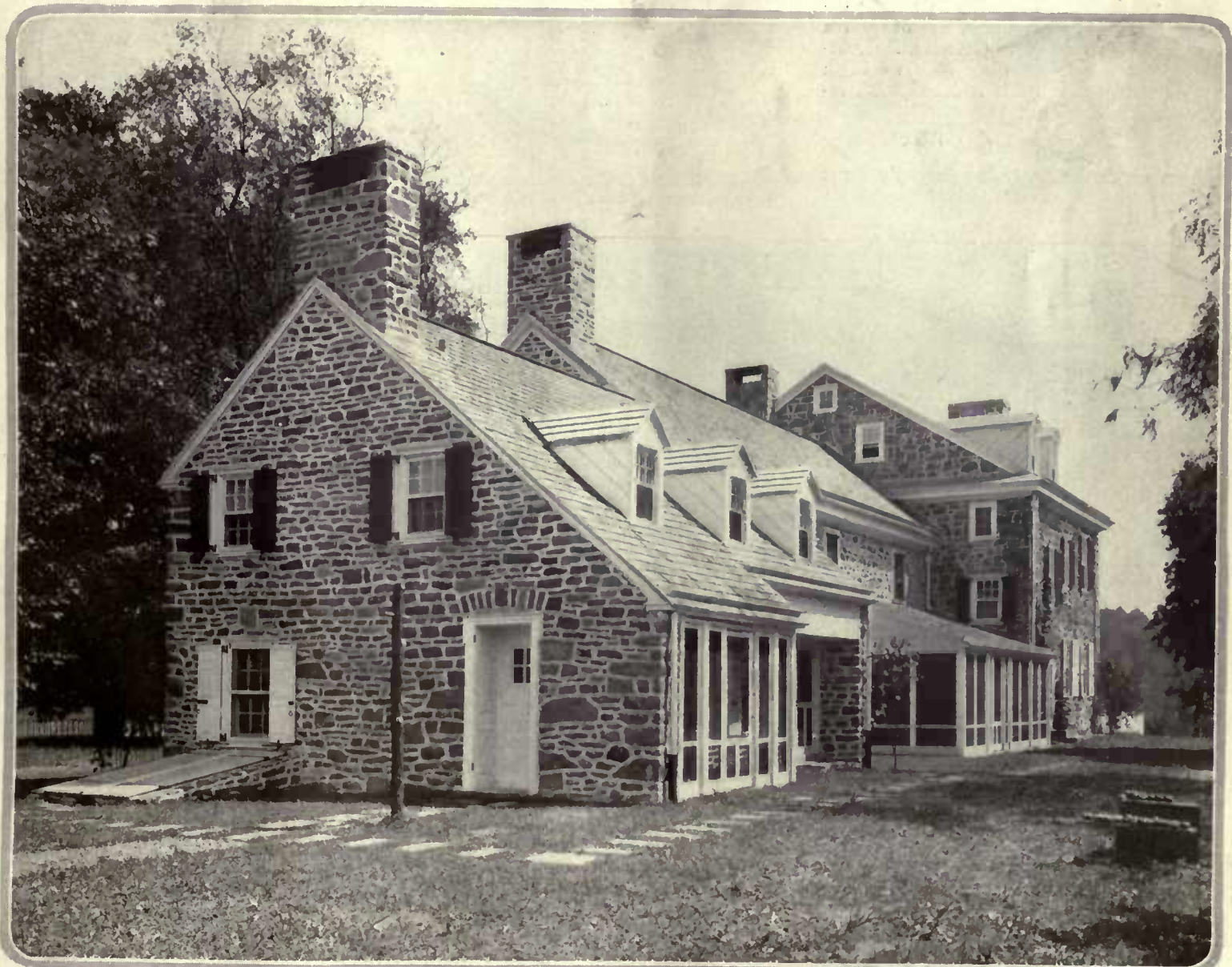
The spirit of the old house is successfully reproduced in this kitchen wing where field stone laid in wide bond, white painted trim, simple dormers and deep doorways are the elements successfully used
