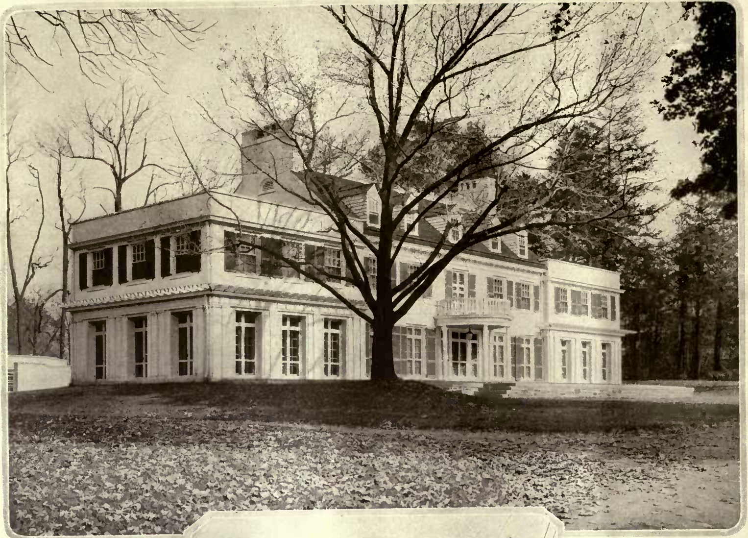
To a large house of Colonial design are added Georgian wings. The regular fenestration adds to the dignity of the architectural ensemble
