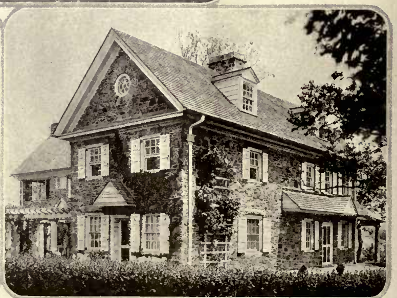
"Wynnestay", Philadelphia, has the Pennsylvania Colonial characteristics—field stone walls, wide eaves, pent roofs over doors
