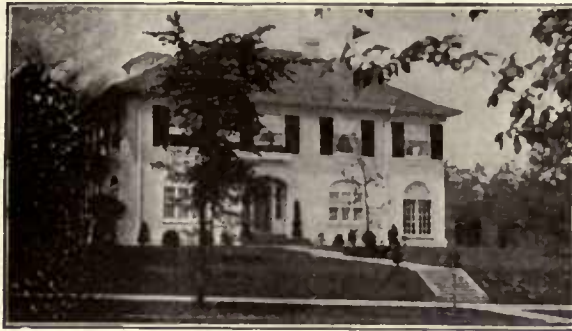
Kelsey Health Heated residence of W. J. Moffat, Edgchill Road, New Haven, Conn. Brown & VonBeren, Architects.
