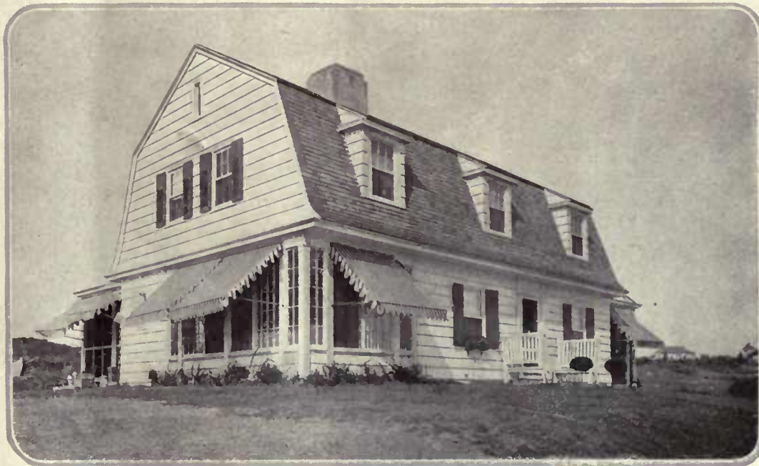
The gambrel roof type is a favorite Colonial style because it is pleasing to the eye and affords the greatest possible space for the outlay. Aymar Embury II, architect
