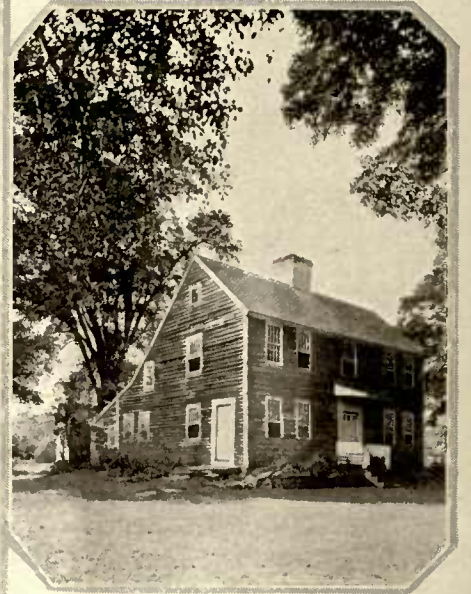
A Connecticut type of Colonial is found in this house on the Green at Branford, Ct. The long sweeping roof is a marking characteristic
