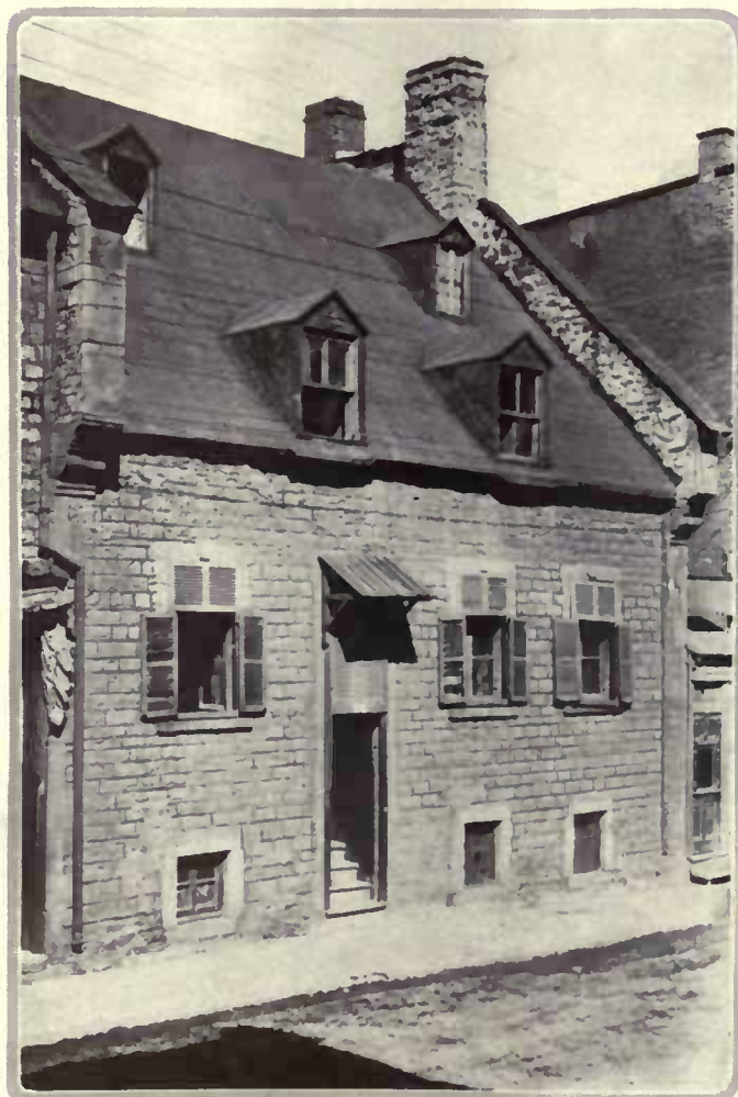
An old town house in Montreal showing the high parapets and double chimneys. Courtesy McGill University
