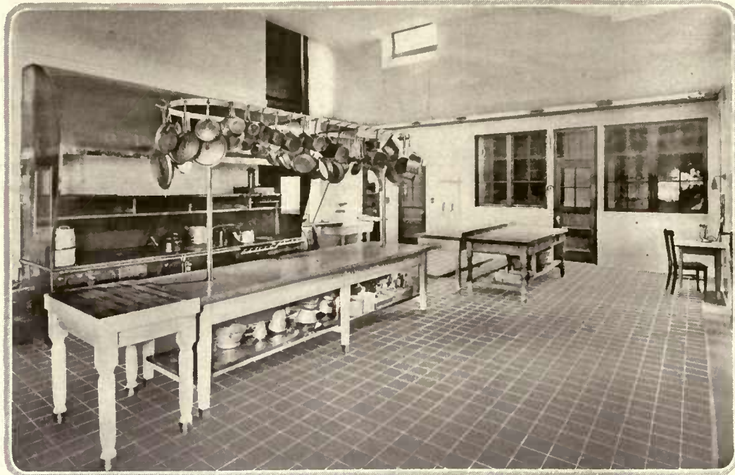
The kitchen in the New York residence of Otto H. Kahn, Esq., is equipped with the most modern facilities. The walls are tile with cove corners and the floor is of cork composition
