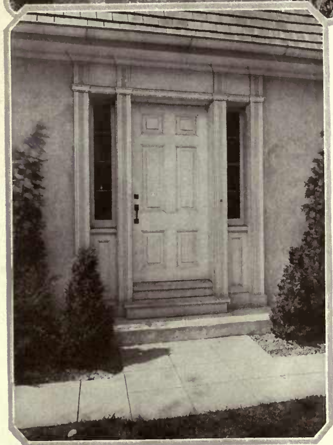
A doorway arrangement, common to certain types of Colonial houses, has been reproduced here. It is a six panel door with side lights set in a frame of dignified moldings. The overhang gives protection to this entrance
