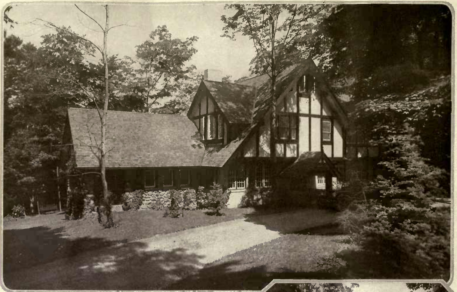
In the construction of the William Wiese residence at Scarsdale, N. Y., stone, tile, half timber and stucco are successfully combined. Roof lines come close to the ground, thereby producing a broad, low and hospitable front
