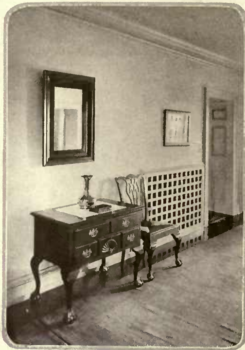
This radiator grille is made of plaited iron strips, behind which the radiator is set
