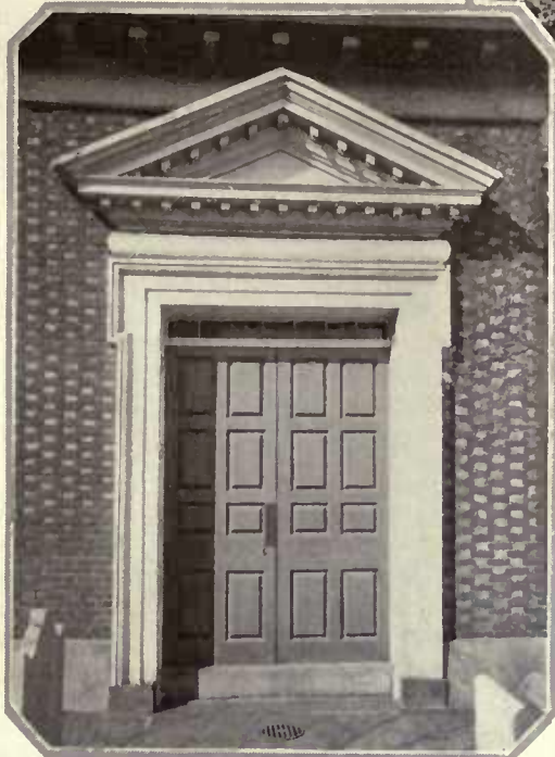
The door of Gloria Dei Church in Philadelphia presents a study in the regular paneling of the early 18th Century. A stately style in a stately frame
