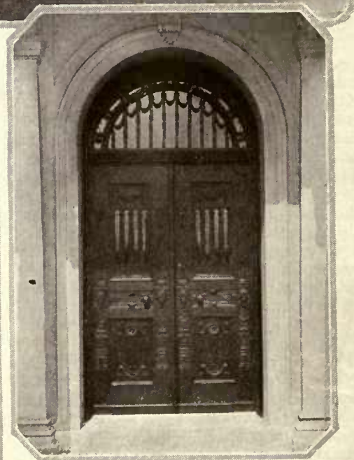
The front door is constructed of teak wood, hand carved and finished with bronze grilles
