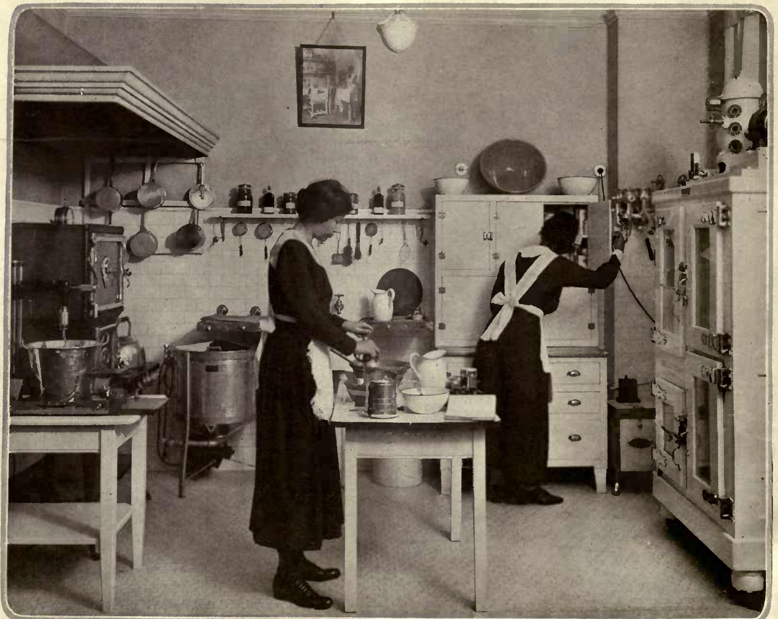
Almost everything runs by electricity in this elaborate kitchenette—electric stove, dishwasher, bread mixer, and ice machine. There are no back-breaking cupboards, but the utensils are hung up at a reachable height. Courtesy of the Edison Co.
