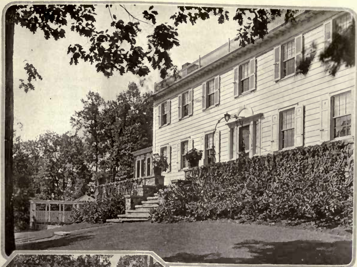
Because of the steepness of the ground, the site is cut into several levels. The house is placed on a broad terrace paved with flags and with blue flowering plants in spaces here and there. The style is taken from the simplest New England prototypes. A railing crowns the cornice
