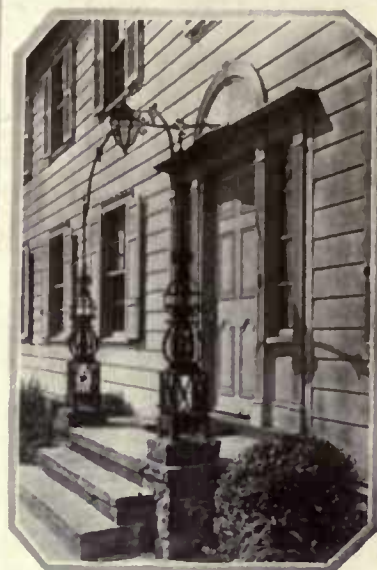
The doorway, one of the features of the front, is flanked with an arch bearing a lamp made from a pair of antique iron newels taken from an old house in New York. The exterior—clapboard walls and brick chimneys—is painted white, and the iron porch and entrance archway bottle green
