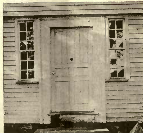
At Milford, Conn., is found a seven-panel narrow type of Colonial door of late 17th Century design
