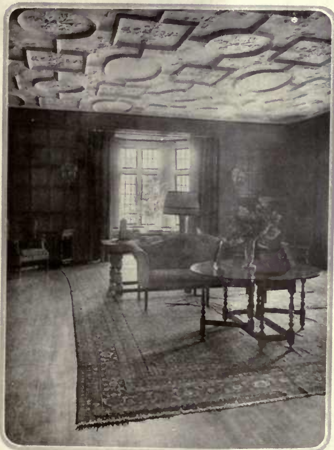
A reproduction of English Renaissance molded plaster ceiling with geometrical ribbing and low relief panels. Wilson Eyre & McIlvaine, architects
