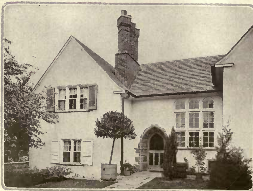
A stack rising out of the valley of the eaves is an interesting architectural expression. Its form is in keeping with the simplicity of the facade. Edmund R. Gilchrist was the architect
