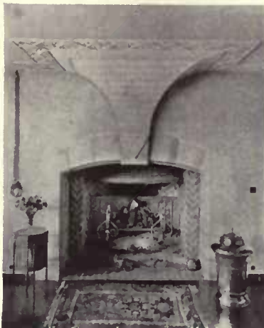
Ornamental plaster walls are considered in February
