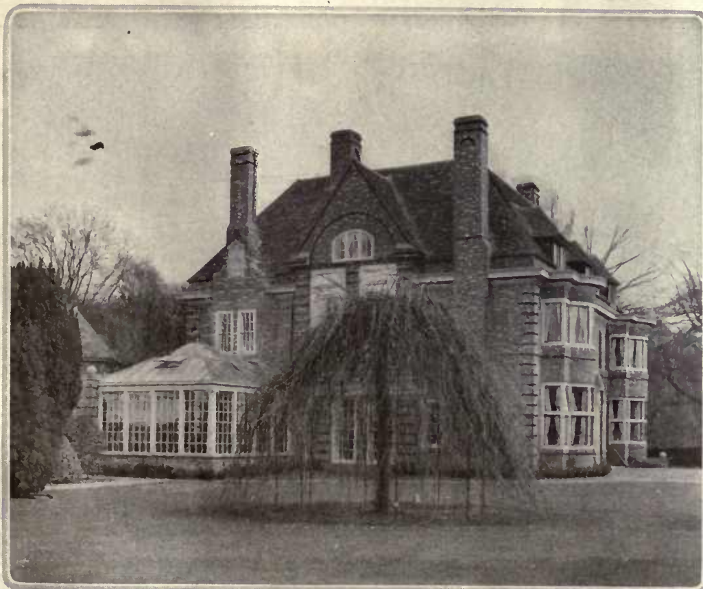
In formal types of architecture a balanced disposition of the chimneys lends great dignity to a residence. In this English country house, designed by A. Winter Rose, architect, one of the garden side chimneys has a vertical sundial
