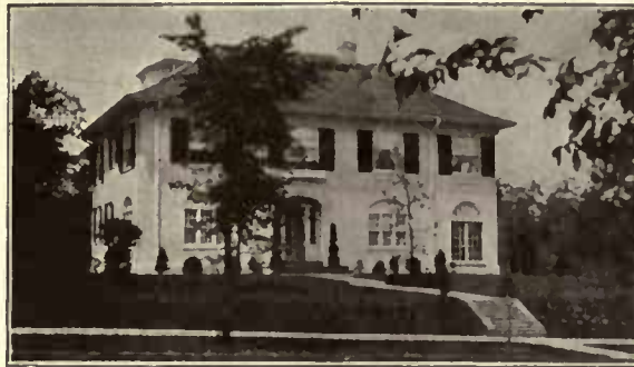
Kelsey Health Heated residence of W. J. Moffat, Edgohill Road, New Haven, Conn. Brown & Von Beren, Architects.
