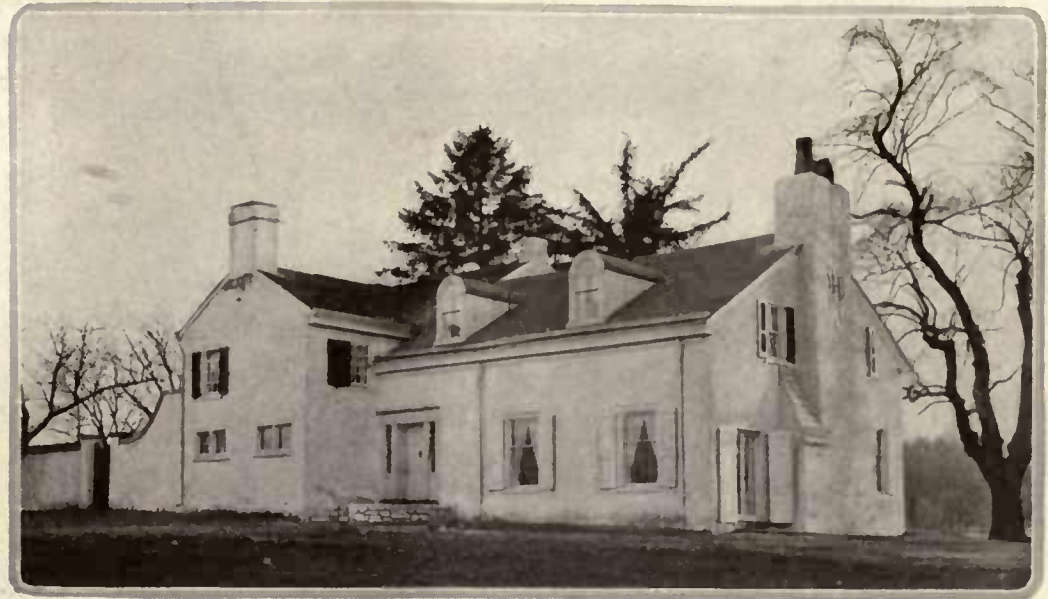
The buttressed chimney gives an air of solidity to the wall. In this home of the Pickering Hunt, Phoenixville, Pa., part of the buttress is shingled and the chimney face broken with a wrought iron monogram. Mellor & Meigs, architects
