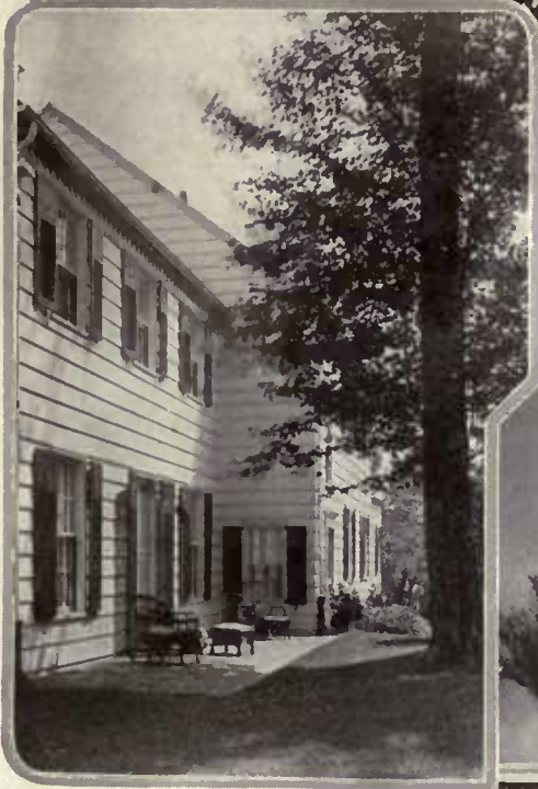
Off the living room entrance is given to a paved terrace through a French door. From this is commanded a view across the hills and woods. The old moon cut shutters and black hardware are in keeping with farmhouse architecture
