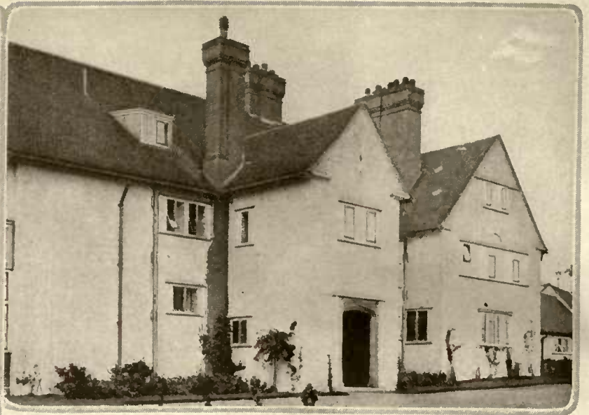
An unusual location for the chimney is in the angle of the wall, where, as here, it can crop out against the contrasting stucco. From a house in England designed by Geoffry Luca, architect
