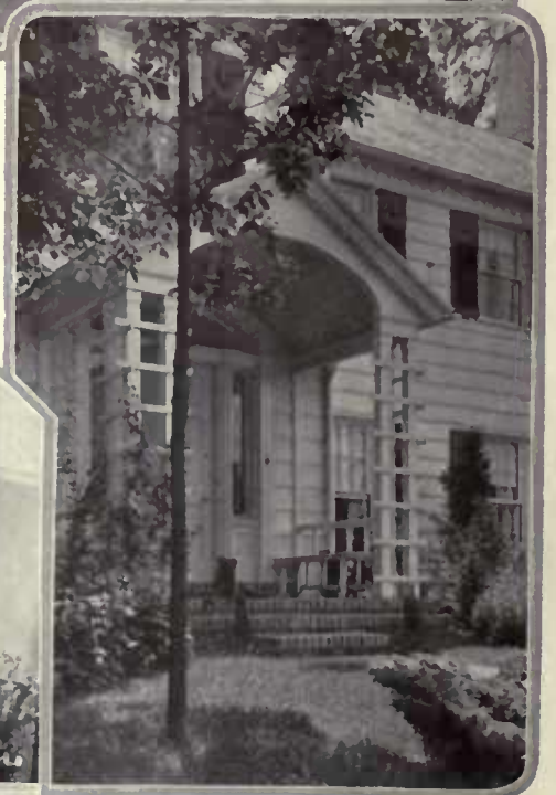
The main entrance follows the Colonial classic proportions, with post and lattice work in place of the usual stock columns. The door has an old Colonial fan light at top and two leaded lights on the side. Bricks form the floor
