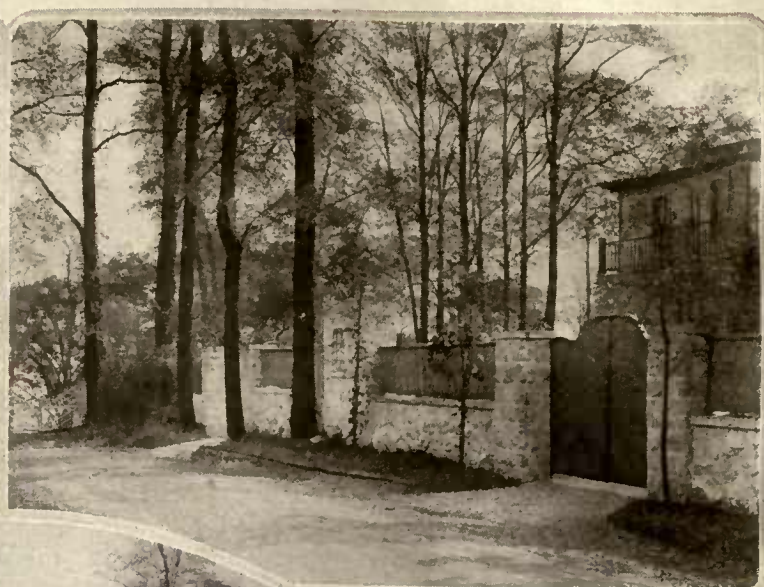
Stone walls should, by rights, keep people out, but when beyond green railings and gates appear gay green balconies it can't be done
