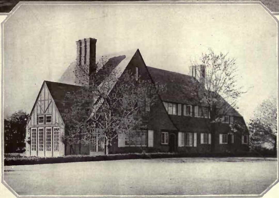
The house is modern English adapted to American requirements. Built of rough red brick laid in English bond; roof variegated rough slate. This view shows driveway entrance
