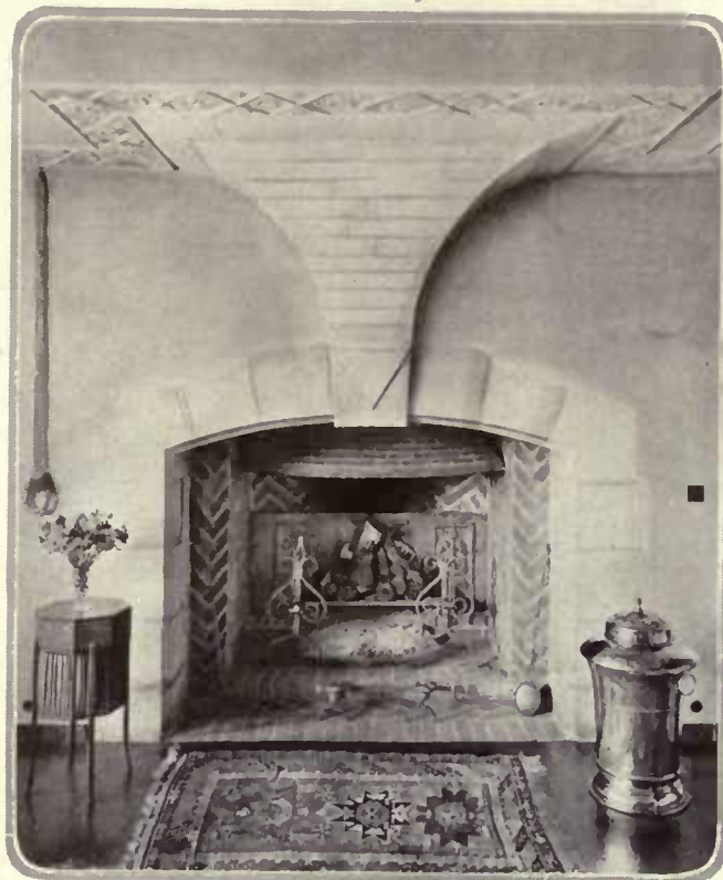
The keystone of the fireplace supports a brick bracket finished with a plaster ornament that extends around the ceiling. From an English house
