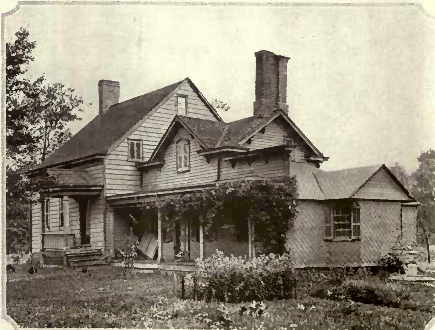
The original house has evidently twice been enlarged, once with the wing and the second time when the shingled, one-story, false-front rooms were added. Yet it has merit worth saving and improving
