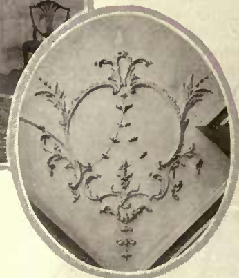
Another of the molded plaster ceiling decorations which are found in the old Powel House at Philadelphia
