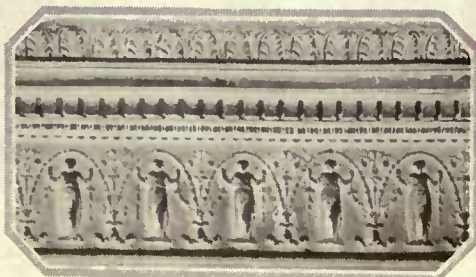
A molded plaster frieze, pilasters and ceiling enrichment enter into the decorative composition of this mid-18th Century dining room. Sir Ernest Newton, architect
