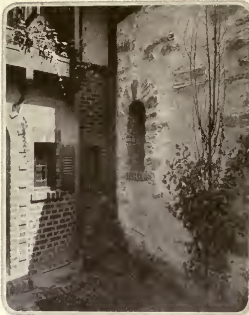
A variety of elements combined make an unusual entrance. D. J. Baum, architect
