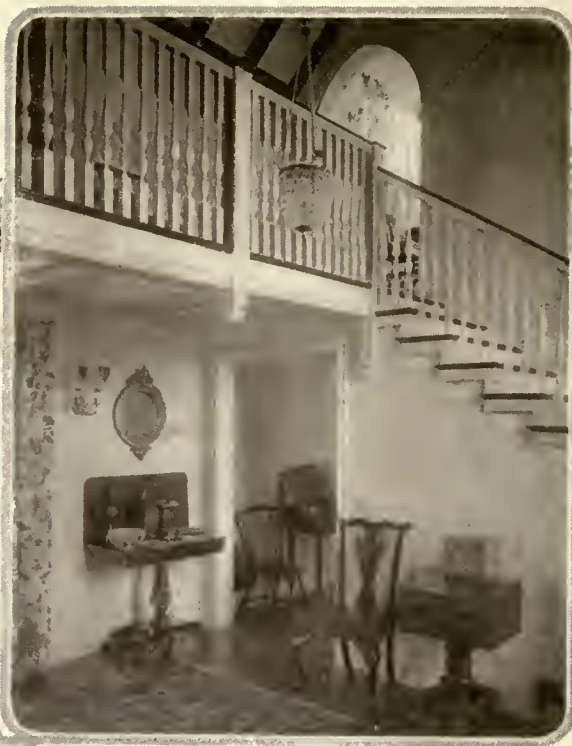
Modern turned spindles of good line are used on the stairs at "Cogskill," the Philadelphia home of Jessie Wilcox Smith. E. B. Gilchrist, architect
