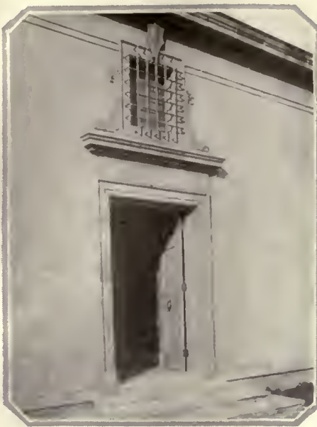
The sharp contrast between this Spanish Renaissance iron window grill and the stucco surface of the wall gives the whole composition a remarkable touch of piquancy. Mellor & Meigs, architects
