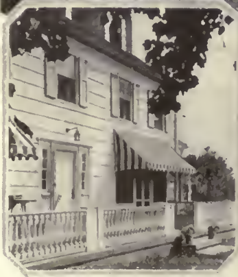
Along the front was built a brick terrace with a balustrade and step leading down to the lawn
