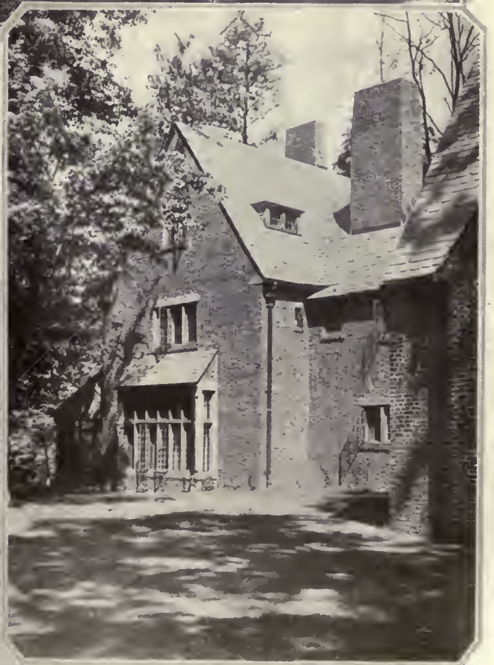
This detail of the exterior shows the uneven quality of the brick and the unusual disposition of the casements that give the façade character
