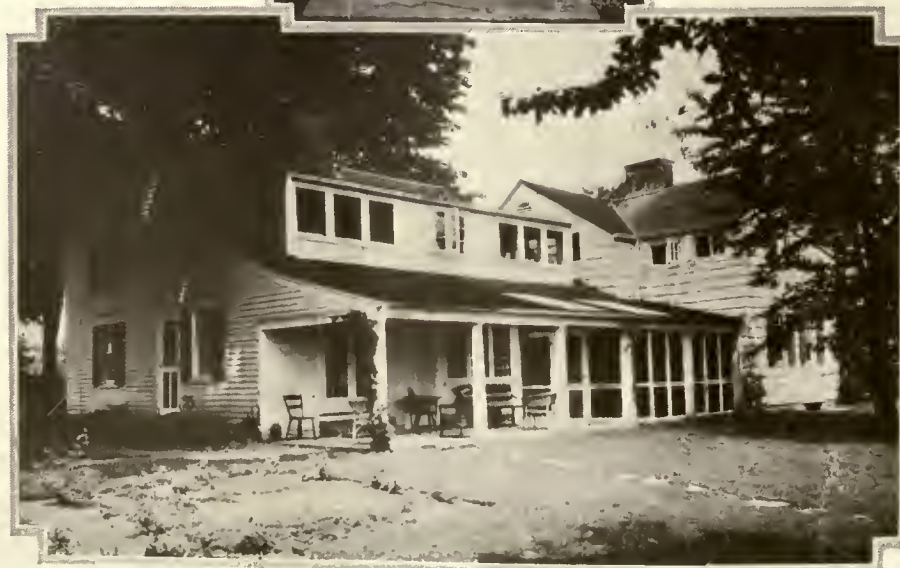
The roof swings low in the rear, covering a broad porch. A long dormer adequately lights the upstairs chambers
