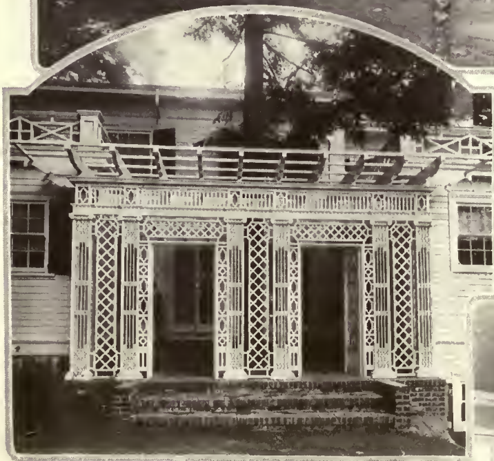
The bricked court is surrounded by an ornate, delicate lattice with pergola roof beams. It is built around a huge fir whose branches shade the spot. This addition gives color to the severely Colonial lines of the rest of the house
