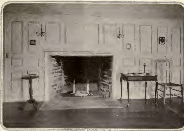
A detail of the living room shows the paneling and fireplace. The frame around the opening, with no mantel shelf, is typical of pre-Revolutionary work
