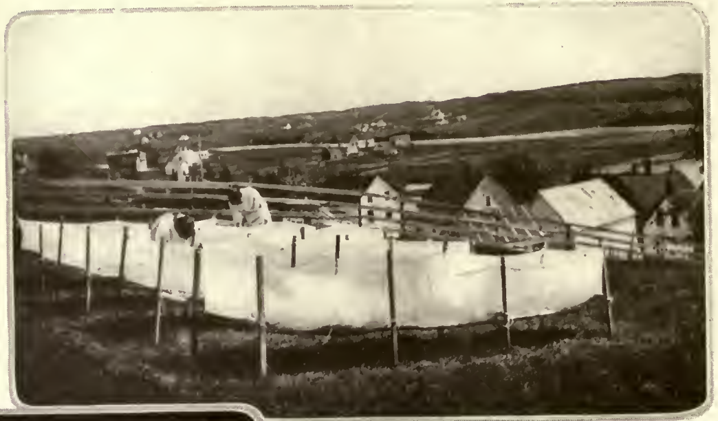
The moss is cured in drying frames of cheesecloth raised from the ground and set up in a spot where there is good air circulation
