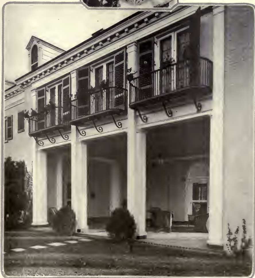
Wrought iron balconies with brackets beneath are used above the sun porch of the Francis L. Hine residence at Lattington Road, L. I. Walker & Gillette, architects
