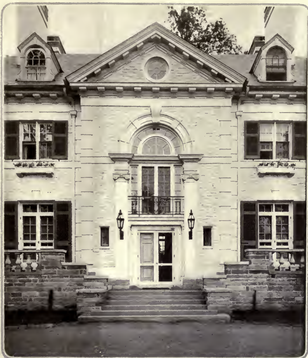
Even in formal architectural work white-wash is permissible and effective as a final coating to rough stone walls
