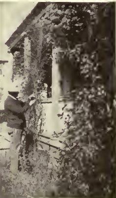
Porch vines, too, need fastening to prevent damage during the winter
