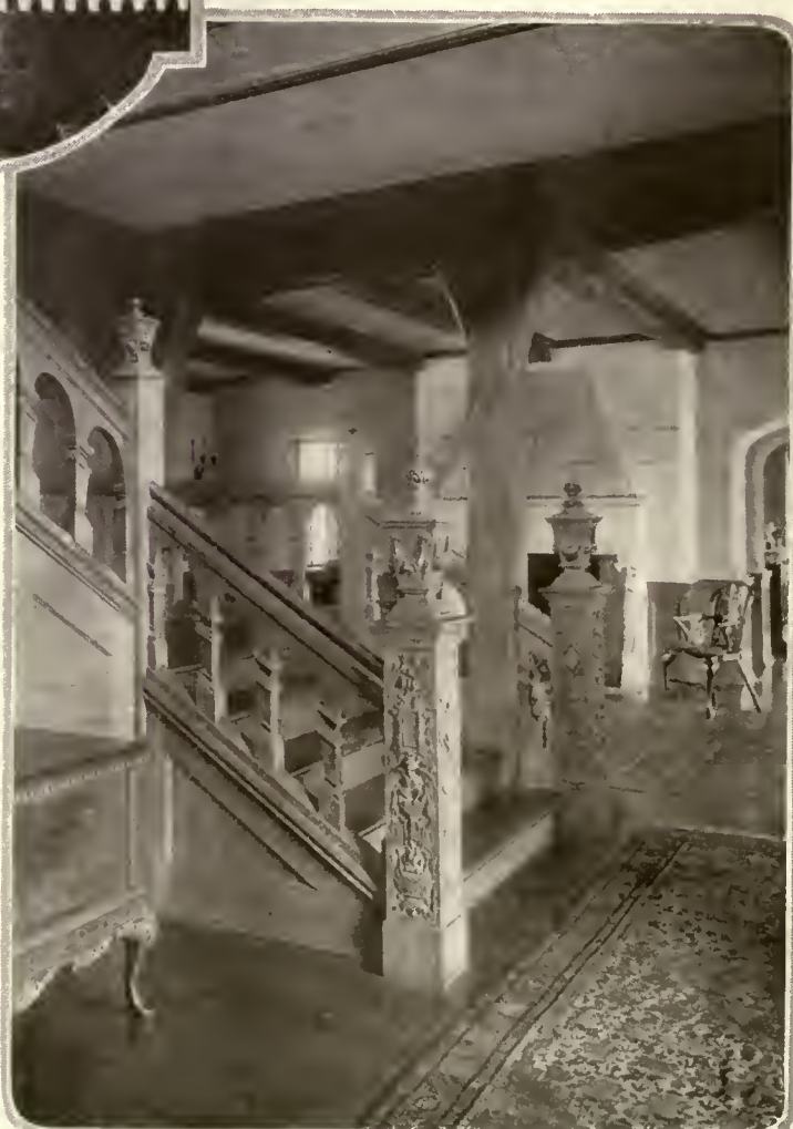
Arcaded English Renaissance spindles and newels, in the home of J. B. Townsend, Esq., Bryn Mawr, Pa. Eyre & McIlvaine, architects
