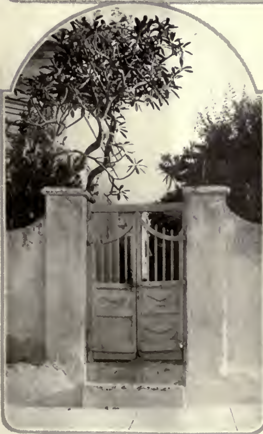
In Bermuda the most prevalent use of white-wash is found. The coral rock walls regularly receive their annual coat, the wash being tinted pink or blue or yellow
