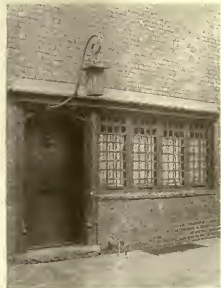
Wrought iron window grill, showing adaptation of Italian inspiration to modern needs. Mellor & Meigs, architects
