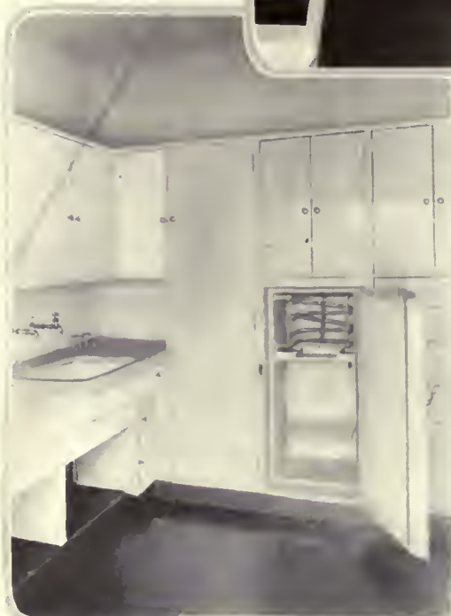
Another view of the same kitchen shows the electric coils for keeping the ice box cool, and the sanitary cabinets
