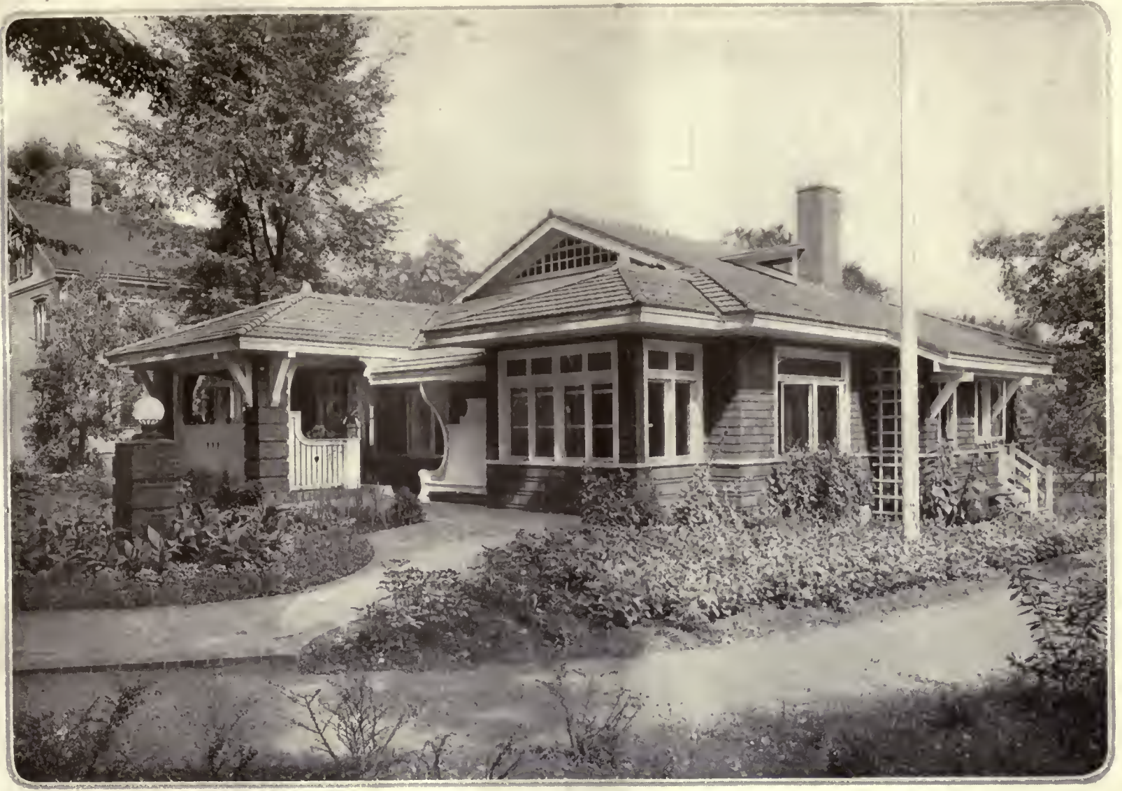
The exterior shows a clever adaptation of the bungalow idea to a structure containing interior features usually possible only in a full sized house. The walls, floors and ceilings are insulated with seaweed, resulting in winter warmth and summer coolness
