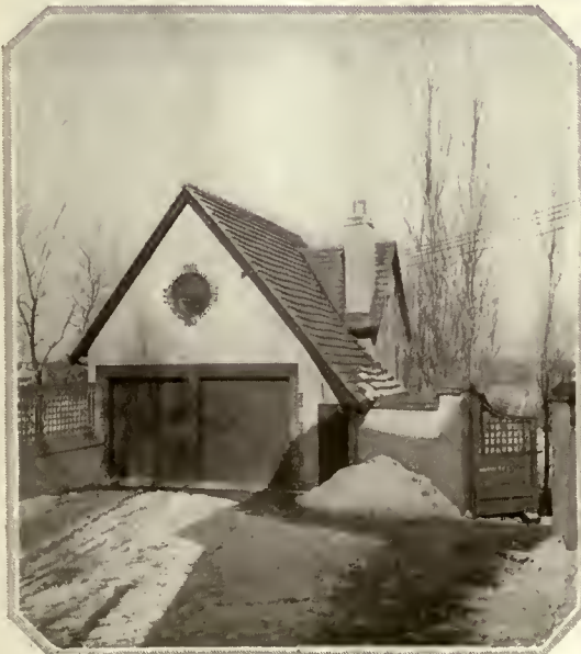
The main necessity in any garage entrance is ample door space. As in this case, which is on the property of G. W. Davidson, Esq., at Greenwich, Conn., practically the entire façade has doors. G. J. Harmon, architect
