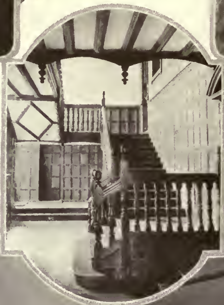
The substantial characteristics of late 17th Century spindles and newels are found in the hall at "Heale House," Salisbury, England
