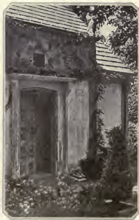
A quaint entrance was made with an old carved wood paneled door and stone architrave. To make this Tudor door the architect used old stone fragments and two stone heads. A candle fixture set in the little window above lights the doorway and vestibule
