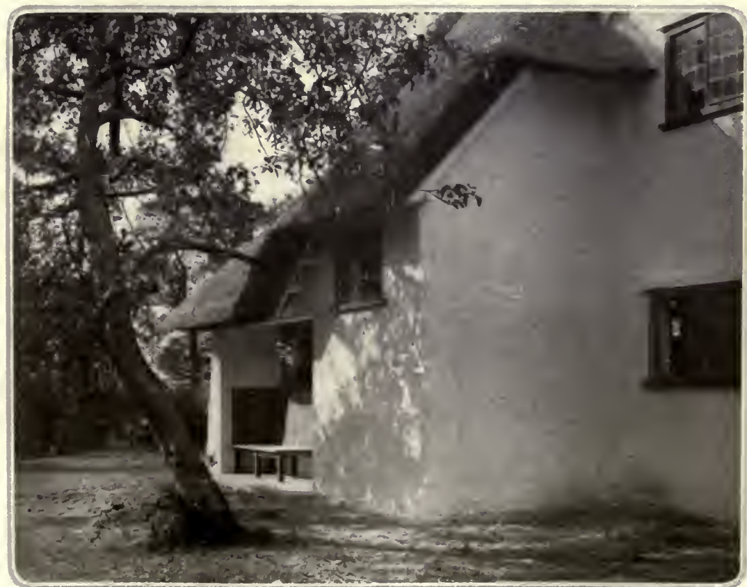
Even in formal architectural work white-wash is permissible and effective as a final coating to rough stone walls
