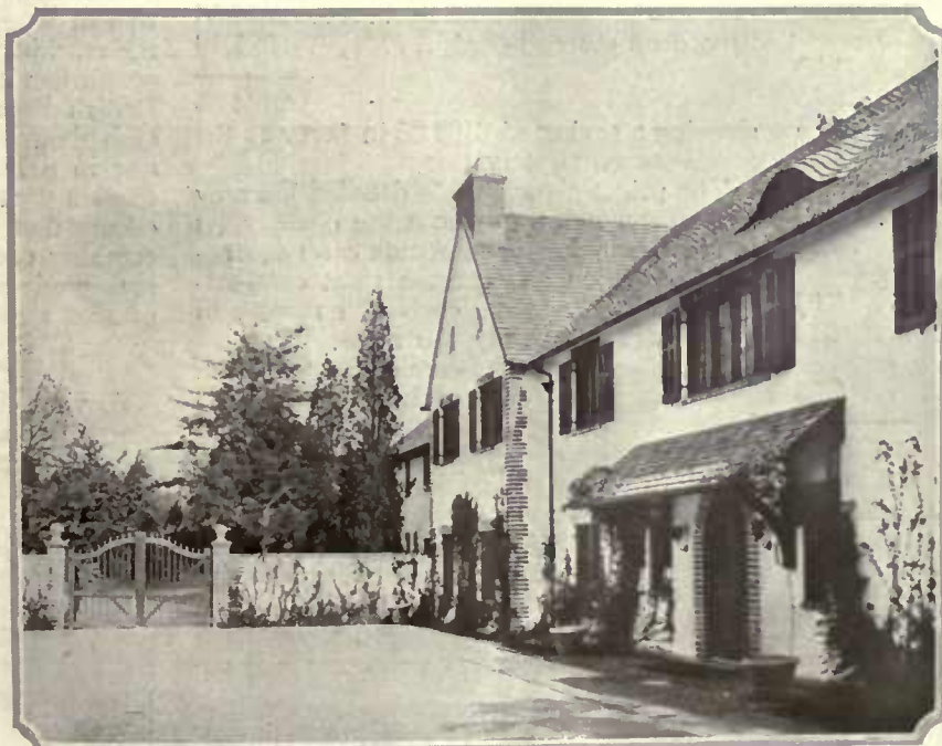
Stucco can be successfully combined with so many other elements that its uses are almost legion. Stone and stucco, tile and stucco or half timber and stucco, and as here, brick and stucco, are among the combinations. Residence of B. Winthrop, Esq., at Syosset, L. I. Delano & Aldrich, architects
