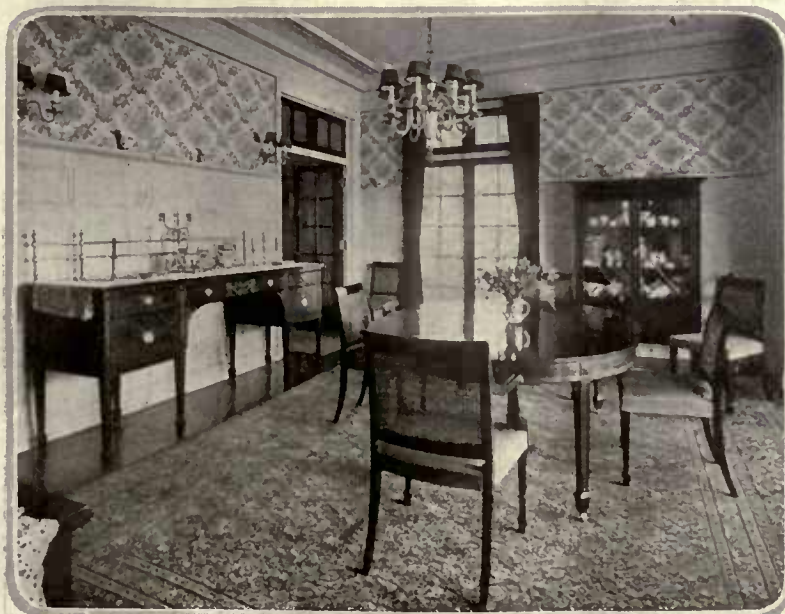
In some cases the woodwork was restricted to a chair rail; in others it was developed into a wainscot topped with a rail or even a ceiling-high paneling
