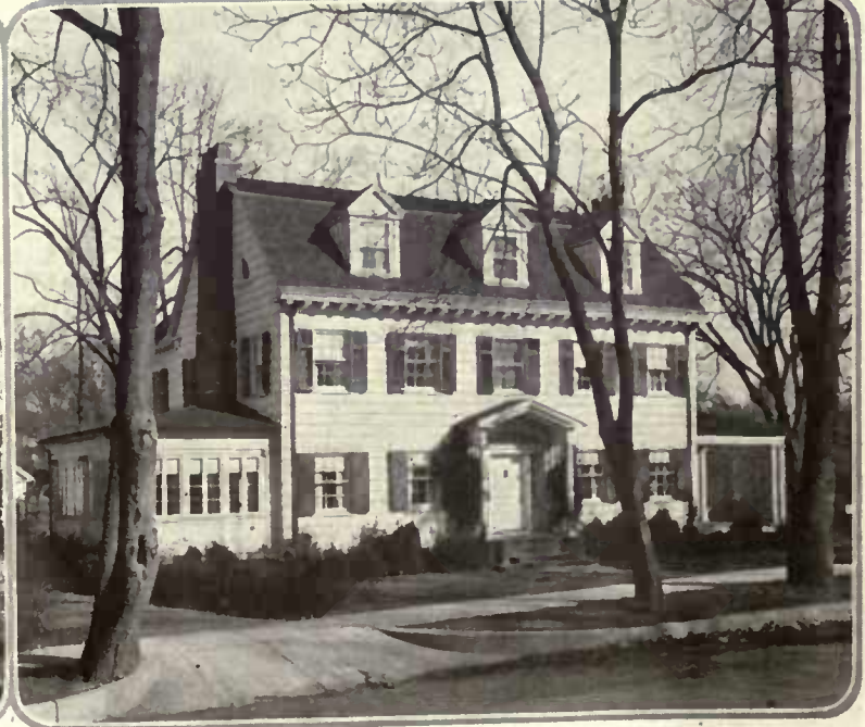
Balance is the keynote of the Colonial design. There are chimneys at each end, and each end terminates in a porch, open or enclosed as here in the Mix residence at Cranford, N. J.
