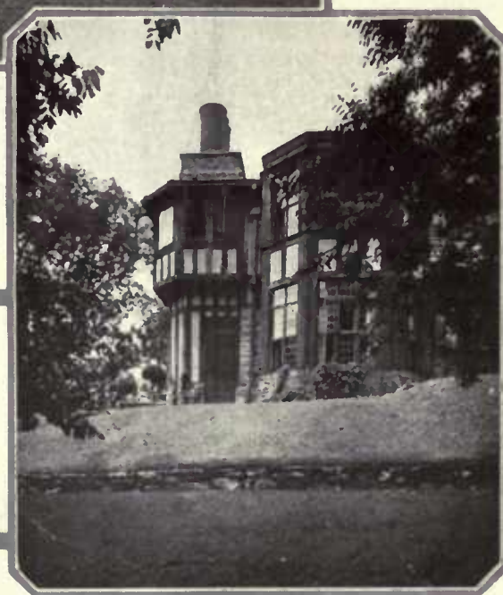
The overhanging story is an inheritance from old times. So are the leaded windows and the towering chimney pots above
