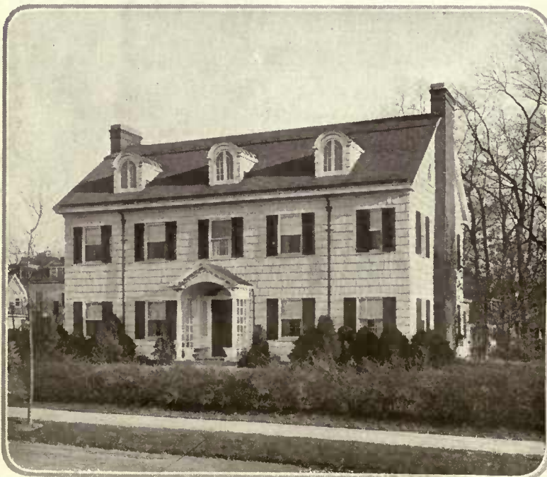
Texture was given the walls of old Colonial homes by the use of hand-hewn shingles. This same charm is imparted by them to the modern residence of Louis A. Mathey, Esq., Cranford, N. J.
