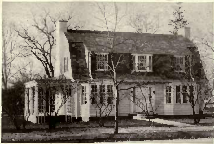
House on Fresh Pond Parkway, Cambridge, Mass. Charles R. Greco, Architect, Boston, Mass.
