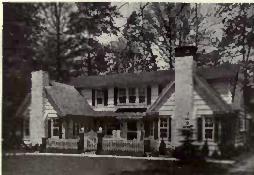
There is a little 'vest pocket house' in November, made of shingle, built around a court. The very sort of house you hope some day to build
