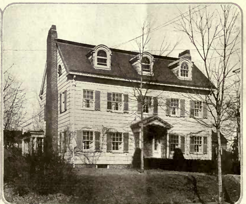
In grouping the windows at the right and left of the entrance consideration of the one room treatment is born in mind, so that these windows, although separated, form one composition
