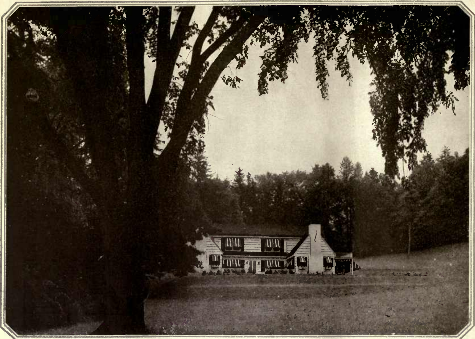
The house has a background of trees that set off the white walls. Chester A. Patterson, architect
