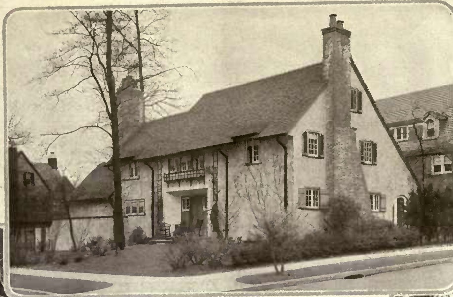
Among the unusual features is the walled-in front garden, lending an atmosphere of secrecy and privacy to the garden. A brick coping adds a touch of color to the rough stucco finish. A heavy gate pierces the wall. The residence of Charles A. Miller, Esq., Forest Hills, L. I.
