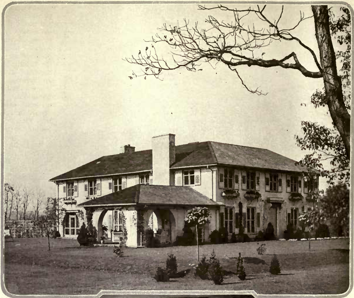
Almost the first thing one notices about the house is its abundance of windows and doors and the consequent profusion of light in the rooms. The roof is unusual
