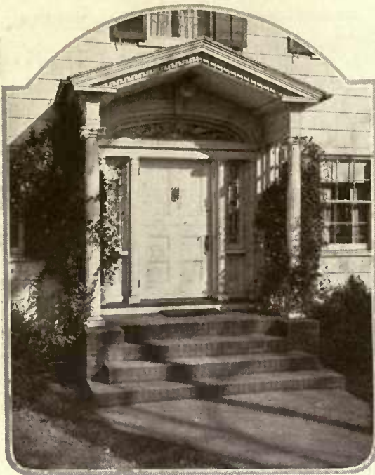
The Colonial exterior follows the rule of marking the main entrance at the center of the house by a simple porch. This is on the residence of Robert J. Mix, Esq., at Cranford, N. J.
