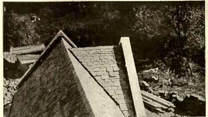
A good example of a varied graduated roof surface, showing large slates laid wide to the weather and smaller slates near the ridge
