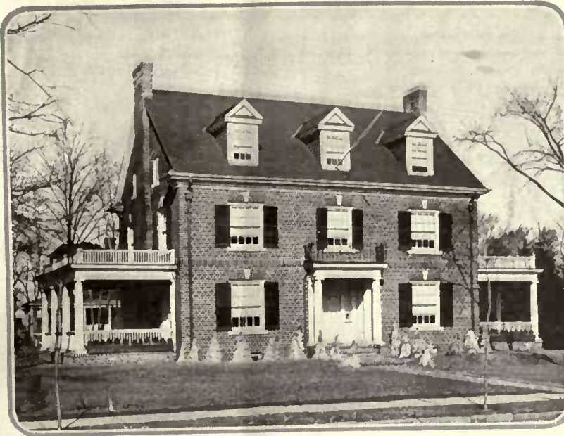
Where porches flank the ends, the column and cornice treatment of the entrance is repeated, but usually the side porch roofs are flat decks. Residence of Dr. Frank Moore, Rahway, N. J.
