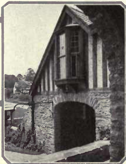
Stone on the first floor gives a solid basis for the house. It crops out naturally as stone crops out on a hillside
