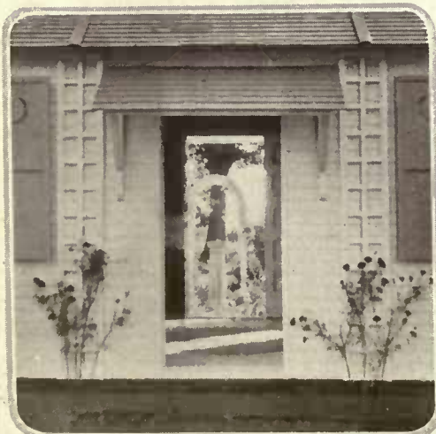
Door hoods and lattice panels for each side of the doors were among the extras that were added
