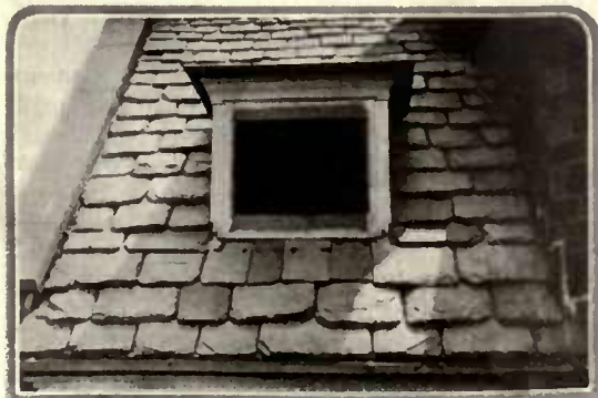
A beautiful example of well selected slate laid in contrast to adjoining masonry and detail of dormer
