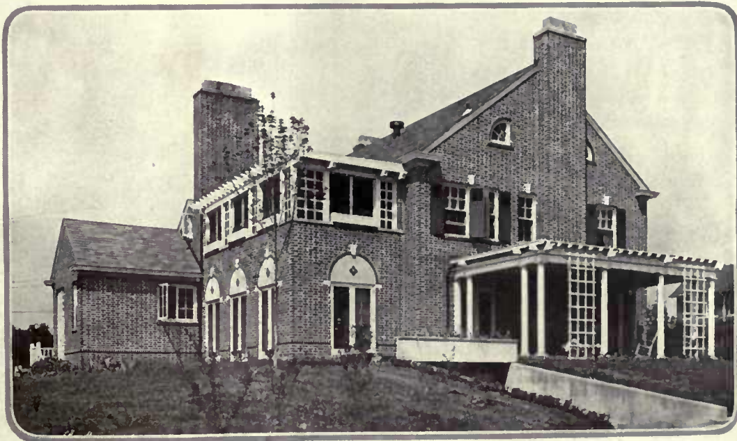
The front elevation shows a house of the simplest Colonial lines, interest being found in the color of the brick, the white trim, entrance and end porch, the blinds and the white keystones. A year's planting is but just under way
