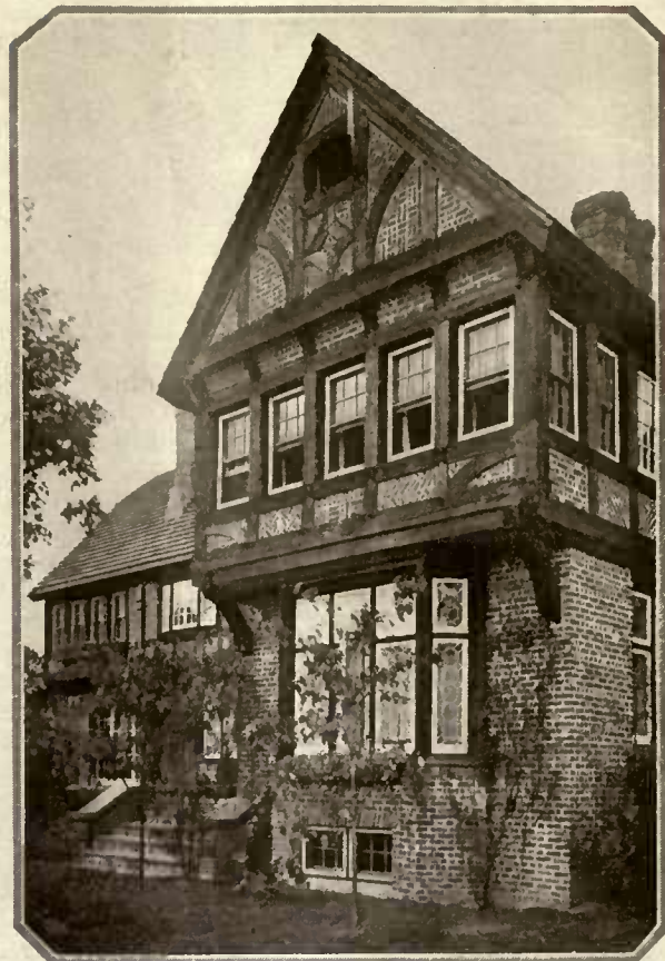
Brick nogging—the filling in between the timbers—can be laid in any pattern desired. A variety of designs are shown on this façade
