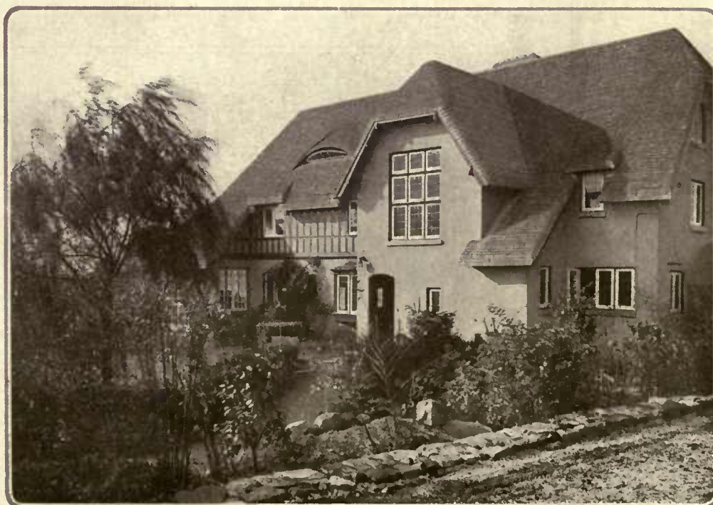
The thatch simulation is successfully carried out with shingle in the curves and valleys of this roof. It covers the residence of Mr. Burrows at Hartsdale, N. Y., of which A. J. Bodker was architect
