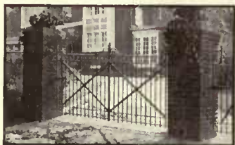
Railings and Gates
