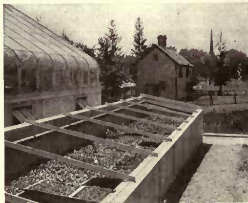
When it comes to hotbeds and cold-frames the possibilities are almost unlimited. Concrete is used here for greater endurance
