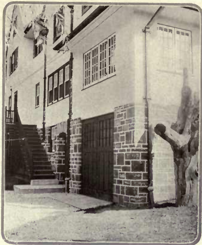
A third example of the garage in the house—to the right—shows it an integral part of the foundation. A glassed-in porch is above. The kitchen being at this end of the house, the service quarters are kept separate
