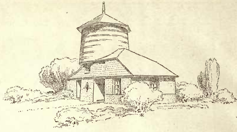
A successful grouping shows engine house and elevated tank in a compact unit. Below the tank is provided a room for tools
