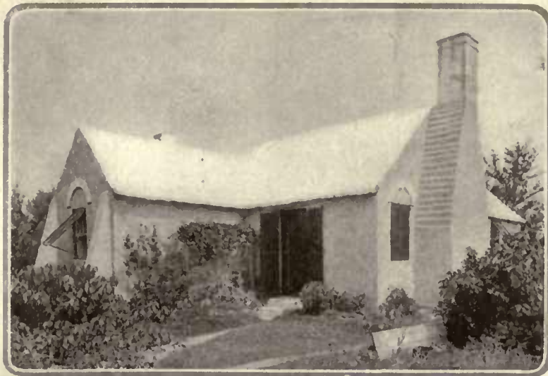
"St. John's Hill House," built about 1688, is reminiscent of Gothic days in its buttresses, high arched dripstones and the finial surmounting the gable peak. The walls and roof at the gable ends join at right angles without any barge, capping or eave projection
