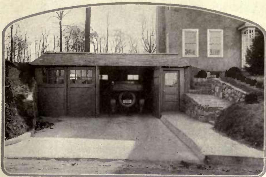
A hillside always provides the possibility of a garage. In the case above it has been fitted snugly into the scheme, its roof coming slightly above the terrace level. The flat part of the roof can be used as a porch
