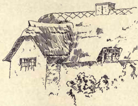
The effect on the ridge of a rye thatch roof is not unlike that of a stiff, straight comb
