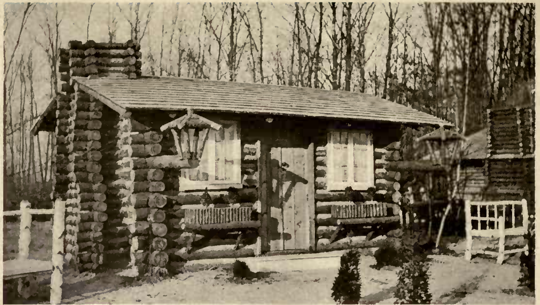
Fifty-five cedar logs of varying lengths went into the building of this cabin. The logs are left in the rough outside and stripped and oiled within. Cement was used for caulking. The cost, including labor, was approximately $450
