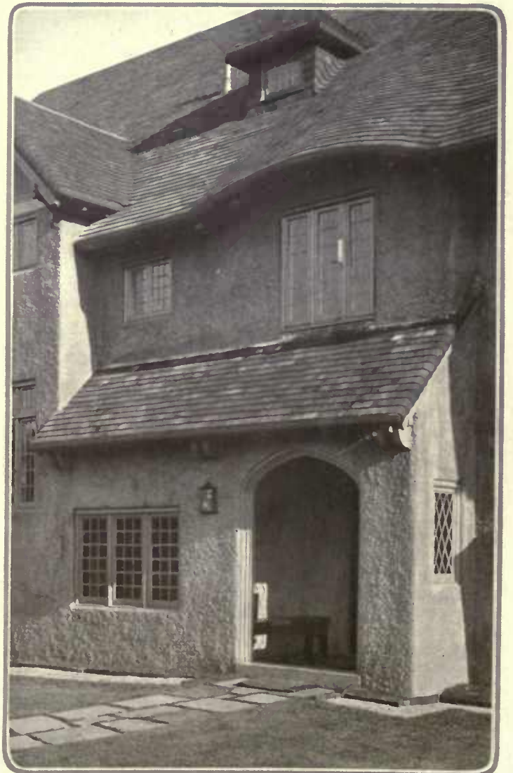
Although the materials of construction offer no unusual features, distinction is given by the method of handling them. The exterior walls are finished in grey stucco and the roof shingling is carried out in a manner to simulate the rounded and softened lines of ancient thatch. The massing of the house, the grouping of the windows and the relation of the house to the land are reminiscent of the English work of Baillie Scott
