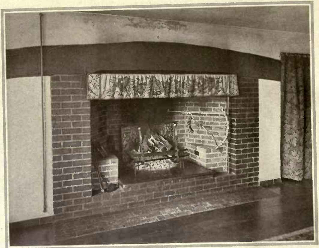
In this view of an English cottage fireplace can be seen the primitive use of the smoke valance. It served a purely practical, utilitarian purpose
