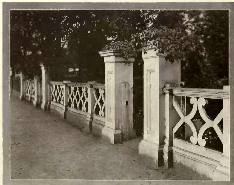
In New England many of the old Colonial fences still stand. Since they were built of white pine, they are still in good condition
