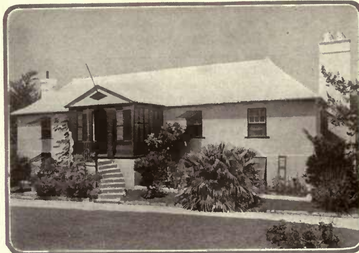
In its hipped roof, modified classical porch and general plan—which is in the form of an "E" with wings projecting toward the water front, "Waterville" exhibits decided Queen Anne influence
