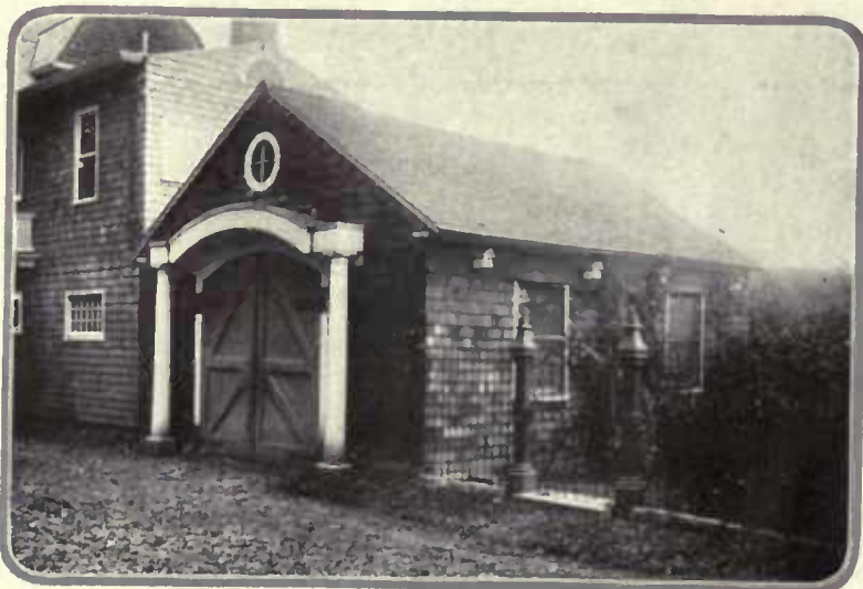
Another example of the garage treated in the same manner as the house. It is unobtrusive and well lighted. The door is generously wide. The bird house decorations under the eaves are a whimsical touch that is pleasing
