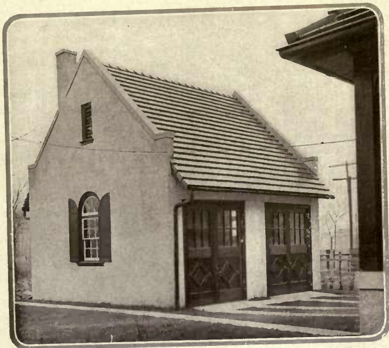
The high roof of the garage above allows for a half story attic where winter tops can be stored in summer and extra supplies kept. With vines trained up the walls or a border planting at the foundation it becomes a worth while addition to the garden
