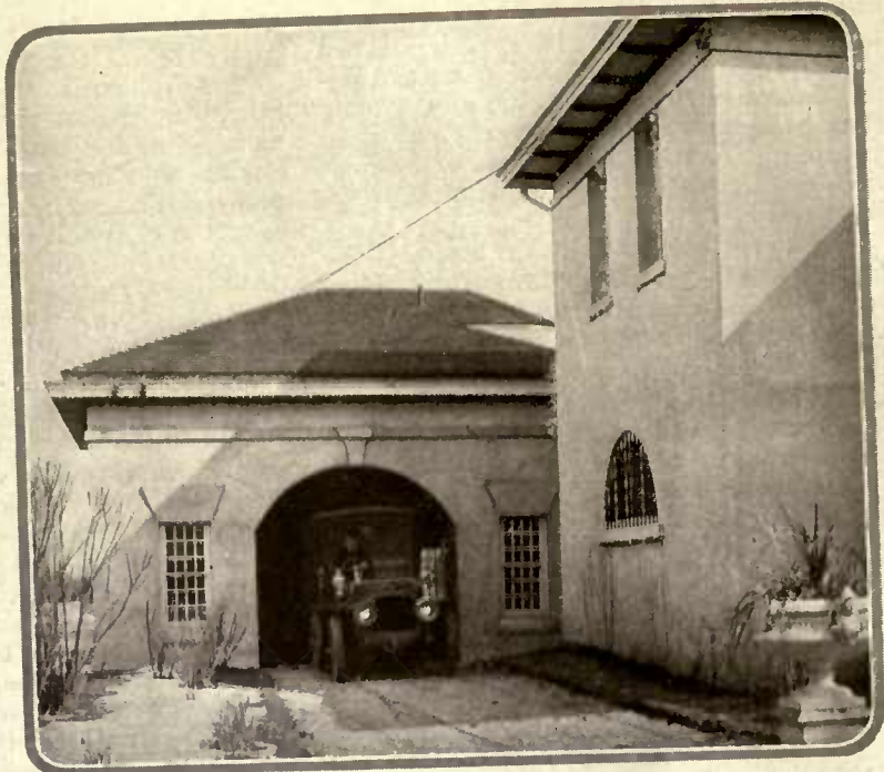
The garage as one unit in a series of attached buildings can also serve the purpose of holding the heating plant, the chauffeur being stokesman in winter. The peculiar advantage in the garage above is the wide door. Many garages have doors too narrow
