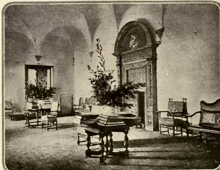
Fig. 18. Italian furniture was in excellent harmony with the plain whitewashed walls and the groined and vaulted ceilings. In the Villa Curonia is this original architectural background
