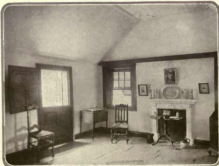
At "Waterlot" the parlour—to use the good old English name—has a "tray" ceiling, carried up to the height of the roof, keeping the room cool. This ceiling can be adapted to American summer homes
