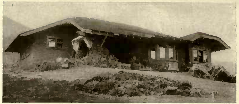
Wood in some form is the only exterior treatment which would so well tie this bungalow to its site and give it its definitely homelike charm. Horizontal clapboards instead of stained shingles might have been used
