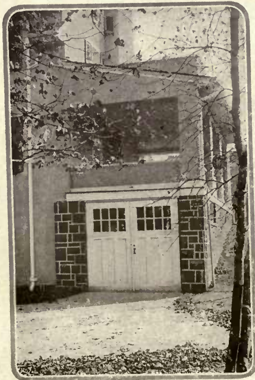
Below is one type of garage in the house. It is cut into a bank and forms the foundation for the porch. Windows on the side provide sufficient light. Being a part of the house it requires no extra heating plant and the car is conveniently at hand
