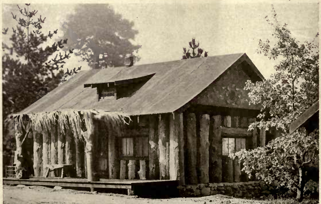
A California cabin was built of vertical logs set on a stone foundation and caulked with cement. The gable ends are buff stucco and the roof tar paper. The cost, including labor, was approximately $400
