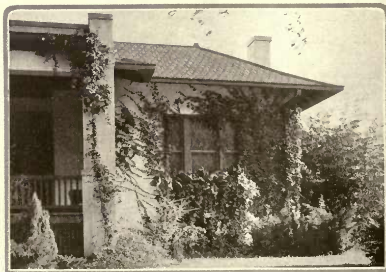
Steel window boxes holding ferns and geraniums add the final touch to the house planting. In the right background Japanese bamboo forms a screen for the servants' quarters
