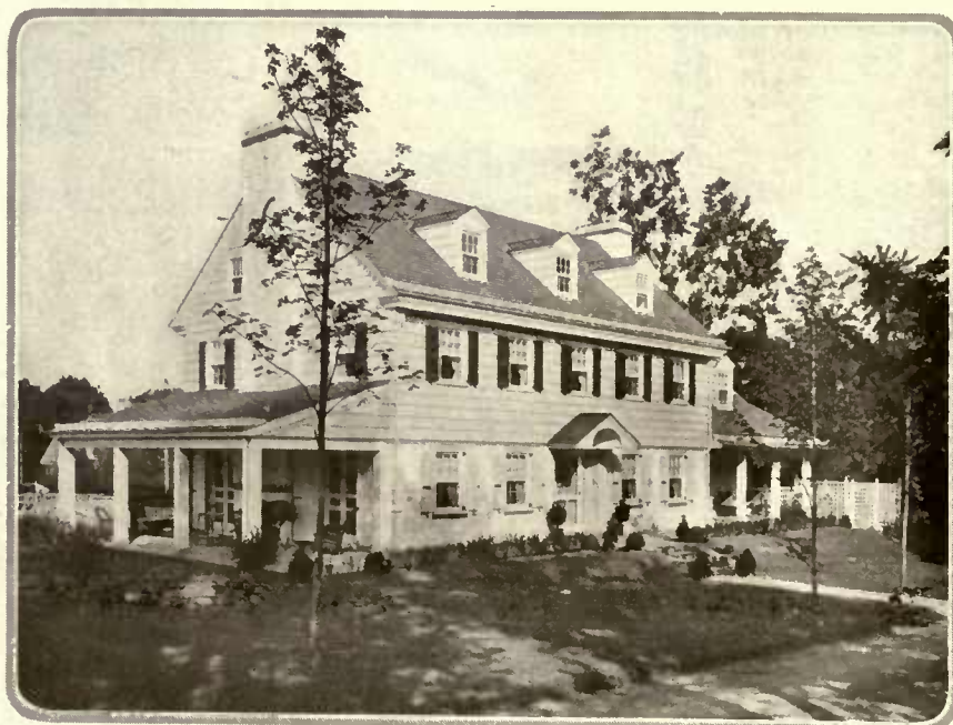
The architecture is a successful fusion of several distinct Colonial types with the Pennsylvania farmhouse style predominating. White-washed local stone constitutes the lower portion of the exterior walls. Above, the walls are sheathed with shingles painted white. Color relief is given by the dark green blinds and the weathered shingle roof
