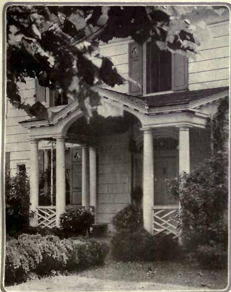
The entrance porch is an elaboration of the usual Colonial stoop, the balustrading being the same as that used on the garden side of the house. Color relief is given the white shingled walls by the green blinds and box-bordered path
