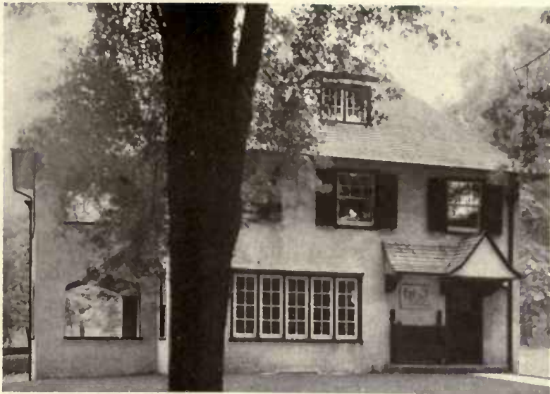
Another square type of house, this time in New York. The construction is stucco over hollow tile. A large cast has been set in over the entrance bench. Above the side porch is a sleeping porch
