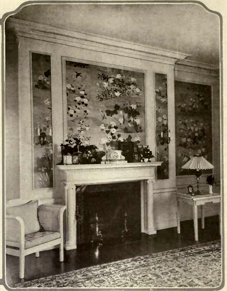
The ornate wood paneling on the dining-room above can be reproduced at a minimum expense by nailing moulding to the wall and painting it. Care should be taken in the proportions of the panels
