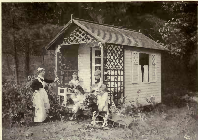
© E. F. Hodgson Co. An attractive little house up whose trellises vines can be trained. It is made of cedar, and has a 6' x 7' room and 3' x 6' porch with two seats
