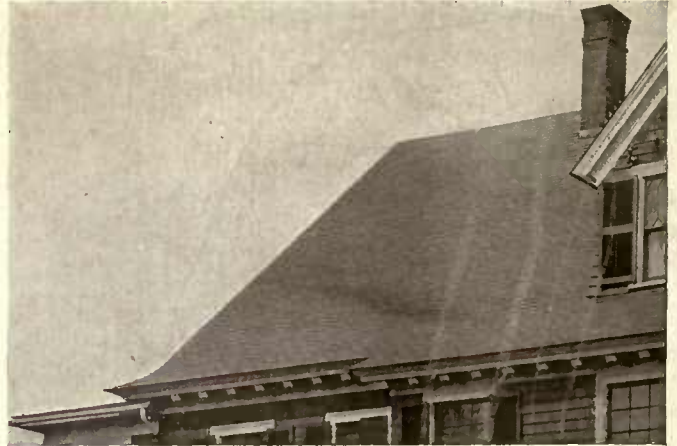
WORCESTER RESIDENCE Roofed with SMALL (9"x7") LUSTRE-SLATE
