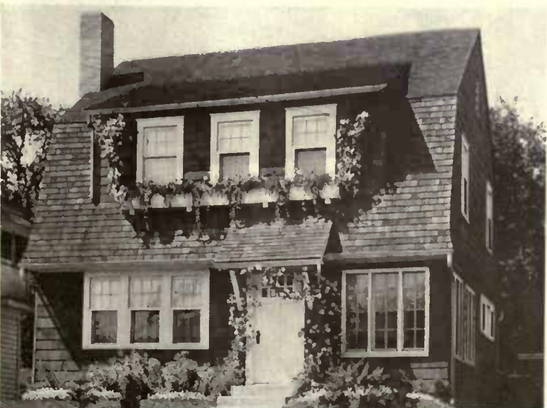
O. F. Conner, architect This type in Ohio serves to show one unit of Dutch Colonial. The North Carolina house opposite shows the same original unit expanded. Pitch of roof, fenestration and stained shingle differ
