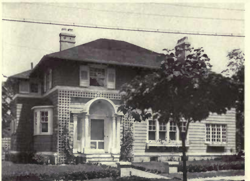
R. C. Edwards, architect The timber frame of this house has been clothed with shingles stained brown. The shutters, wood trim and lattice are painted white. Two sets of grouped windows add interest to the front
