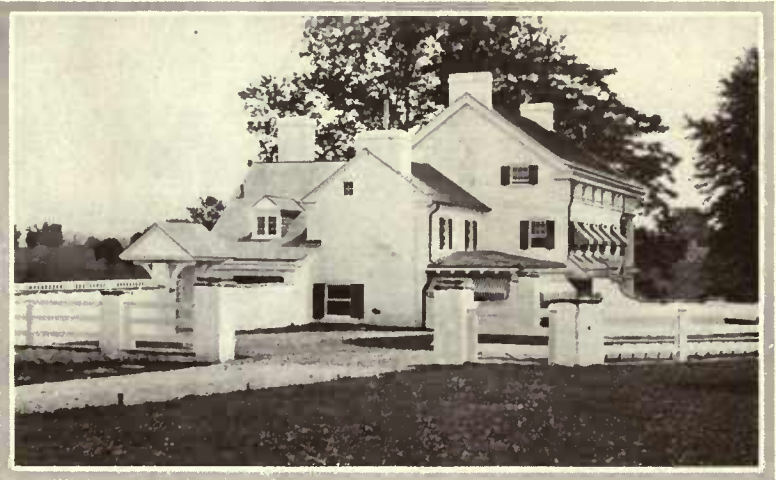
Then mark the changes in roof line, the addition of the service quarters and the entrance improvements that gave the house a sense of privacy
