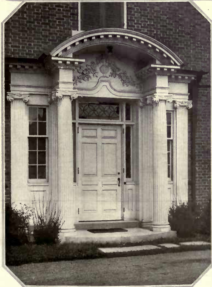
Among the interesting details is the entrance, a hooded pediment of classical design with a carved entablature, supported and flanked by Ionic columns and pilasters
