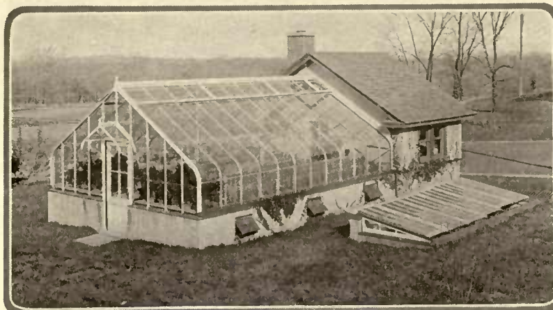
The "single-unit" house, measuring about 25' in length and set on a concrete foundation, is small but capable of producing real results. Its length can readily be extended if desired
