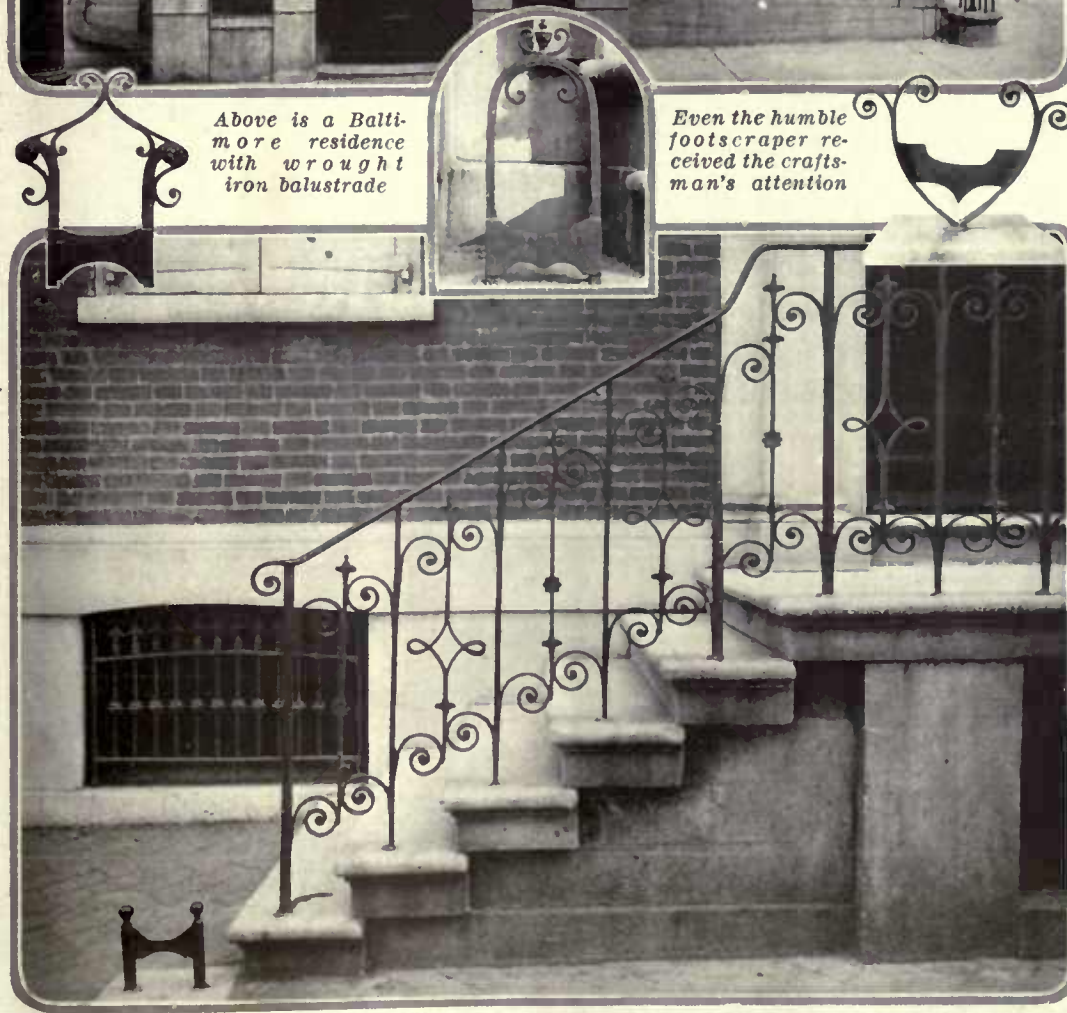
In Philadelphia, where the houses approached the building line, a suitable entrance for the door had to be provided. This was effected by stone steps and an iron railing. The color value of the iron can be visualized from this combination with bricks and stone
