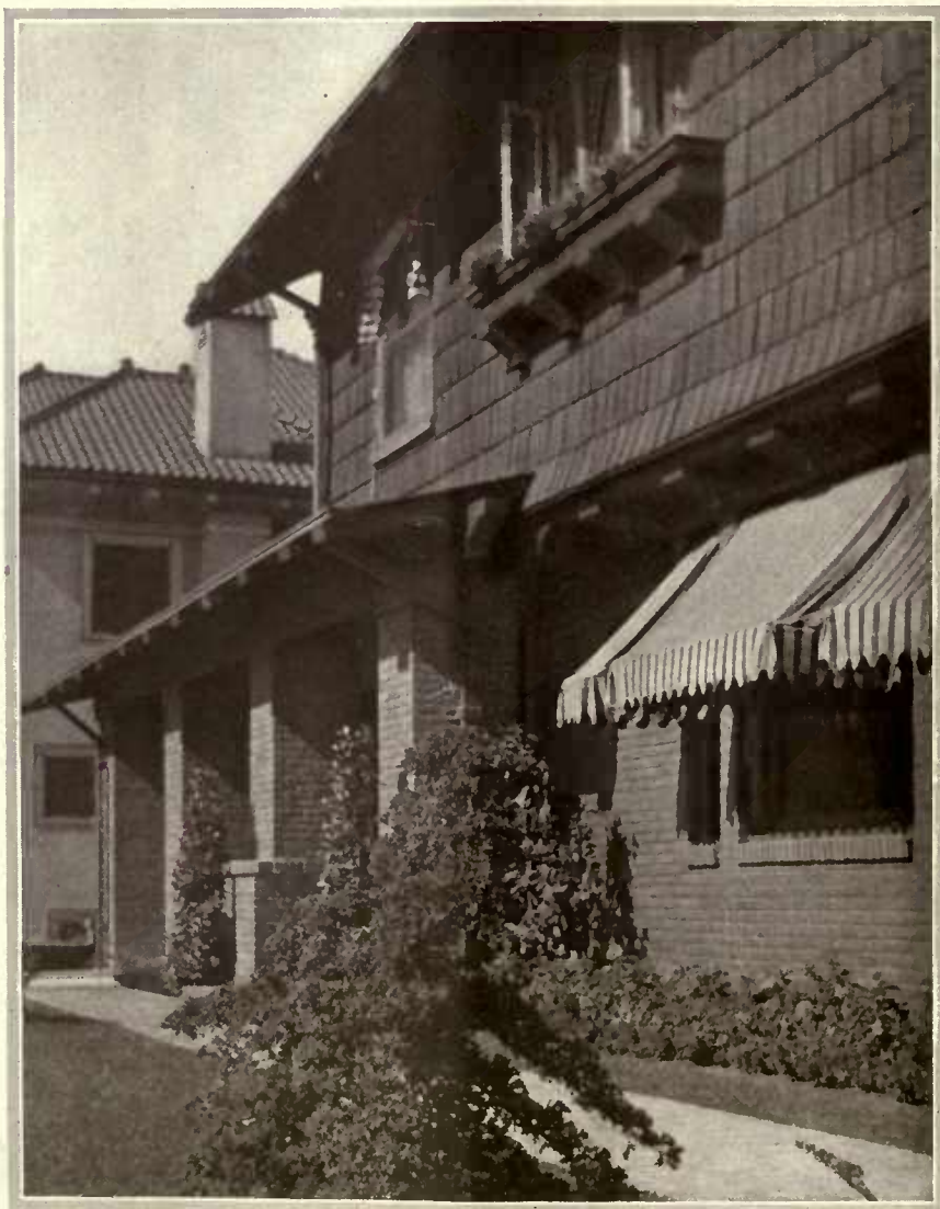
When properly handled shakes and masonry combine well, as here, where the wide jointed brickwork combines in perfect harmony with the shakes above
