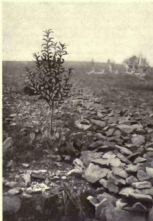
The hillside gullies worn by the rain were filled with stone which will eventually catch and hold the soil
