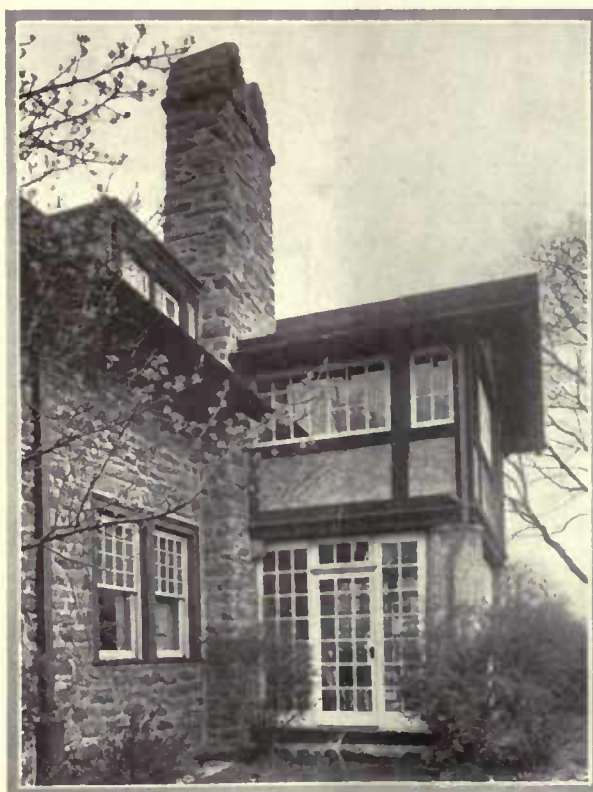
A close view showing the porch and the sleeping porch above. The walls are rubble built of native Chestnut Hill stone
