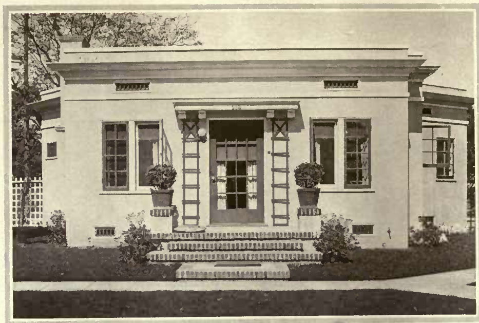
It is neither a bungalow, a shack, a seaside cottage nor a mountain camp, but a house built of tile and stucco and adorned with brick trim, where two more or less conventional people live permanently
