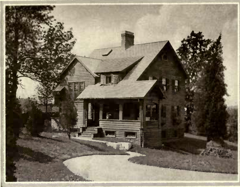
The original house was a comfortable cottage, indigenous to the rugged New England hills that surround it, both in color and design. Its one fault was a lack of adequate accommodations
