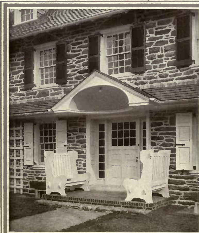
The "Germantown hood" is an outgrowth of the pent roof, originally attached to Colonial houses. The benches shown are also a modern elaboration
