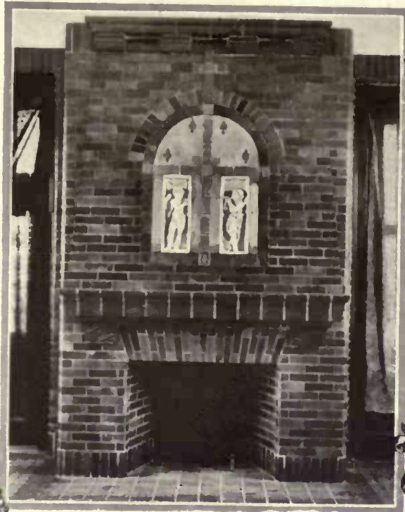
By the use of tile inserts and tile figures the fireplace in this nursery has been given genuine interest
