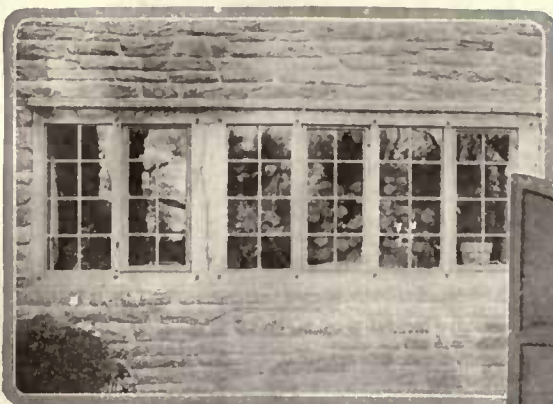
A range of leaded casement windows, suitable for a country house. The framework is oak, without any sort of finish, fastened together with oak pins which project
