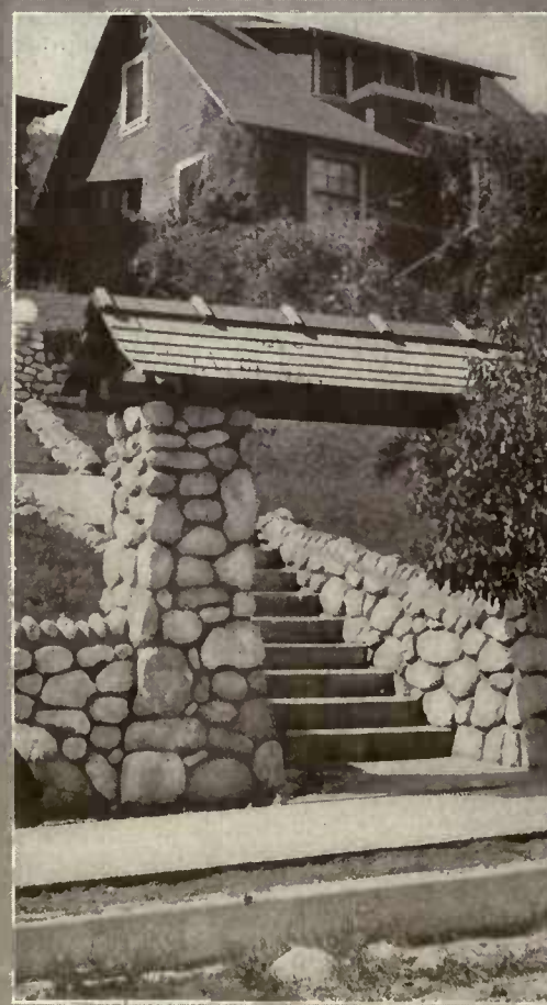
The roofed gate idea came from the lych gate of the English rural church. Here it is modified to suit its use with boulder pillars in a New Jersey garden
