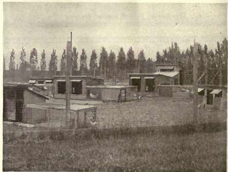
The eastern entrance to the Homestead Campine Farms Poultry Yards, showing the houses for the young stock. The birds remain in these houses with wire runs until they are about six weeks old, when they have free range until they are brought in for their winter quarters
