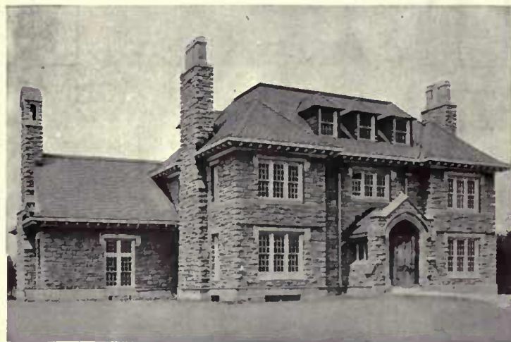
New residence of Spencer Kellogg, Jr., Buffalo, N. Y. Roofed with \frac{1}{2} " "Smooth thick," 18" x 10"
