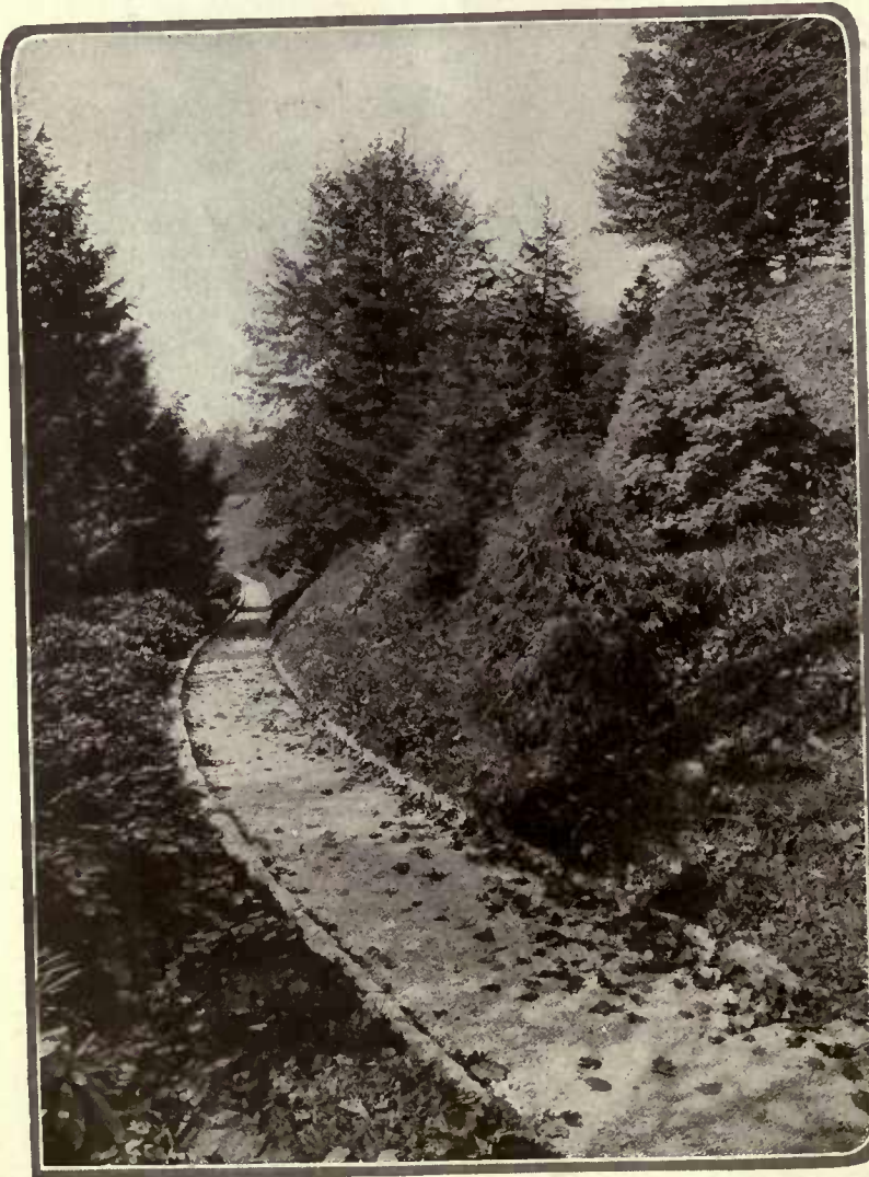
There should be a definite reason for the path curving. Sometimes it avoids a large tree or skirts an embankment, as here. This also is an example of a concrete path treated with a naturalistic pebble finish
