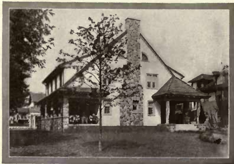
A. Raymond Ellis, architect Two similar houses. This one was built of frame covered with stucco, in Akron, Ohio, and cost about $14,000
