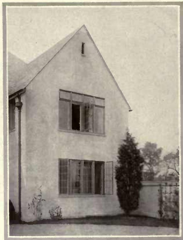
A flat stucco wall face totally unadorned. But casement windows give it the master touch. Delano & Aldrich, architects
