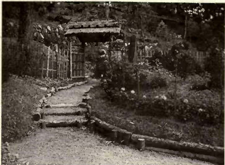
The Nipponese use of rustic timber, wattles and thatch is shown in this gate to the Japanese garden of C. Brown, Esq., on Staten Island, New York. T. Shiota, landscape architect
