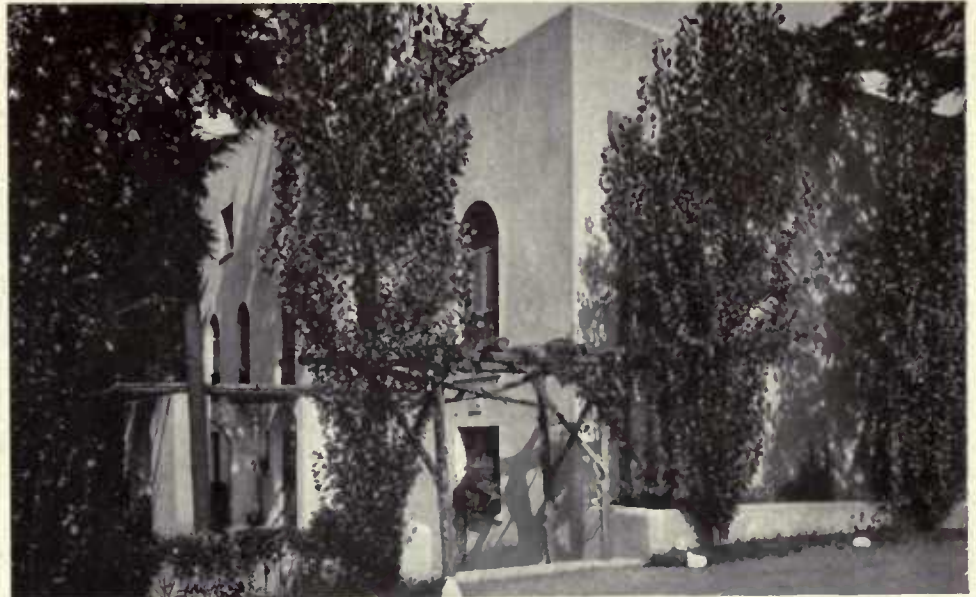
Hollow tile was used—6,500 of them put in place by three masons and seven helpers in twenty-seven working days. The whole was then covered with cement. There is one chimney to serve the four flues
