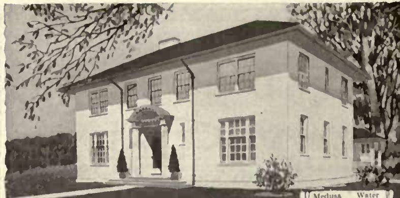
Medusa Water proofed White Portland Cement Exterior on Hol- low Tile
