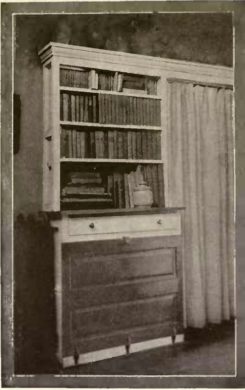
Figure IV—Used to conceal an ugly jog in the wall, this type of bookcase and cupboard can readily be made by the amateur from the scale drawing shown below
