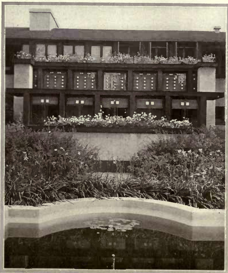
The residence of E. E. Boynton, Esq., at Rochester, N. Y., is built along the Frank Lloyd Wright lines, admitting an unusual display of window-boxes. Pitkin & Weinrichter, landscape architects
