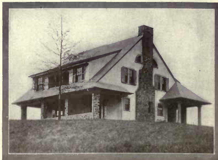
A. Raymond Ellis, architect Built from the plan of that shown above, this house erected in Newington, Conn., with slate roof and stone chimney, cost about $10,000
