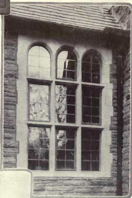
The idea of the old English iron casement is being adapted successfully by American architects. They are modernly practical and yet lack none of the old charm. In a house of English Tudor or Elizabethan design, such as this, nothing is more suitable than a tiered and stone mullioned staircase leaded casement window. Edmund B. Gilchrist, architect
