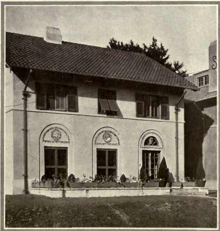
The factors which here mitigate the concrete nakedness are the wide overhanging eaves, the small window and door panes, the indented arches and mosaic work. Mann & MacNeille, architects
