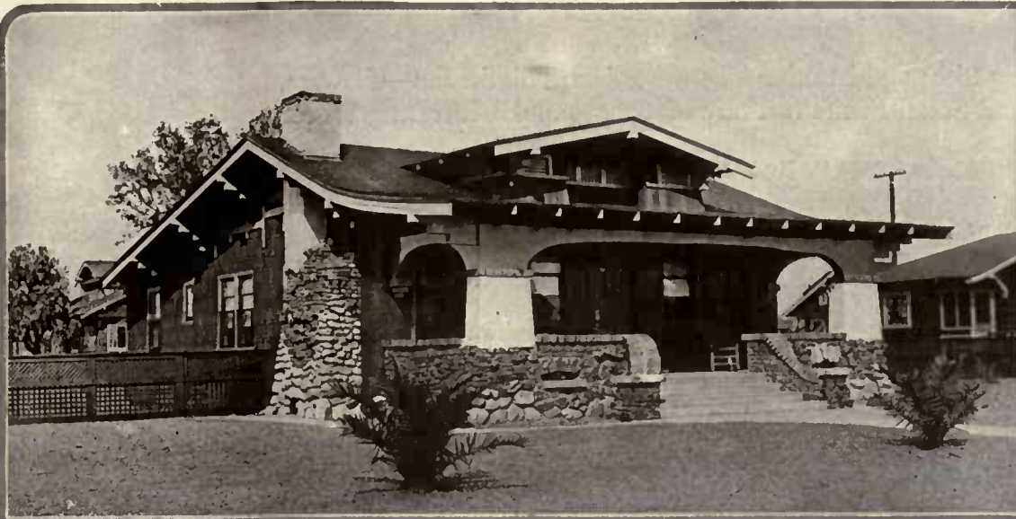
Grey cobblestones, dark red clinker brick and cream-tinted stucco comprise the masonry work, dark brown stained shakes cover the walls and shingles painted a soft green shade constitute the roofing, while the trimming is done in creamy white. The main front door opens directly into the living-room, but from the veranda also lead two pairs of French doors—one into a den and the other into the music-room. These three rooms, occupying the front of the house, are connected by broad colonnade openings. Approximate cost, $3,500. F. A. Brown, architect
