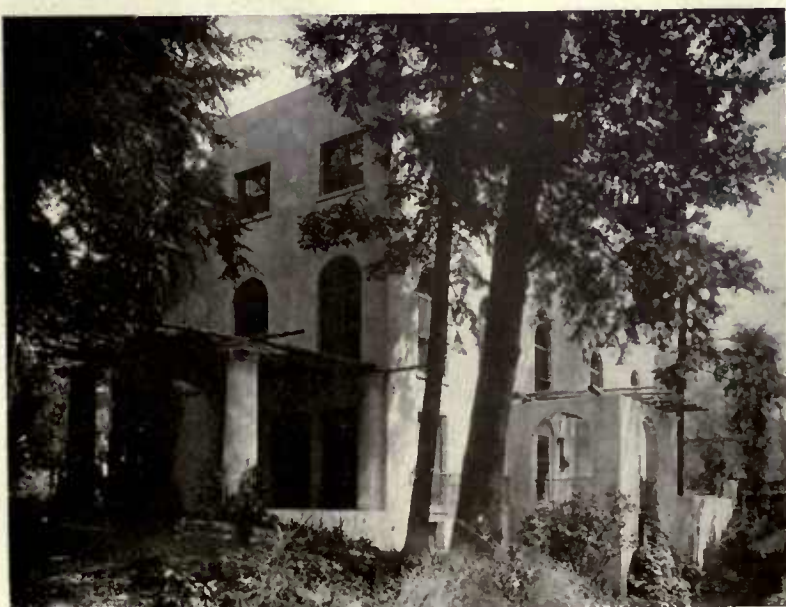
The house contains five bedrooms, three baths, dining-room, kitchen, pantry, laundry, workroom, studio, dining-porch and flat roof. The last feature is well used as a sleeping porch
