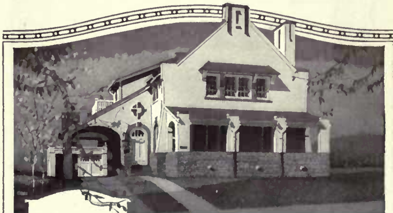
Residence of Dr. A. L. Kennedy, Denver, Colorado, Biscoe & Hewitt, Architects.
