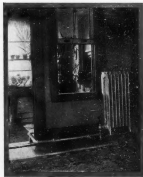
By elevating the radiator, a water pocket was avoided and the proper drainage assured
