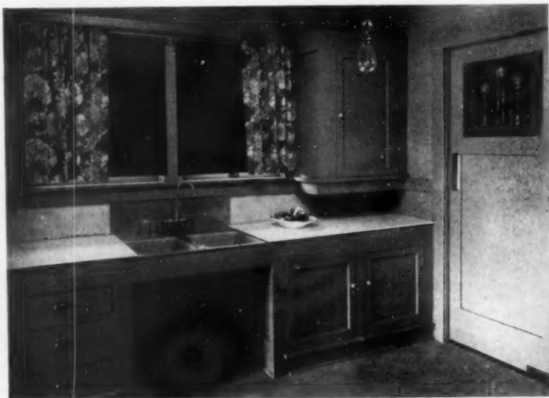
Concentrated efficiency—twin cobaltum sinks, sanitary vitrolite drainboard and work table, with flower bin and drawers below
