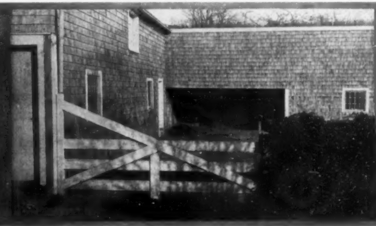
The post difficulty in this instance has been obviated, the strain resting solely on the hinges and diagonal bars
