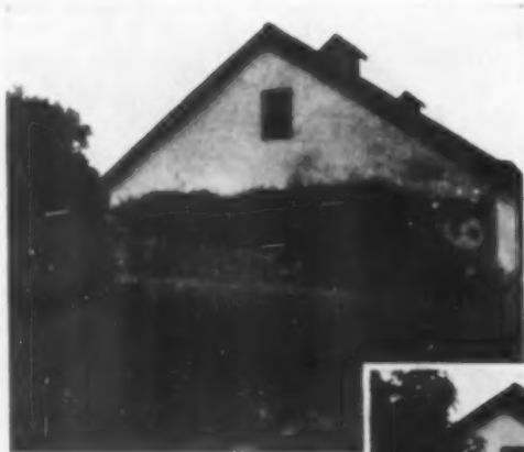
Much grading was necessary—ice-houses are well banked
