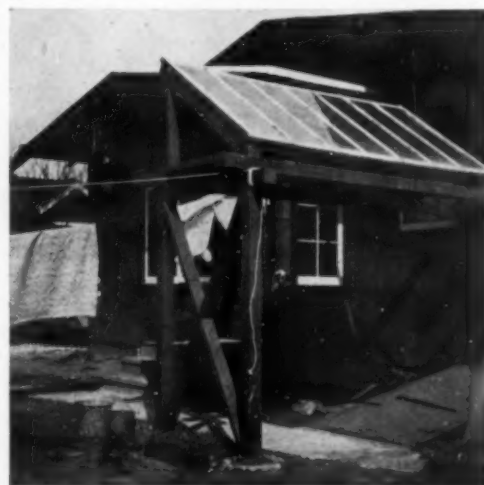
A solar water-heater mounted on the roof and supplying water at a temperature of 100 deg. F.
