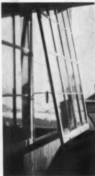
Sash hung according to the swinging cellar type
