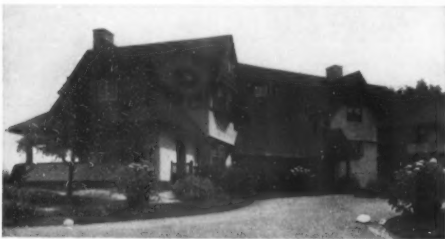
This stucco and timbered house is built on several radial axes, thus insuring a maximum of light and ventilation
