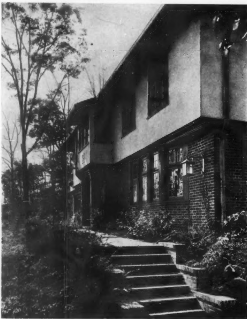
The treatment at one end of the house shows a particularly successful sun parlor and sleeping porch addition. The screened-in room on the first floor is paved in tile
