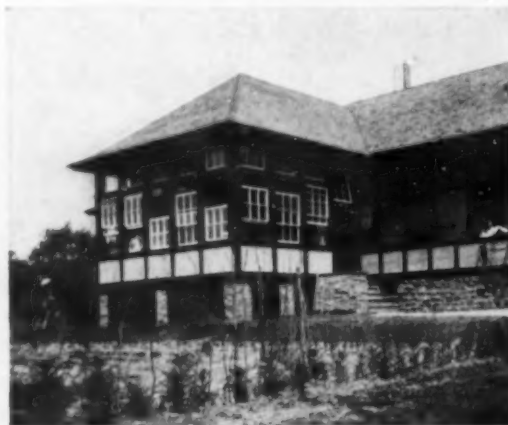
The entire wing of this cottage is devoted to outdoor sleeping. The enclosures are of the ordinary double-sash type, with transoms above
