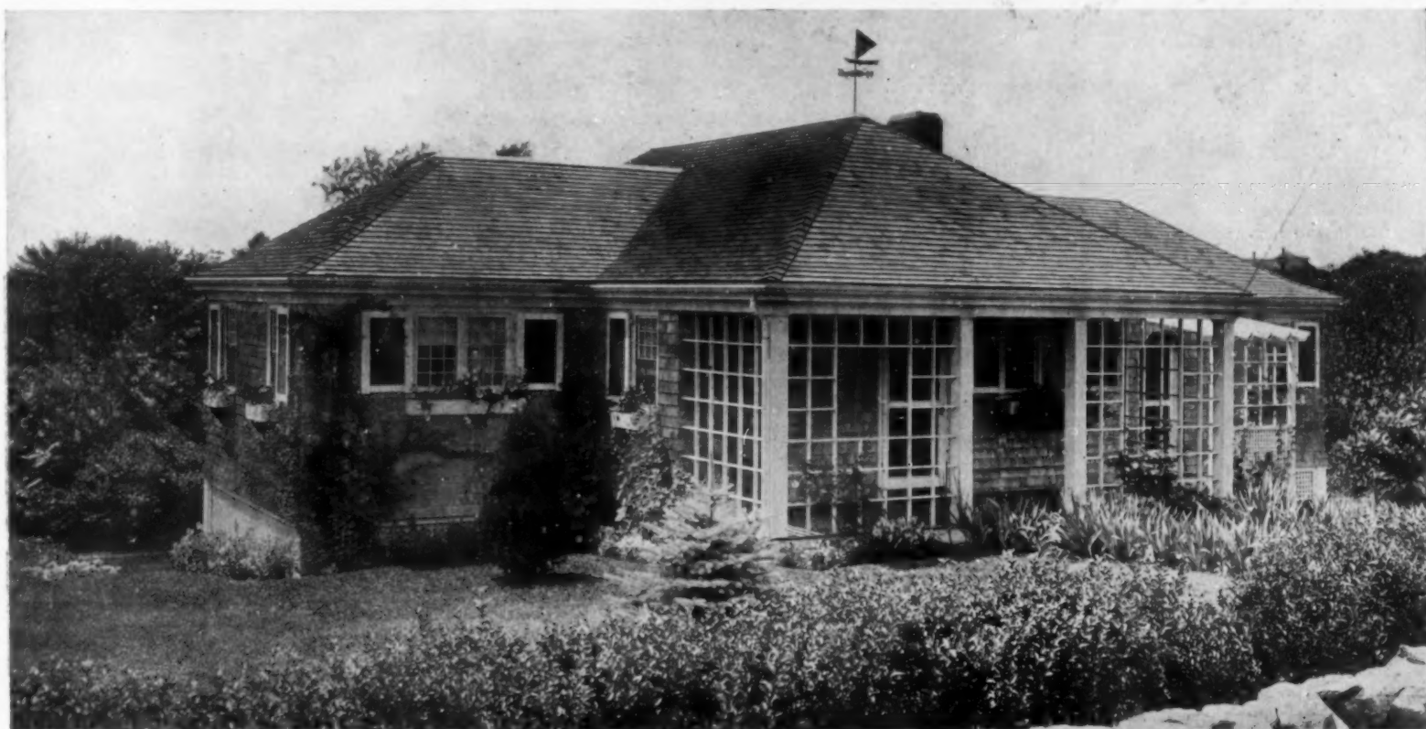
Cellar and foundation work is expensive. The summer house built on a steep slope may provide cool cellar space at little beyond the cost of excavation. A house of this plan provides opportunity for many windows and consequent cross draft
