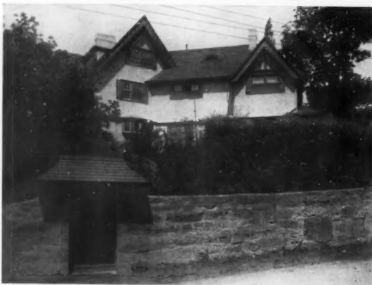
A good example of a wall of faced stones of irregular sizes and shapes, but well laid to harmonize with the style of building
