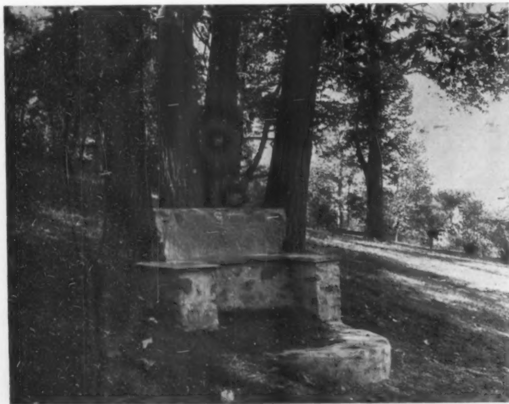
A little cement, some waste slate slabs and the litter of stone work makes "the wishing chair" that commands a magnificent view of the whole garden
