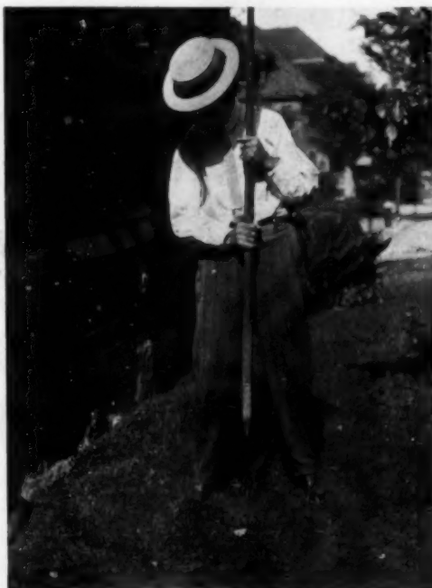
Ram the crowbar down hard and open each hole well
