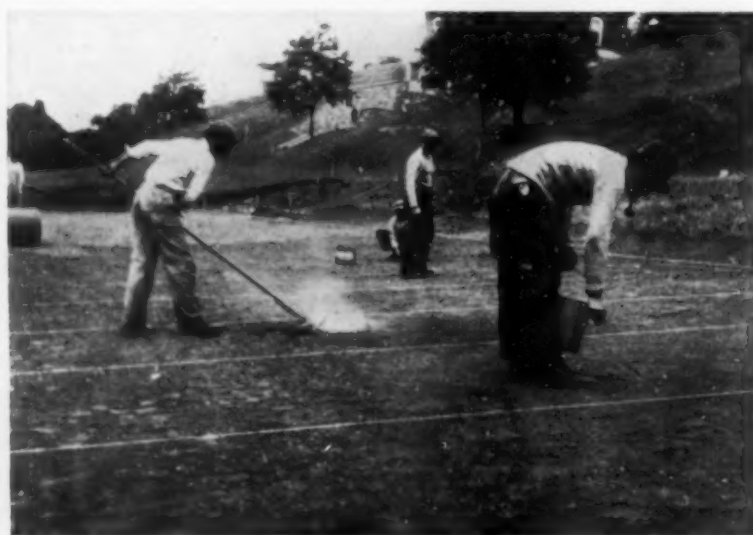
The lawn, thirty feet wide, was divided into six-foot strips, which were seeded separately, then raked and rolled at once
