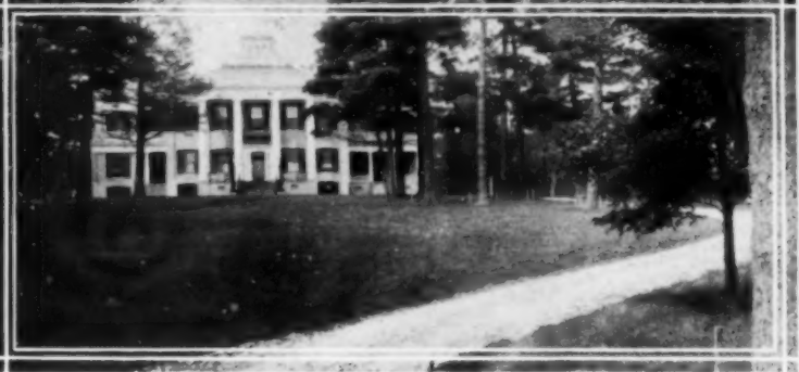
The Manor House at Walnut Hall Farm
