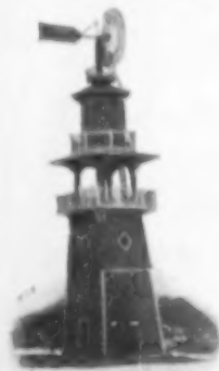
A Church Pneumatic Tank with Pumping Engine
