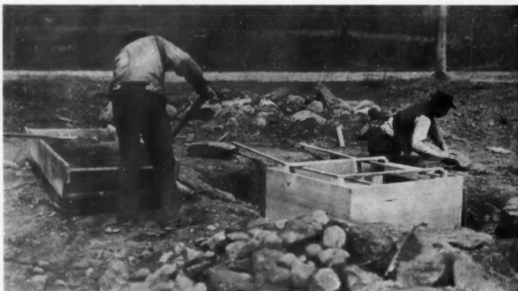
The construction is simple. A wooden "mold" is made, into which the cement is poured and allowed to harden
