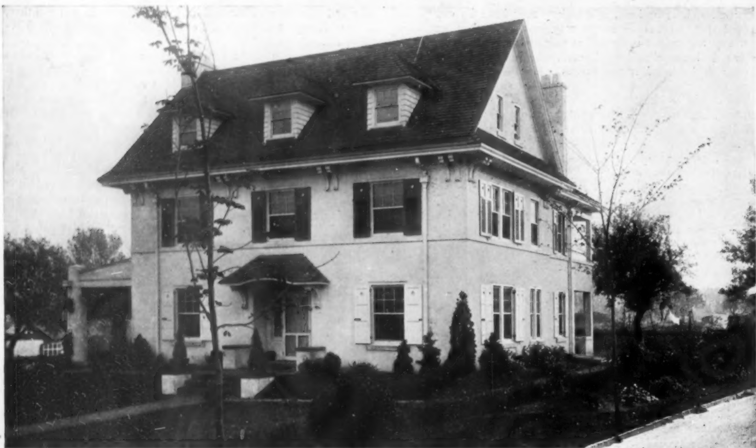
Mr. Shrigley's house is a good example of hollow tile construction, twelve-inch blocks being used on the first story and eight-inch above. To finish this, plaster and stucco are applied directly to the tile. In the floors of the entrance vestibule and the porches hollow tile and concrete were used and finished with cement
