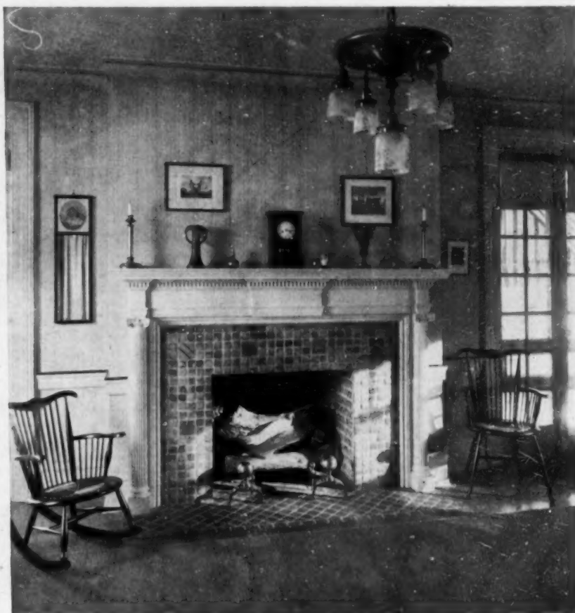
The living-room is sunny and is interesting in its simple fireplace and its plain paper. Tiles in the upper corners of the facing bear the family coat of arms, those in the back and jams are laid on edge to resist fire
