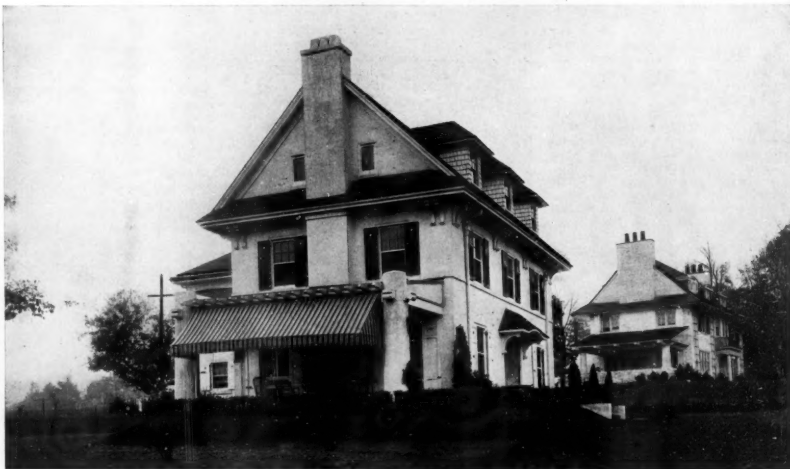
A deep green stain on the shingles is fitting with the stucco finish. The blinds are also green and the putty beads on all the window panes are painted black, which enhances the brilliancy of the glass. There is a rough stone fireplace on the porch
