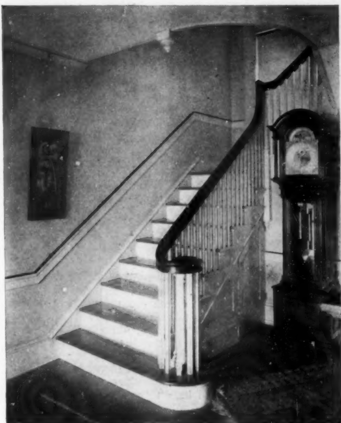
Beneath the landing a large closet with a window is placed and a small closet for overshoes is beneath the first flight. The stairway treatment of dark treads and white risers is effective
