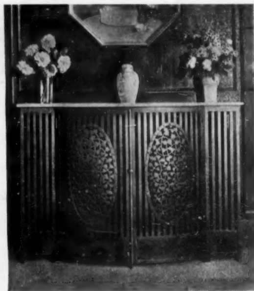
Above all, a radiator cover must provide easy access for regulating and cleaning the pipes
