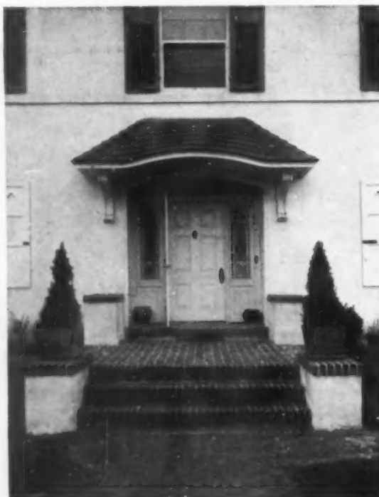
As the house faces north, the vestibule entrance was necessary. The door is set back about three feet and in winter a portable frame with door and sash may be put in on the outside wall line
