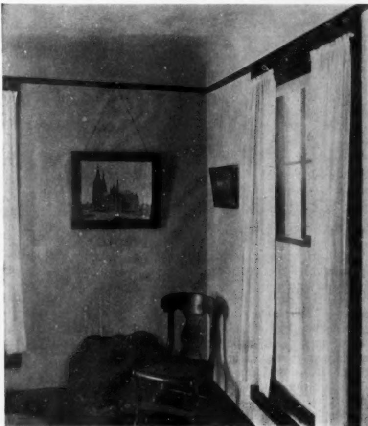
The sand finished walls of especially good construction are uncolored, retaining the grayish tint of the natural plaster
