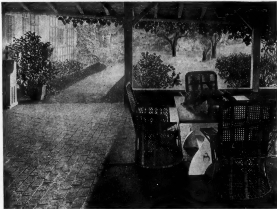
For a porch at ground level the floor should be of brick or other material that is unaffected by dampness. In such a situation wood rots too rapidly
