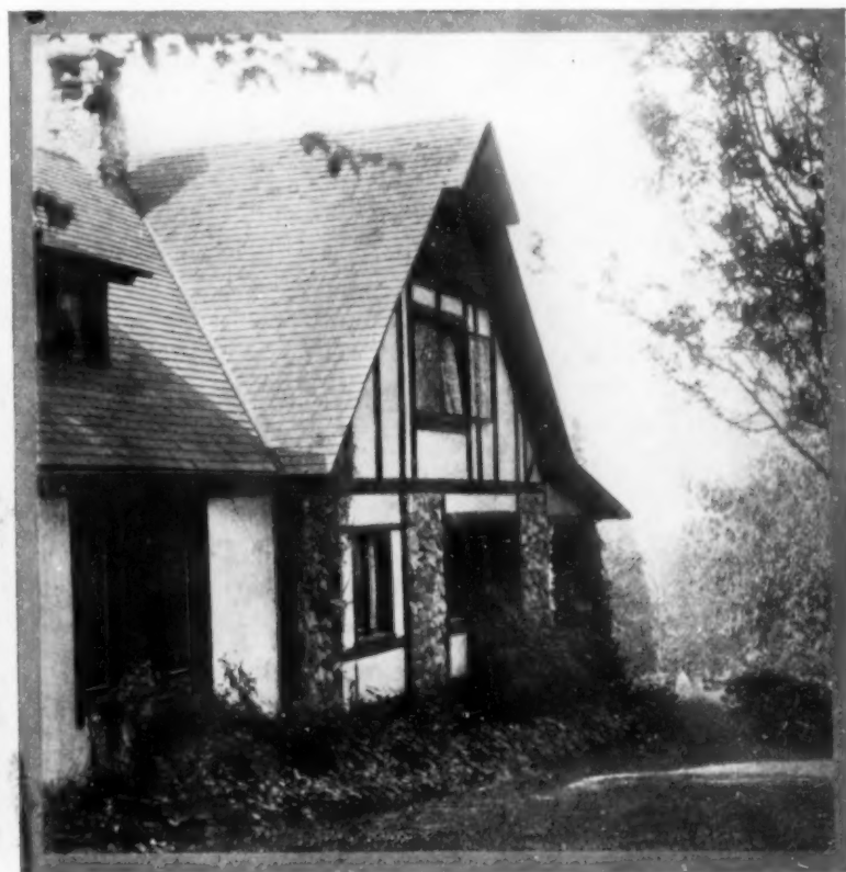
The half-timber work was of the sort used in the English houses; that is, was structural rather than purely decorative
