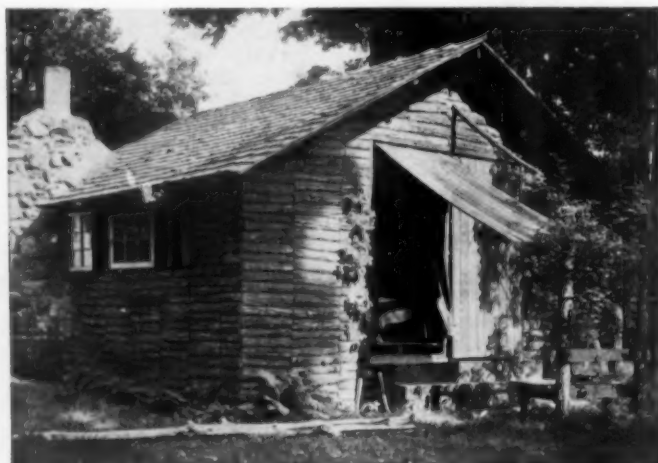
In this four hundred and fifty dollar bungalow sheathing boards overlaid with bark conceal the frame building
