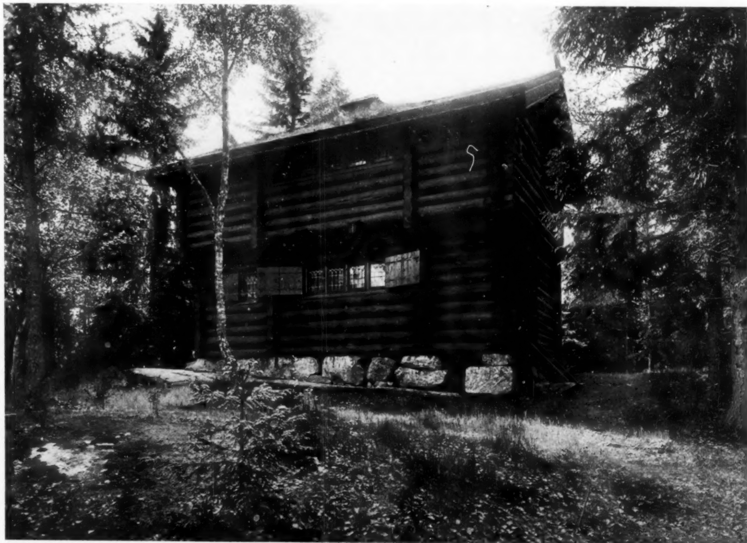
There is no excavated foundation to the log cabins of Sweden, but the house rests upon the ground and a foundation of heavy stones. The leaded windows with solid shutters are characteristic. Nearly all the partitioning is structural, as may be seen from the log ends projecting at either side of the row of windows
