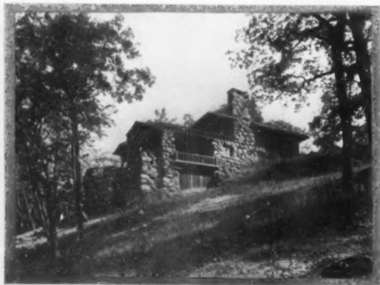
The local stone is built up to form a covered porch and terrace. The excavated slope saves in foundation cost
