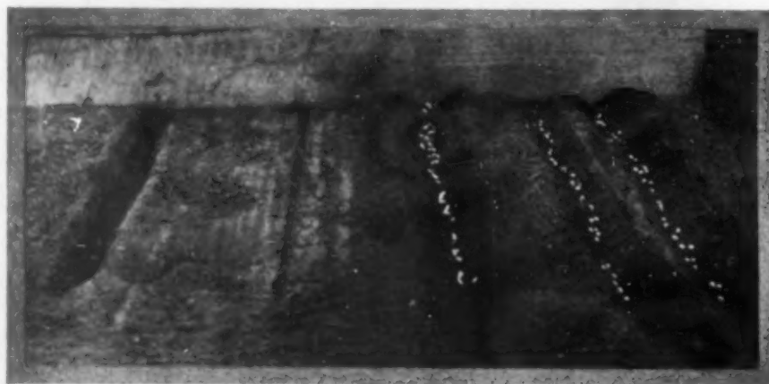
Drills for various seeds. From left to right: ¼" to ½" deep for lettuce; ½" to 1" for early beets; 2" for early beans; 2" double row for early peas
