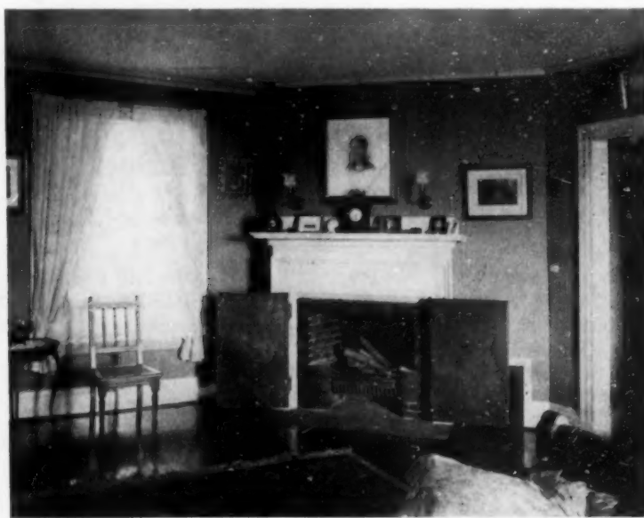
The annoyance of drafts from the fireplace may be remedied by hanging two doors such as shown in this illustration
