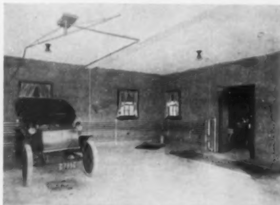
An interior showing overhead washer, heating pipes and wall lights near the floor
