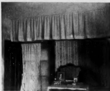
A ceiling closet is made by a redwood board above door and window
