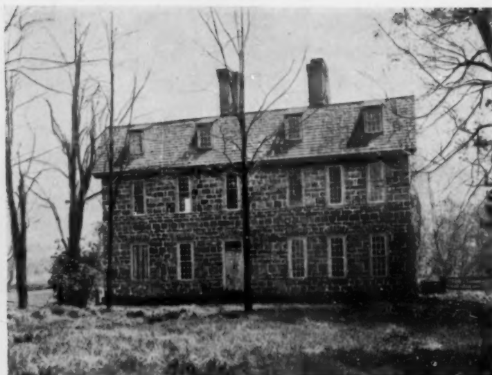
Between the two rows of narrow windows are courses of shaped stones that offer a pleasing variety in the design
