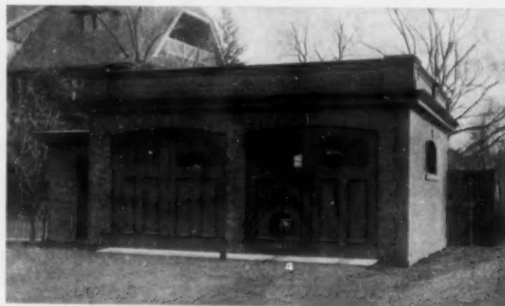
Another example of fireproof construction. Here the brick walls are plastered on the inside
