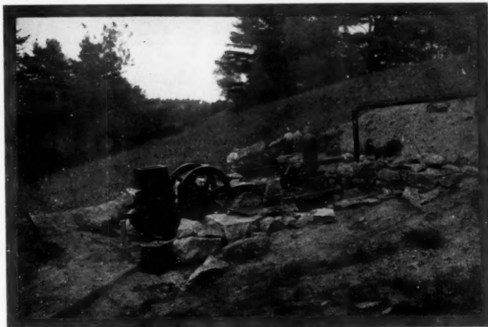
The pump and gasoline engine for forcing water into the spraying pipes were installed on the sloping ground near the pond
