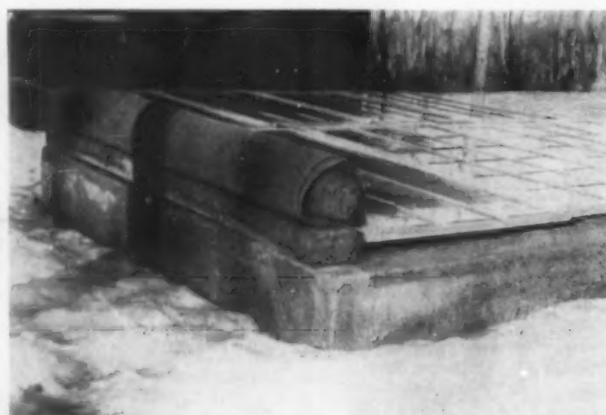
Concrete frames are the most desirable. This one shows a mat that is valuable for conserving warmth in zero weather
