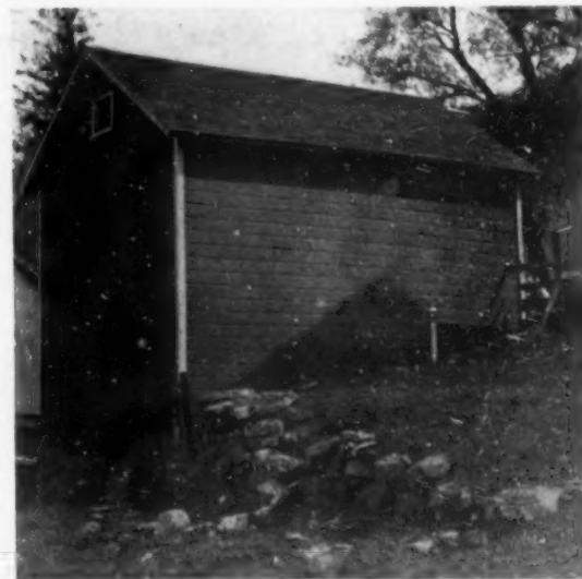
If set in a hillside the ice house may be filled from the upper side with less labor
