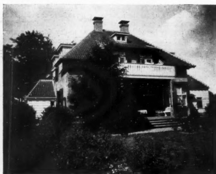
Instead of being a mere shed, this piazza roof is inclosed with a railing and fitted up as a useful porch
