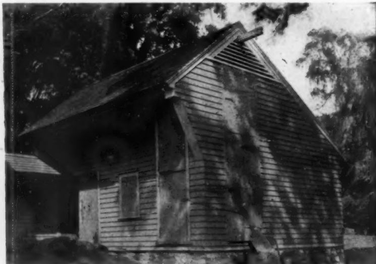
Some sort of ventilation, such as fixed slats or open spaces under the eaves, must be provided to carry off the moist air
