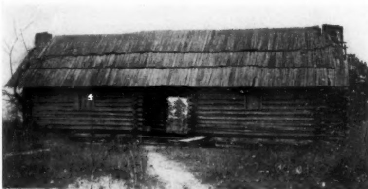
An idea for a camp was taken from the negro cabin roofed with shakes. The ends are living quarters, the open space between, the dining-room
