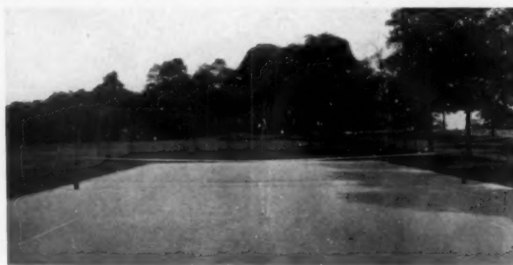
The level dirt court is the most common and more durable type and may be kept in condition by constant rolling
