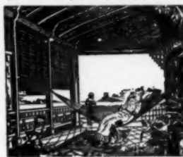
Wilson's Porch and Piazza Blinds
