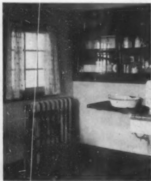
The improved vapor systems bring the steam in at the top of the radiator. It flows steadily and obviates all "knocking in the pipes"
