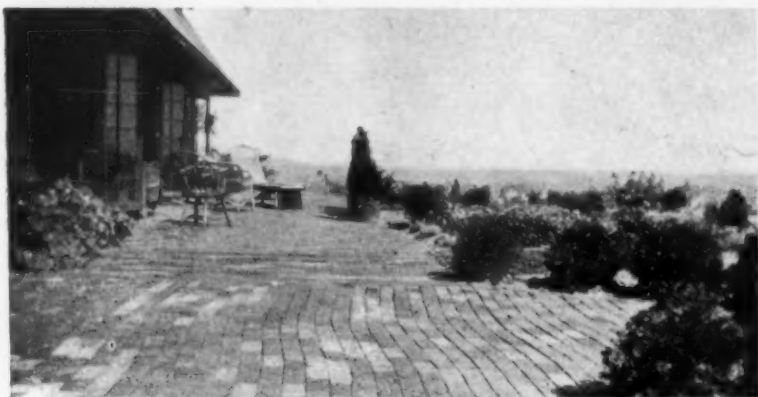
The crest of the hill was extended out and upon this a terrace of fired brick, showing a fine color effect, was built
