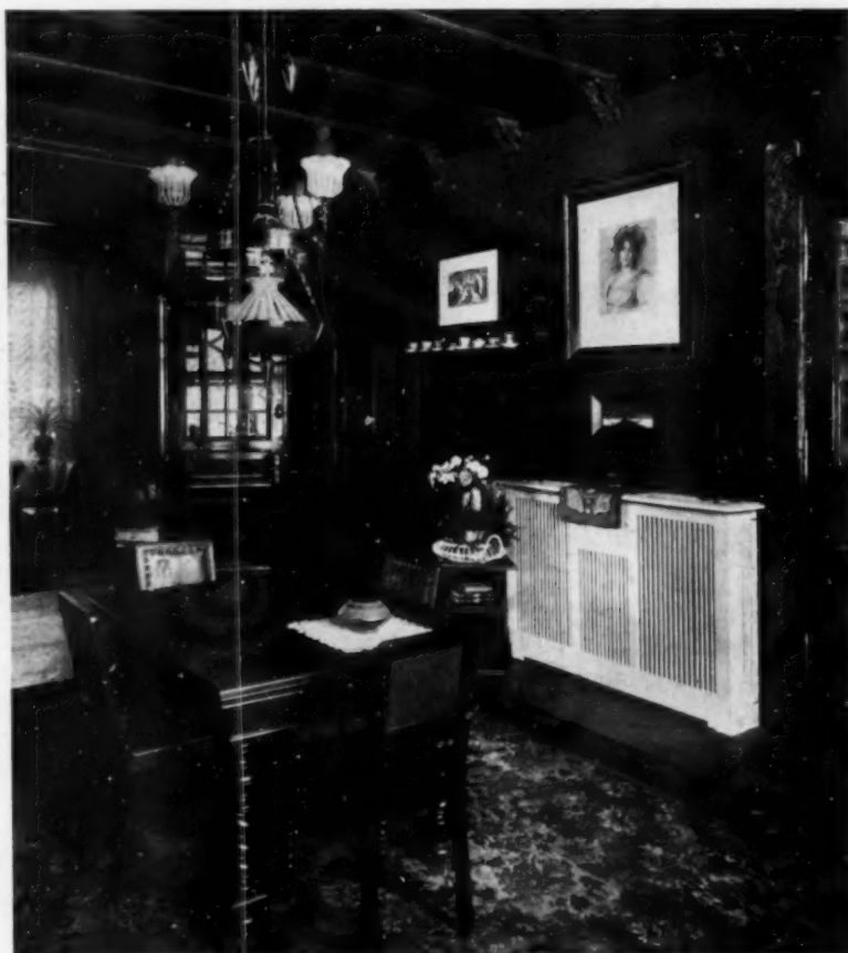
The German architect makes his heating apparatus a decorative feature by using unfinished radiators and covering them with a removable screen
