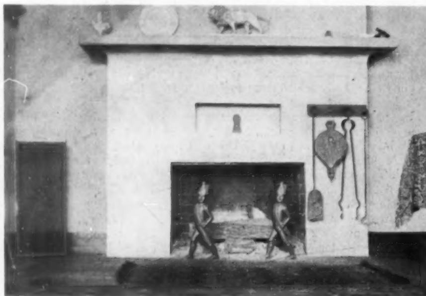
With the new throat and smoke chamber the fire burns perfectly and the new finish of the mantel was found more satisfactory than the former one
