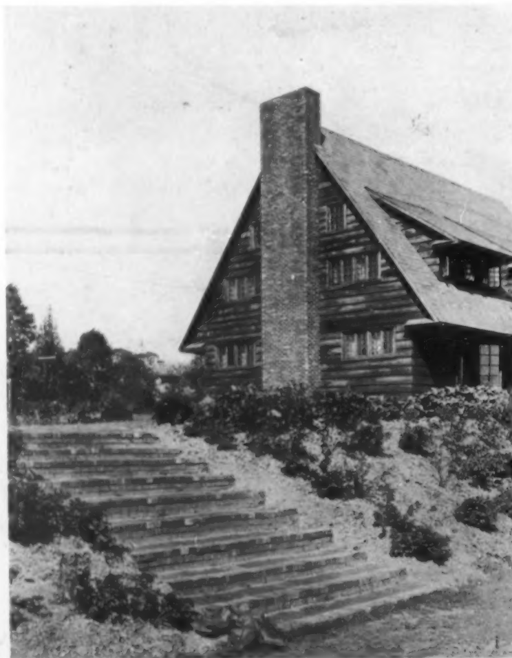
Another view of the terrace front of the cottage, with the brick steps, which lead from the pergola to a lawn and tennis court several feet below. These steps are another example of the artistic value of bricks irregularly laid and of different color
