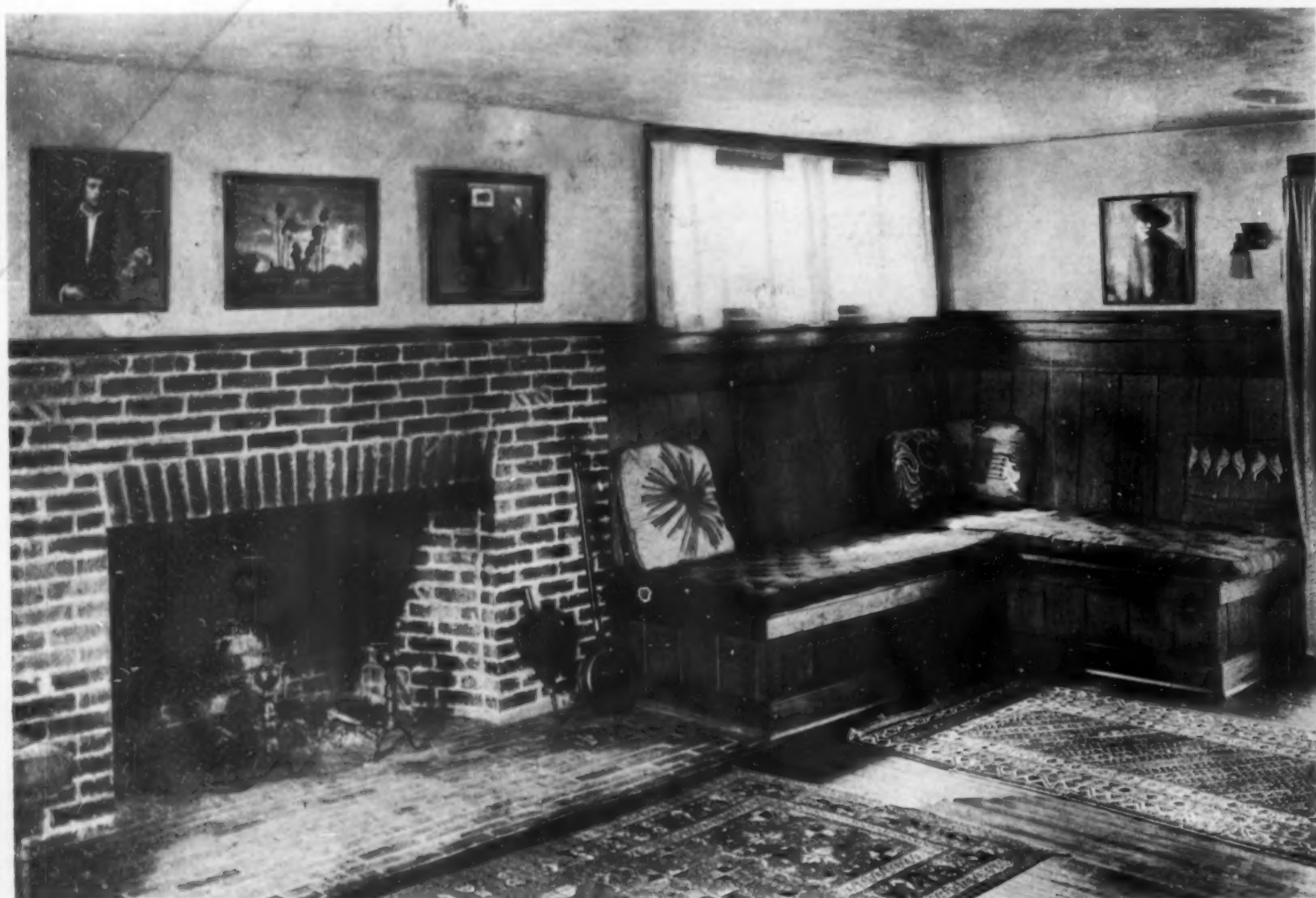
The living-room fireplace, flanked by spacious built-in-seats, is constructed of the exterior brick, varying in tone from a bright red to a dark, bluish gray, put together with ordinary gray mortar
