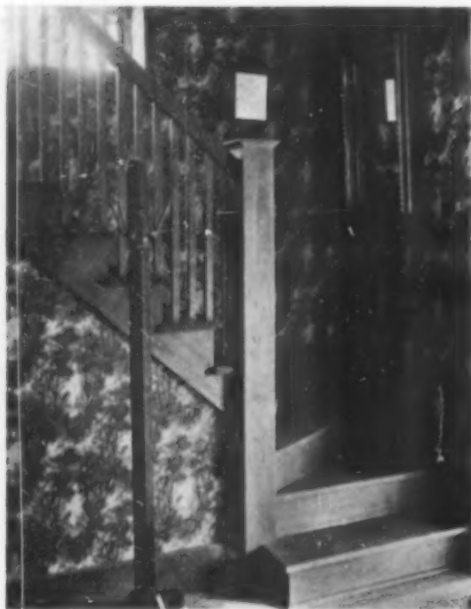
A remarkably effective and inexpensive treatment of cypress. The wood is cheaply milled, stained brown and wax finished
