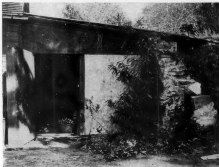
A cellar built into a hillside. Its walls are air spaced and by keeping things dry, cool and well ventilated decay is prevented
